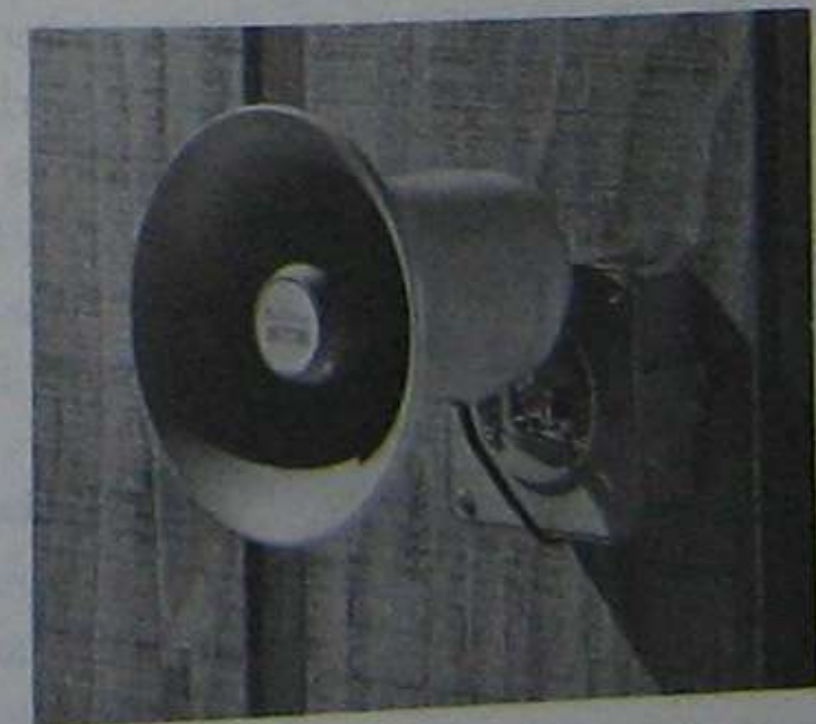
FIGURE 5-21. A horn is often used to alert neighbors that an intruder is on the premises.
