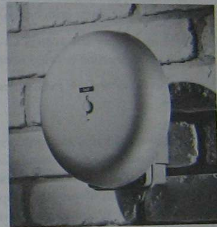
FIGURE 5-20. A bell may be used as a means of sounding the alarm.
