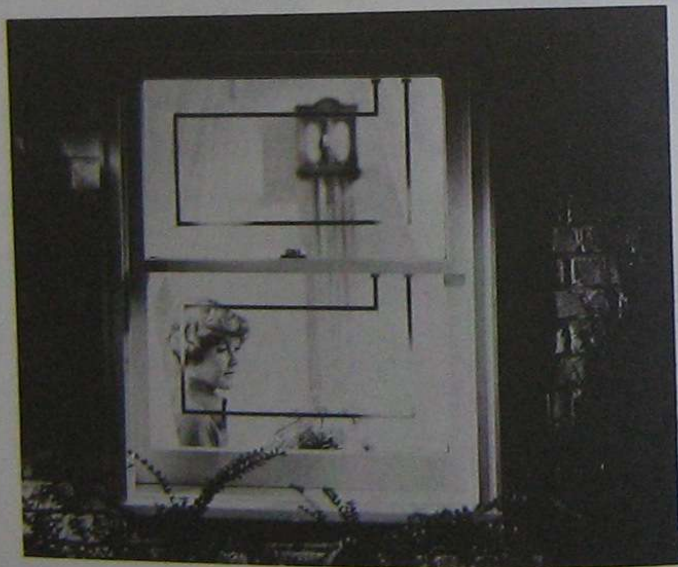
FIGURE 5-15. Window foil should be used on all windows as well as on sliding glass doors.
