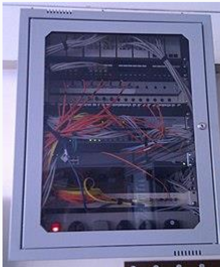
A wall-mount cabinet containing optical fiber interconnects. The yellow cables are single mode fibers ; the orange and aqua cables are multi-mode fibers : 50/125 \mu\text{m} OM2 and 50/125 \mu\text{m} OM3 fibers respectively.
