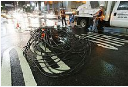
Fiber crew installing a 432-count fiber cable underneath the streets of Midtown Manhattan, New York City
