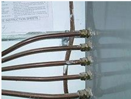
PVC-sheathed MICC cable. Conductor cross section area is 1.5 mm² ; overall diameter is 7.2 mm
