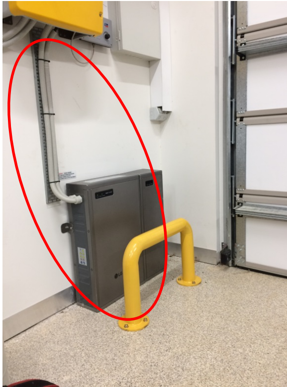
Figure 1 Scope of these guidelines: The battery system including cabling up to PCE terminals
