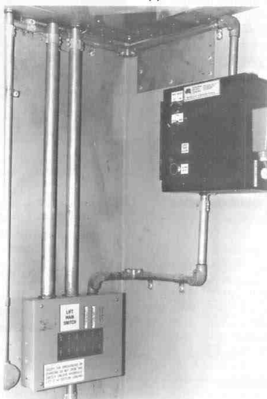
Fig. 19.13 Electrohydraulic lift installation: (a) control panel using PLCs for multifunctional control of the lift; (b) flexible travelling cables emerging from steel trunking in the lift shaft; (c) distribution board installed in accordance with Clause 2.19.4.1
