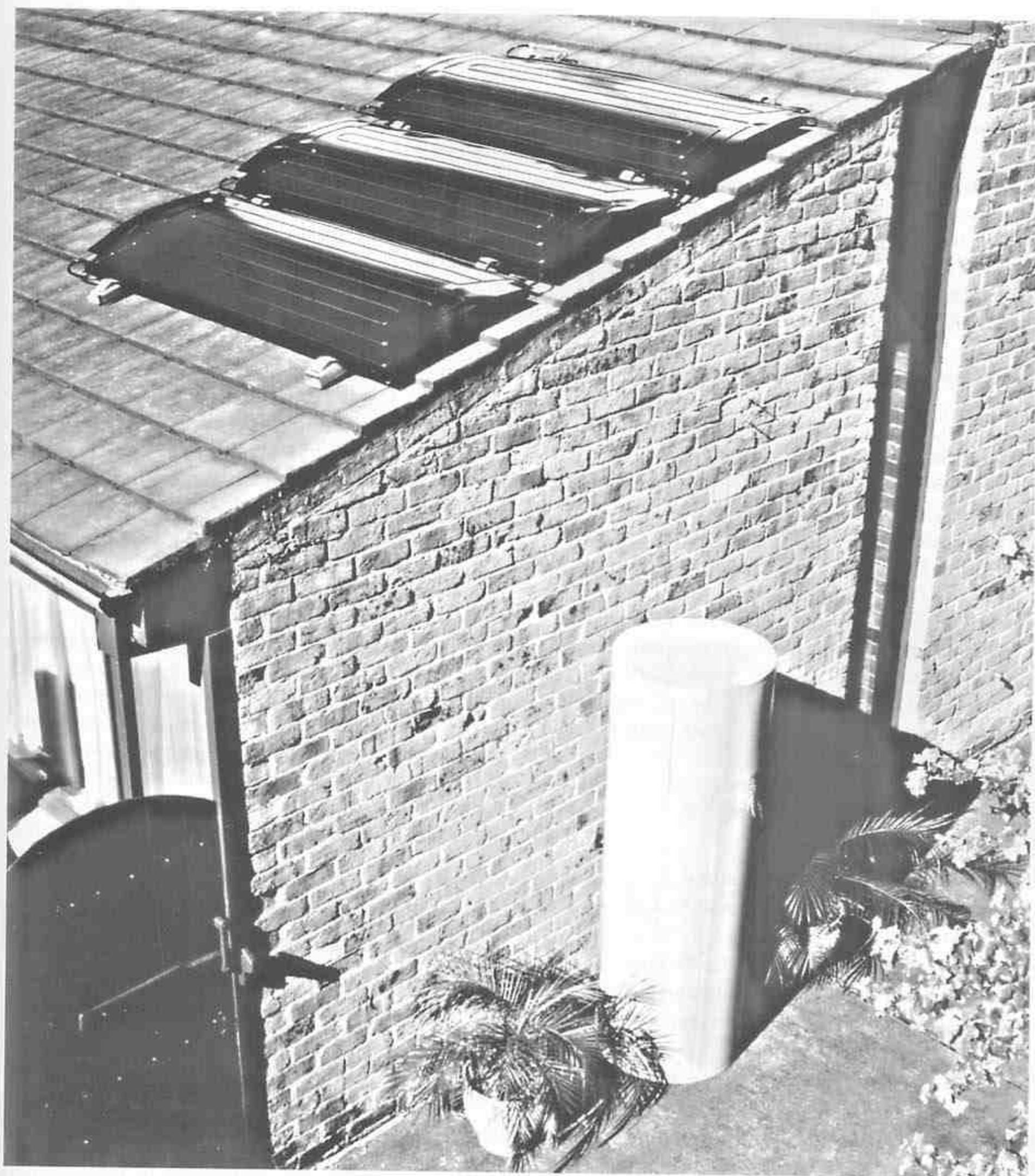
Fig. 21.15(b) Quantum split system SES WATER HEATERS
