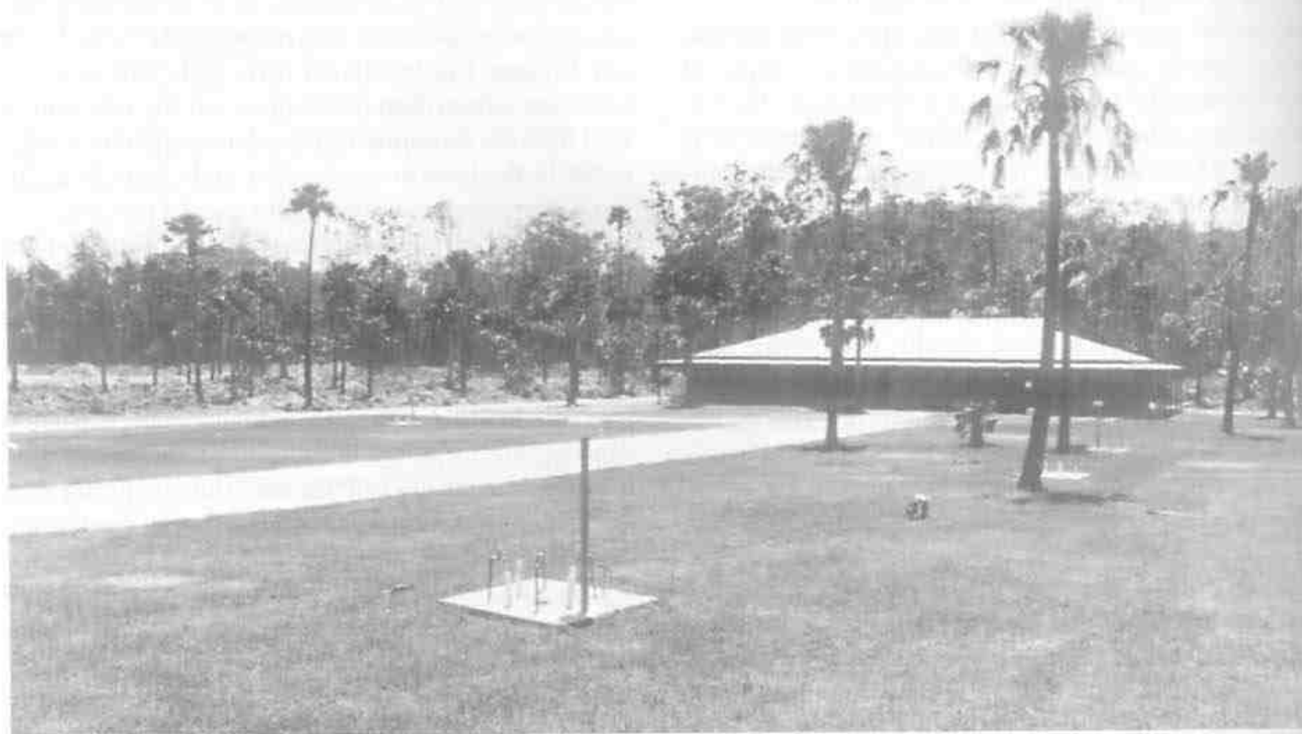
Fig. 19.9 Recreational camping ground showing distribution posts for supplying camp sites. Note the long distances from the distribution board at the left end of the amenities building to each distribution post
