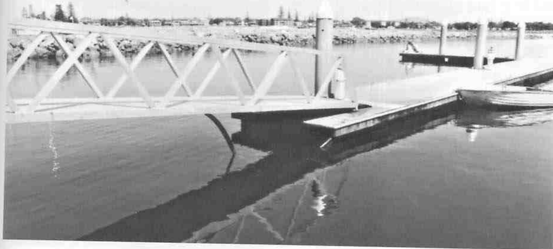
Fig. 19.8 The wiring system installed on this public marina is circular TPS cable. Note the additional section of cable, enclosed in black PVC flexible conduit, from the ramp to the pontoon section to allow for tidal movement
