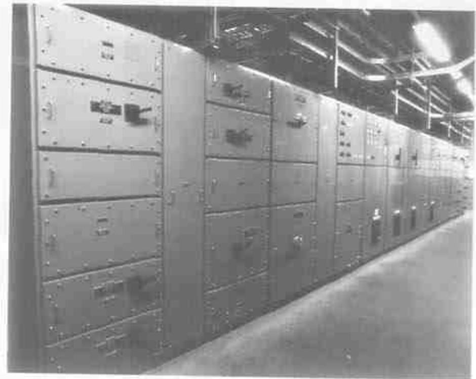
Fig. 17.15 Custom-built 5000 A switchboard: built to customer's as well as relevant energy distributor's specifications K.E. BROWN ELECTRICAL SWITCHBOARDS
