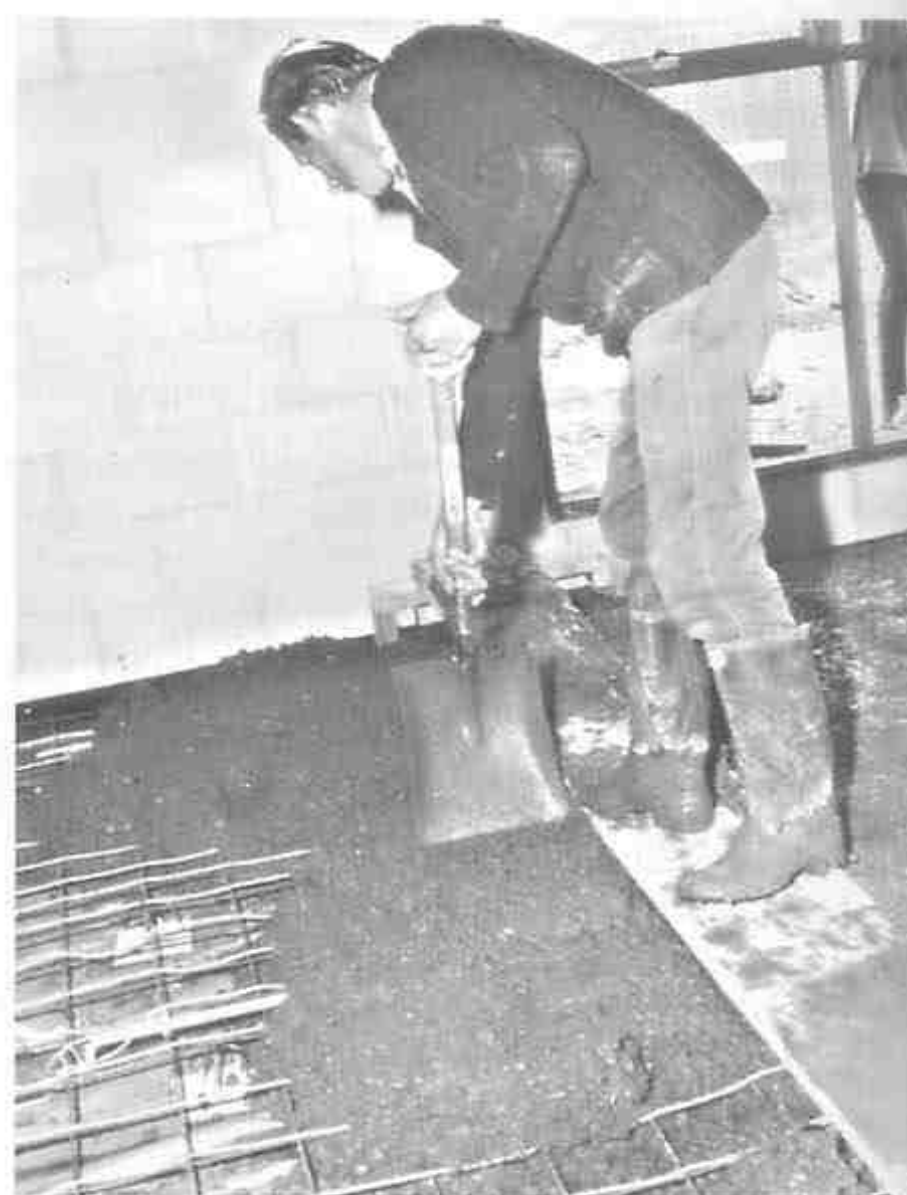
Fig. 21.20(b) Cables embedded in the actual concrete slab. They are continually tested while concrete is being poured
