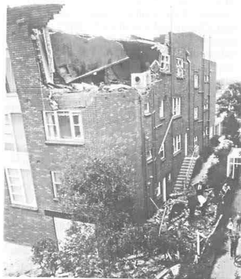
Fig. 21.1 Damage to buildings caused by the explosion of an unvented storage water heater SYDNEY ELECTRICITY
