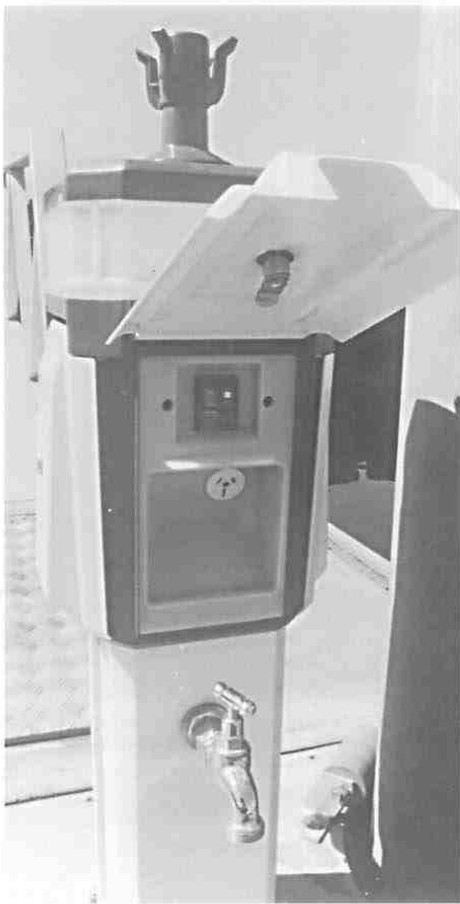
Fig. 19.11(b) Outlet protected by a combined RCD/MCB for connecting shore supply to a moored boat
