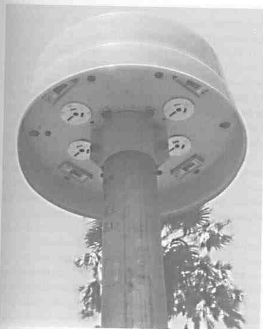
Fig. 19.10(b) The outlets and their circuit breakers are protected from the weather and against mechanical damage by being mounted on the underside of the overhanging cover. This equipment was installed before RCD protection became a requirement in some states
