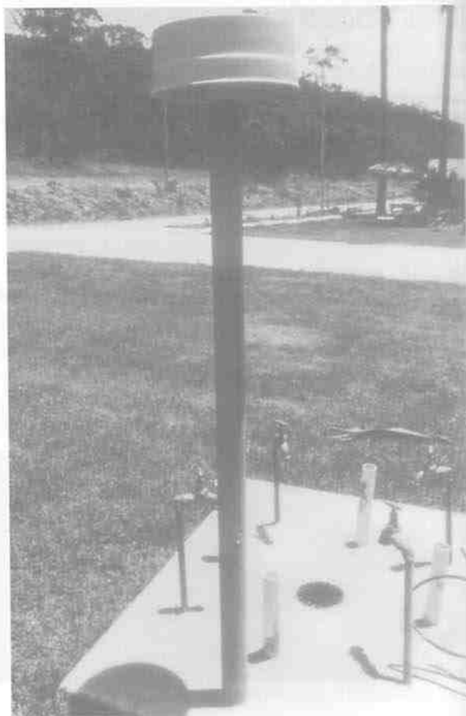
Fig. 19.10(a) Distribution post for servicing four camp sites
