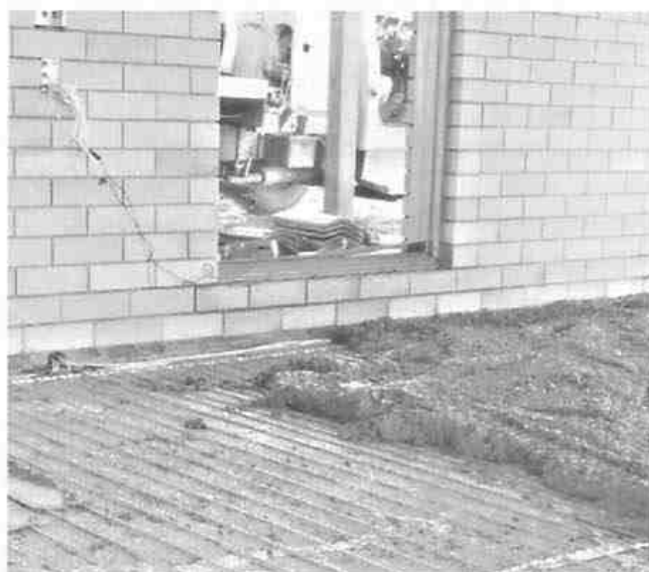
Fig. 21.19 Concrete screed nearing completion covering heating cables that have been fixed to an anchoring strip ELECTRIC HEATING SERVICE
