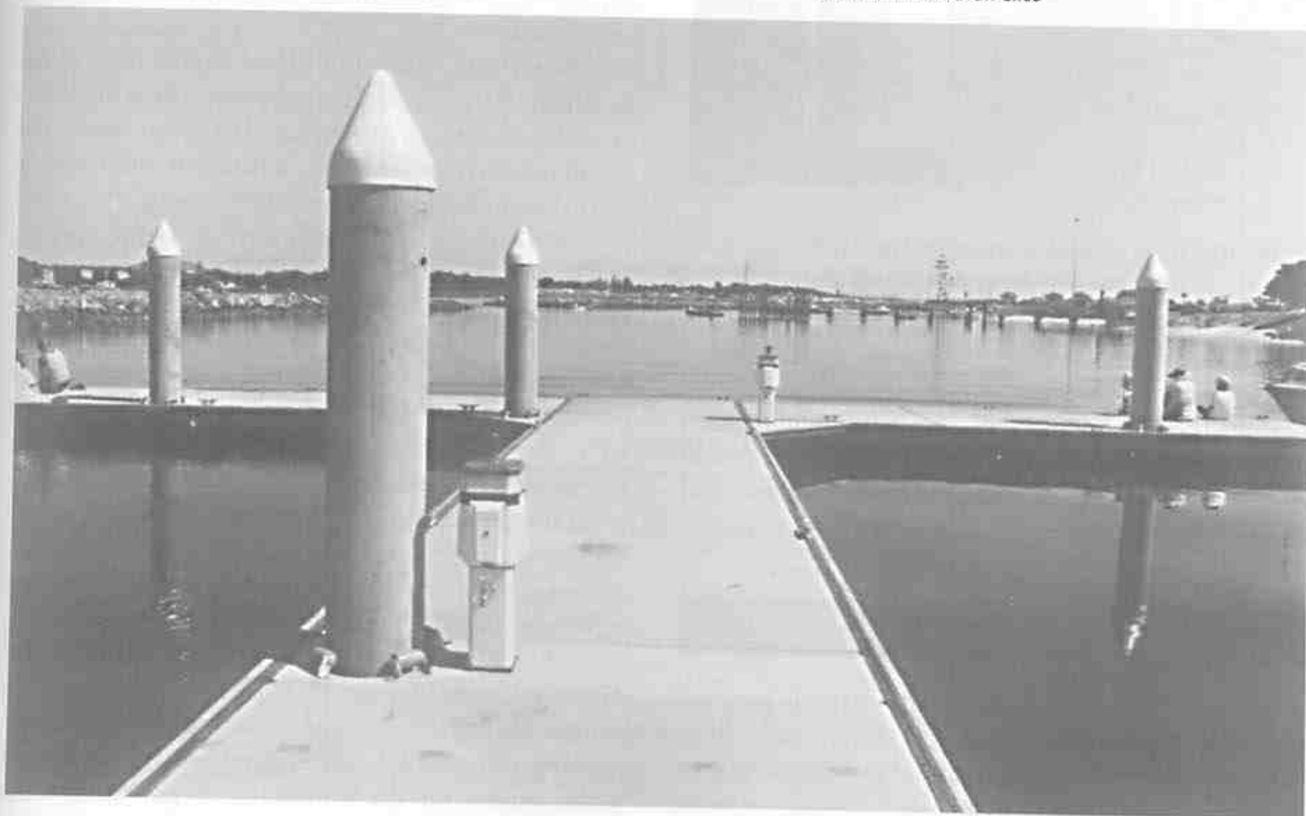
Fig. 19.11(a) Modern marina with distribution centres for the supply of electricity and fresh water to moored pleasure craft
