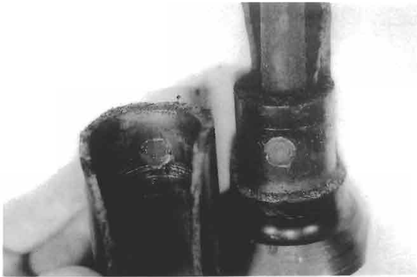
Fig. 2. Typical fracture through the centre of the weld and along the piston rod. The location of one of the rosette welds can be seen.
