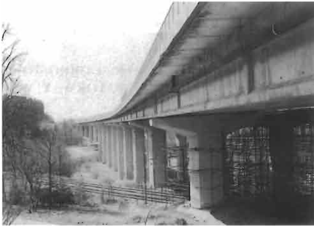
Fig. 1. Prestressed concrete construction of the viaduct.
