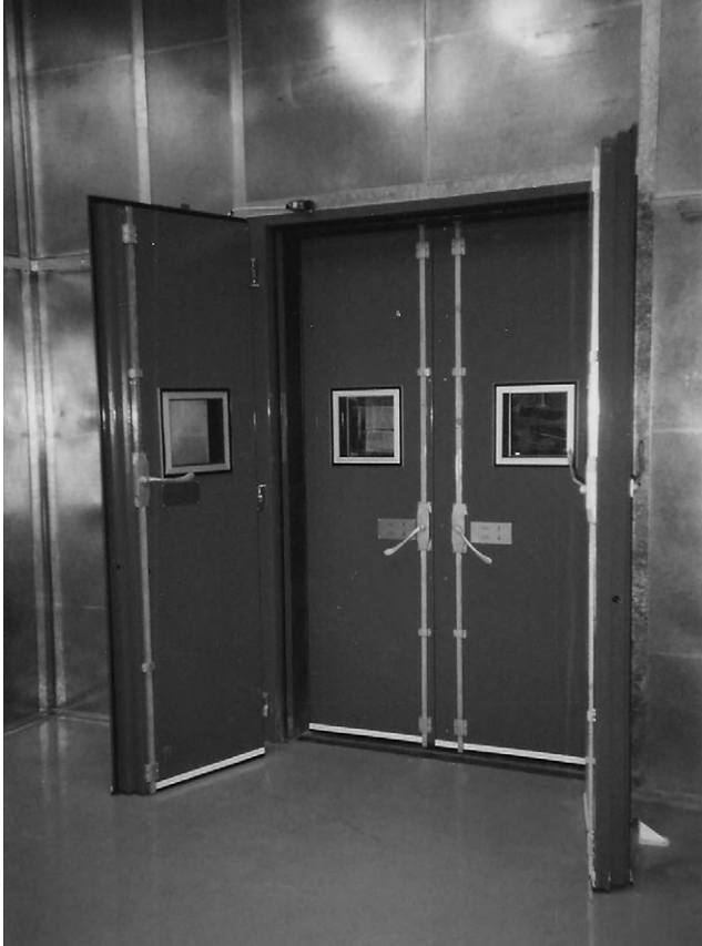
FIGURE 4.6 Double pairs of cell doors built into a high-noise, acoustic-panel-constructed engine test cell. (Photo courtesy of Enviosound Ltd.)
