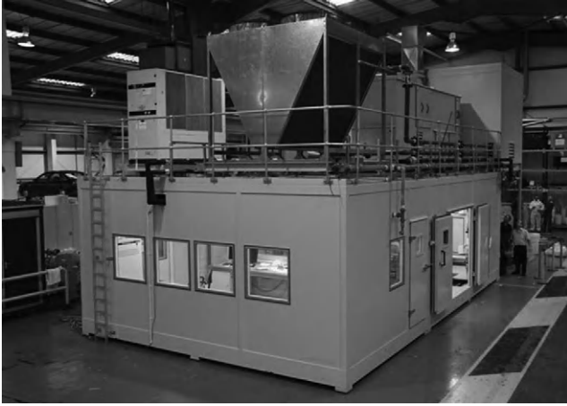
FIGURE 4.1 A “building within a building” test cell and control room, constructed on existing factory floor using acoustic panels within a steel frame. Note the raised door sill. All the services, including air blast cooler, are roof mounted. (Photo courtesy of Envirosound Ltd. )
