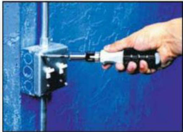
Metal electrical boxes should be grounded to prevent shocks.
