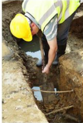
If you touch a live electrical component with an uninsulated hand tool you are more likely to receive a shock when standing in water.
