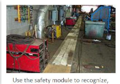
Use the safety module to recognize, evaluate, and control workplace hazards like those in this photo.
