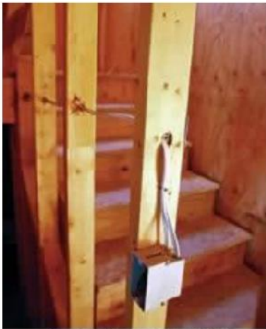
Nonmetallic sheathing helps protect wires from damage.
