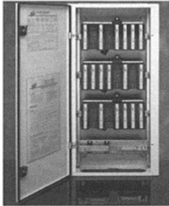
Figure 6.6 Distribution board (Courtesy of Eaton Electric Ltd)
