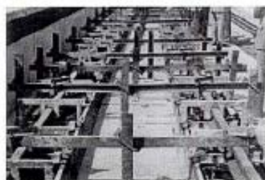
Fig. 6: Supported rail, formwork for the longitudinal plinths.
