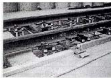
Fig. 13: Details view: Temporary support for the positioning of the rails.
