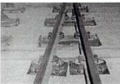
Fig. 12: Delkor Egg® in the entry area of a switch, without safety rails.
