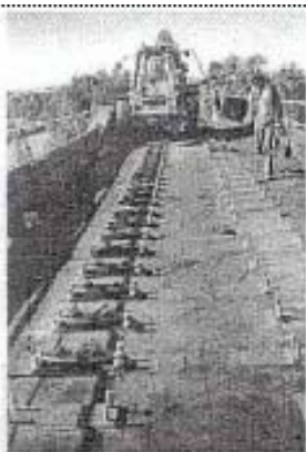
Fig. 7: Mounting of Delkor Egg® type rail fasteners on steel bridge, screw fitting on welded plates.
