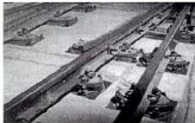
Fig. 11: Delkor Egg® in the entry area of a switch, with safety rails.
