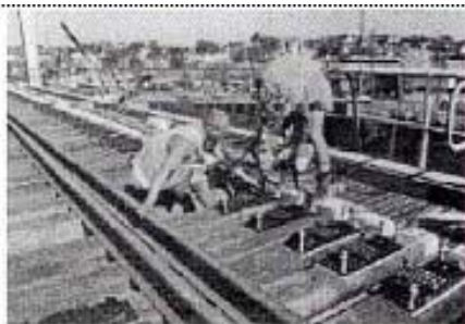
Fig. 8: Screw-fitting of rail fasteners on timber sleepers.
