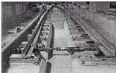
Fig. 10: Delkor Egg® employed in a switch blade/sliding bolster area.
