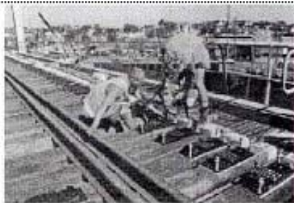
Fig. 8: Screw-fitting of rail fasteners on timber sleepers.
