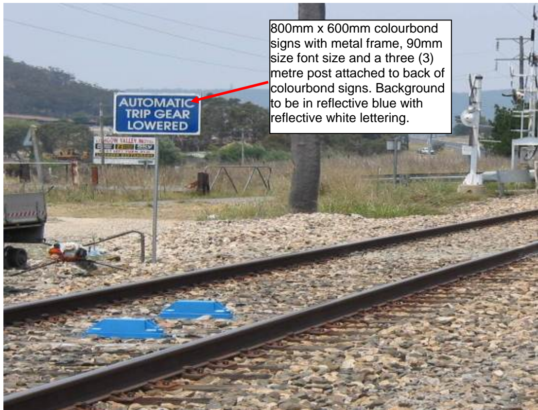
Figure 26: Identifies signage used when Automatic trip gear is lowered
