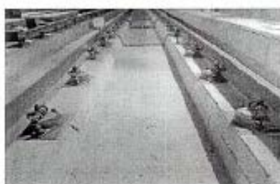
Fig. 5: Delkar Egg® mounted on concrete longitudinal plinths.
