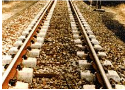
(b) Twin-block concrete sleeper
