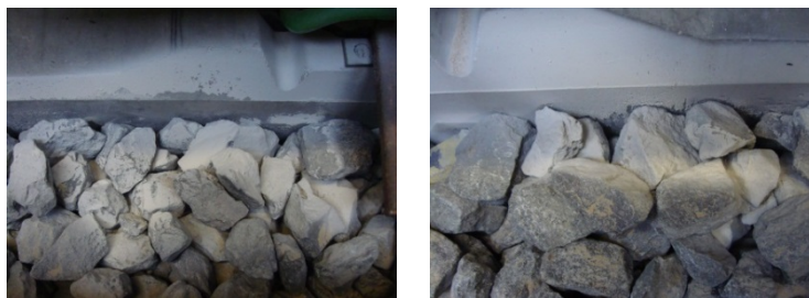
Figure 7.77: Flour-like fines arising from sand crushing brought to the ballast and sleeper surface because of cyclic movement of the sleeper
