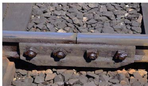
Figure 2.11: Fishplate connection system (De Bold, 2011)
