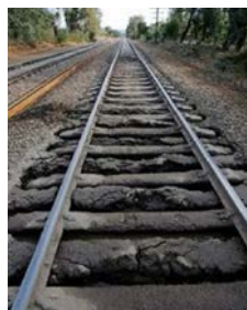
Figure 2.6: Fouled railway track (Kaewunruen, 2011)
