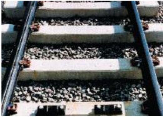
(a) Mono-block concrete sleeper
