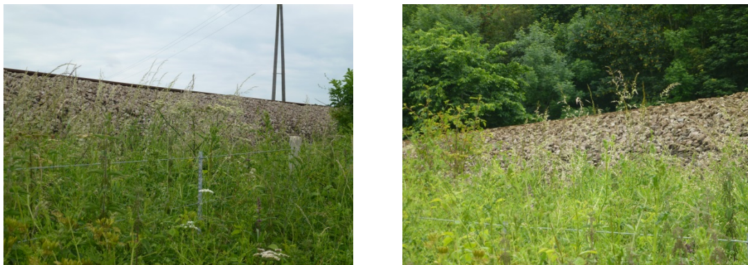
Figure 6.55: High ballast shoulders at Haltwhistle on the railway line between Carlisle and Newcastle upon Tyne (courtesy of Prof. William Powrie)
