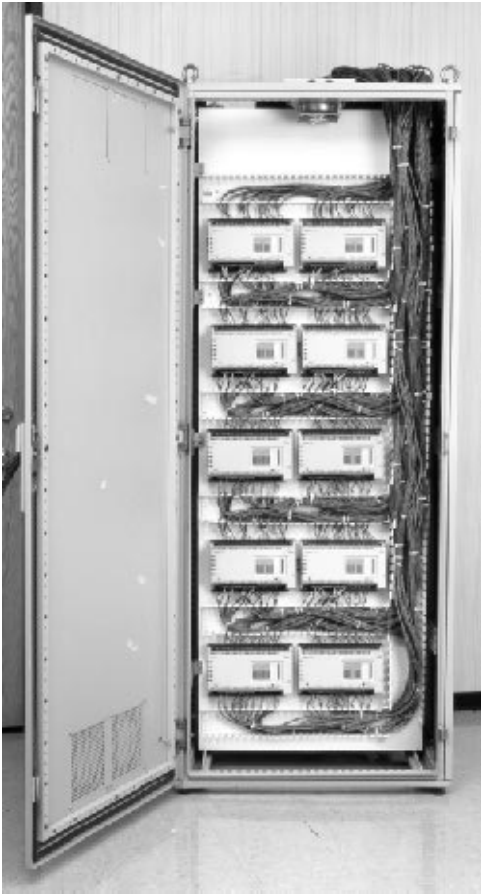
FIGURE 3 Footprint is significantly reduced when FOUNDATION fieldbus is used. The full cabinet handles 320 inputs and outputs (I/O).
