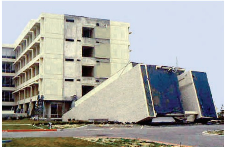
Figure 8-2: Olive View Hospital. A brand new facility that was damaged beyond repair in the 1971 San Fernando earthquake due to a shaking intensity that exceeded what was expected at the site and a design that, although technically complying with code at the time, contained several structural characteristics now considered major deficiencies. The lateral system contained nonductile concrete frames, discontinuous shear walls, and a significant weak story.
