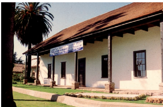
Figure 8-26: The museum at San Gabriel Mission, southern California, a historic adobe structure damaged by earthquakes in 1987 and 1994. It was repaired and strengthened, including installation of a bond beam of steel in the attic, anchor bolts into the wall, and stitching of cracks back together on the interior walls.
