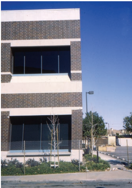
Figure 8-3: An example of a recently designed building with seismic deficiencies not understood at the time of design. In this case, the deficiency was “pre-Northridge” moment-frame connections, which proved to be extremely brittle and unsatisfactory. Hundreds, if not thousands, of these buildings were designed and built in the two decades before the Northridge earthquake (1994).
