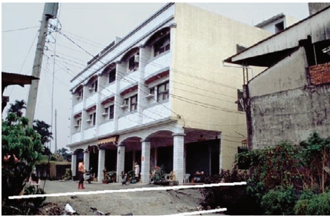
Figure 2-5: This building near Juahan, in Taiwan, was lifted several feet by the fault. Fault rupture runs just near the side of the building, down the alley. The white lines highlight the offset ground surface. There was no apparent damage to the building.
