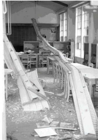
Figure 9-5: Falling objects can be a direct threat to life, as can be envisioned in this example, had children been sitting in the seats in this elementary school library in Coalinga in 1983.
