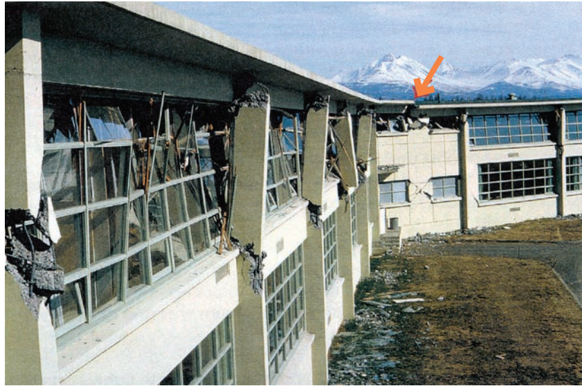
Figure 5-22: West Anchorage High School, Alaska earthquake, 1964. Stress concentration at the notch of this shallow L-shaped building damaged the concrete roof diaphragm.
