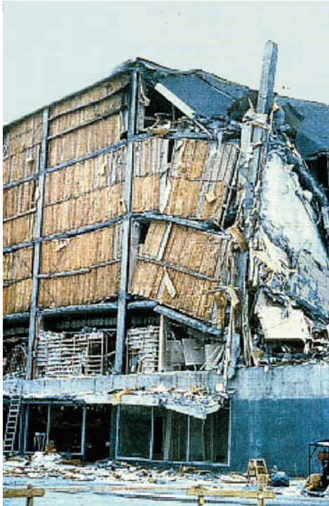
Figure 5-18: Penney's store, Anchorage, Alaska, earthquake, 1964. Left: Damage to the store: loss of perimeter precast panels caused two deaths. Right: Second-floor plan, showing unbalanced perimeter resistance. SOURCE: JAMES L. STRATTA
