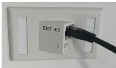
Figure 7 (a) Single RJ45 network socket.
