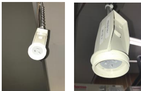
Figure 5 Suspended Pendent type - Industrial captive screw sockets –
