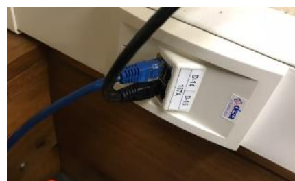
(b) Dual RJ45 network socket.
