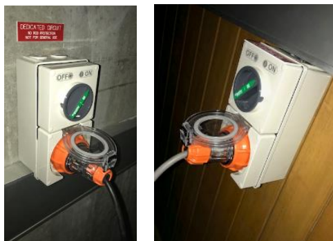
Figure 3 Industrial captive screw sockets – wall mounted- Clipsal type 56 series.
