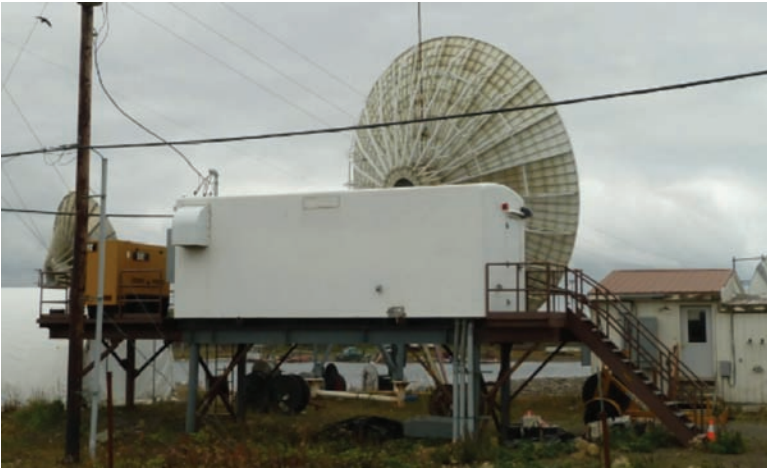
Figure 4.5. C-band satellite earth station constructed in Nome, Alaska.
