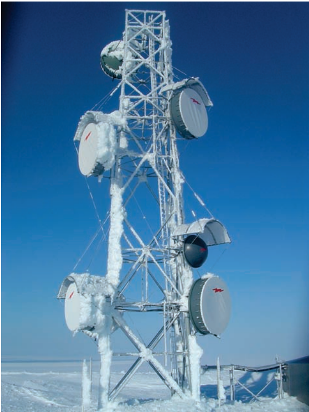
Figure 3.6. Microwave tower damaged by ice formation.
