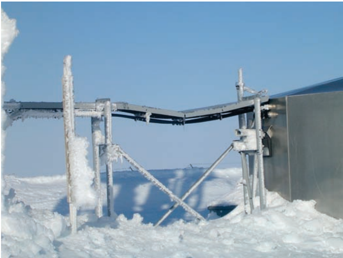
Figure 3.7. Ice bridge infrastructure damaged by ice formation.
