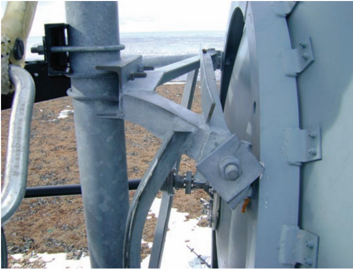
Figure 3.8. Long-haul microwave antenna mount damaged by ice formation.
