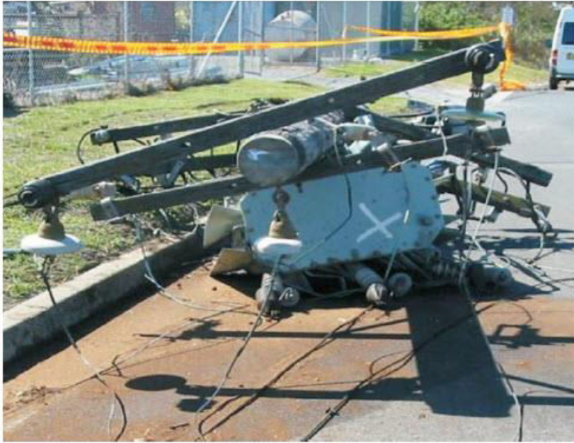
Fallen power pole with transformer leaking oil
