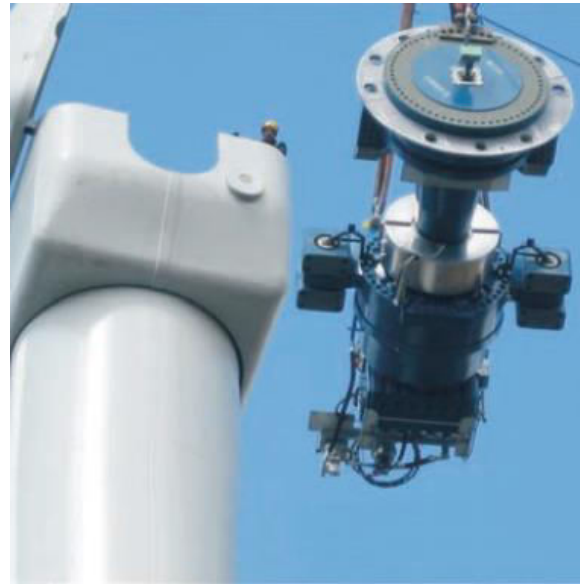
(b) wind generator under construction
