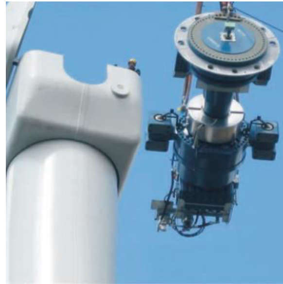
(b) wind generator under construction
