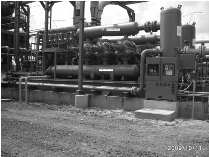
Figure 11-1. Separable Balanced Opposed 6—Throw Engine Driven Compressor in Pipeline Service Complete with Off-skid Mounted Control System.
