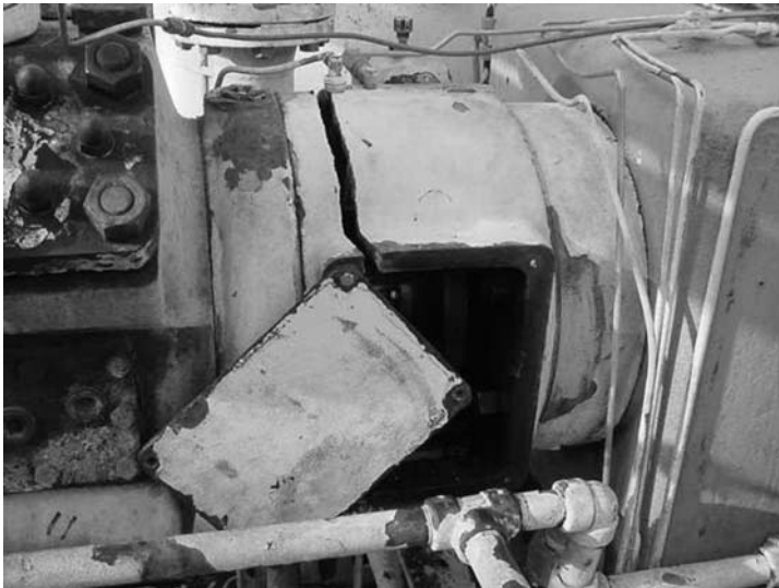
Figure 11-15. Reciprocating Compressor Showing Failed Distance Piece.
