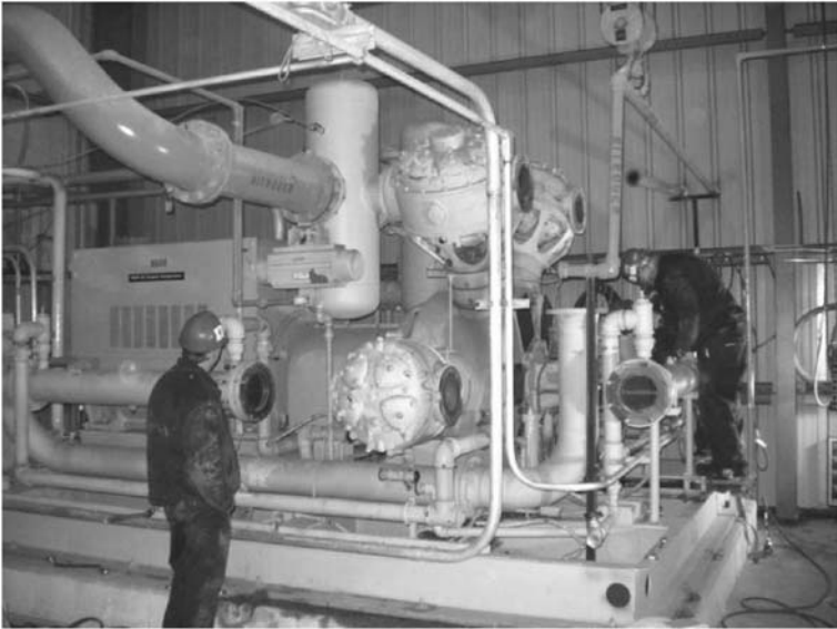
Figure 13-30: Prior to reconfiguring, this oversized 3-stage Joy WB14 nitrogen compressor required 76% of the flow to be recycled.
