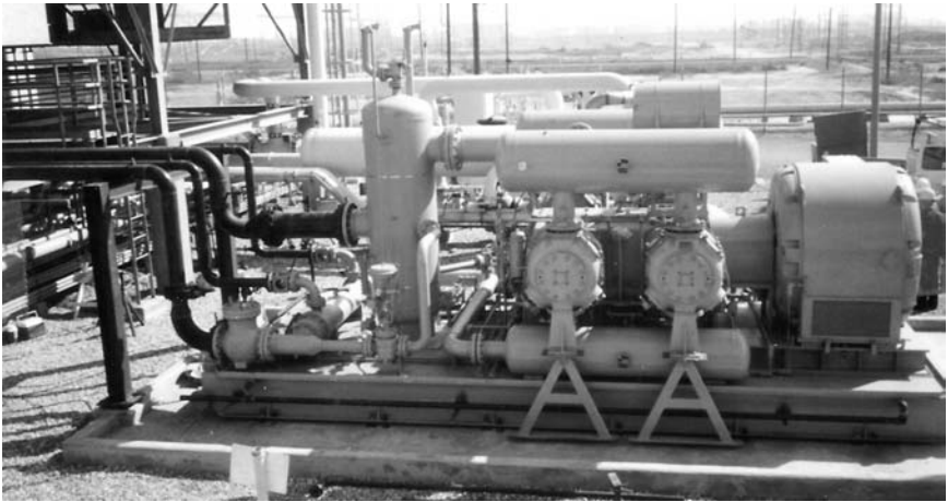
Figure 12-2. Electric motor-driven reciprocating fuel gas booster compressor package
