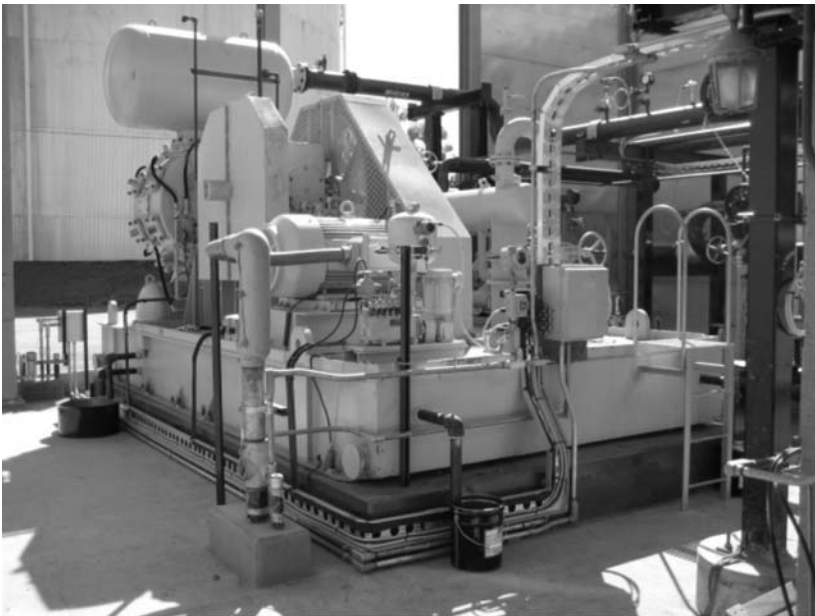
Figure 3-41. Worthington HB GG 24 x 13 Single-stage Compressor after overhaul. Compliments of Sun Engineering Services, Inc., and Power & Compression Systems Co.
