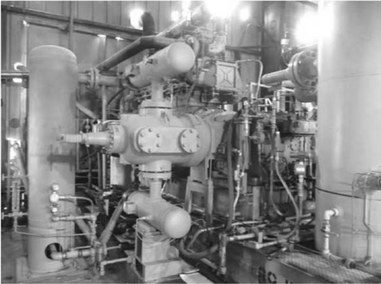
Figure 13-29: Obsolete KOCA/2 frame with new Ariel cylinders applied.
