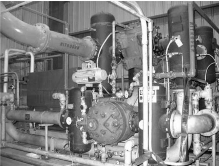
Figure 13-31: The reconfigured unit was sized to meet the process requirements without significant recycled flow.
