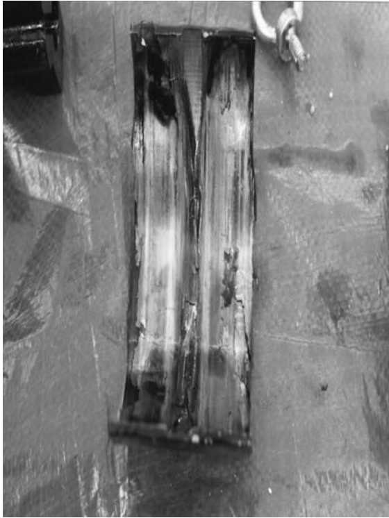
Figure 11-18. Reciprocating Compressor Hydrodynamic Bearing Shoe Showing Distress Following Bearing Failure.
