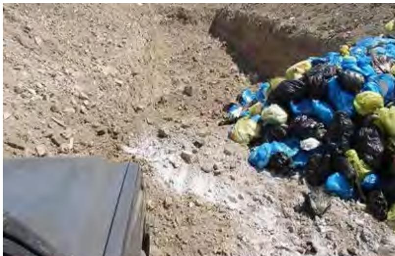
**Figure 14.2** Special cells or trenches for disposal of biocontaminated wastes in a municipal dumping site (10 m long, 3 m wide and 2 m deep)
