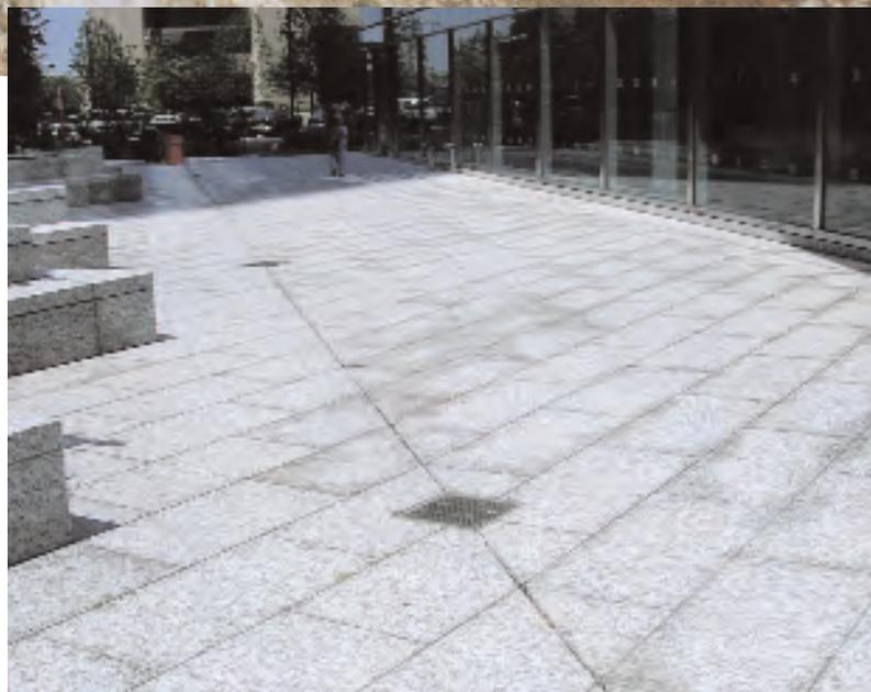
*Moisture damage on exterior floor slabs.*
