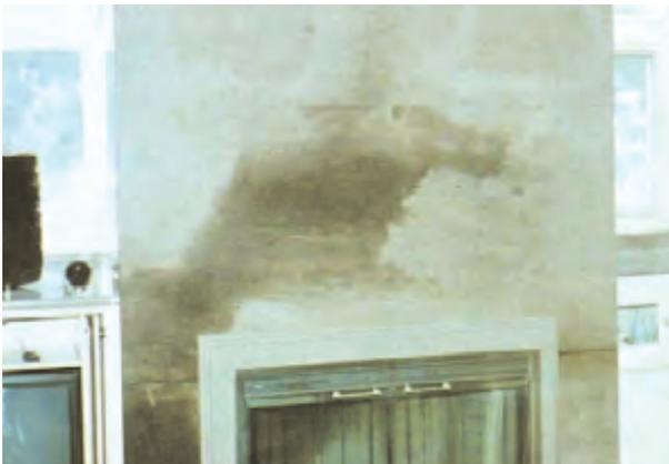
*Wet stone on granite fireplace from a leak in chimney.*
