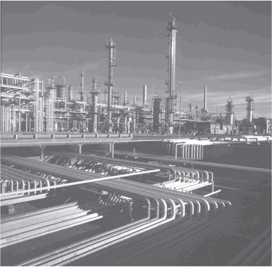
Fig. 19.1 Piperack junction
