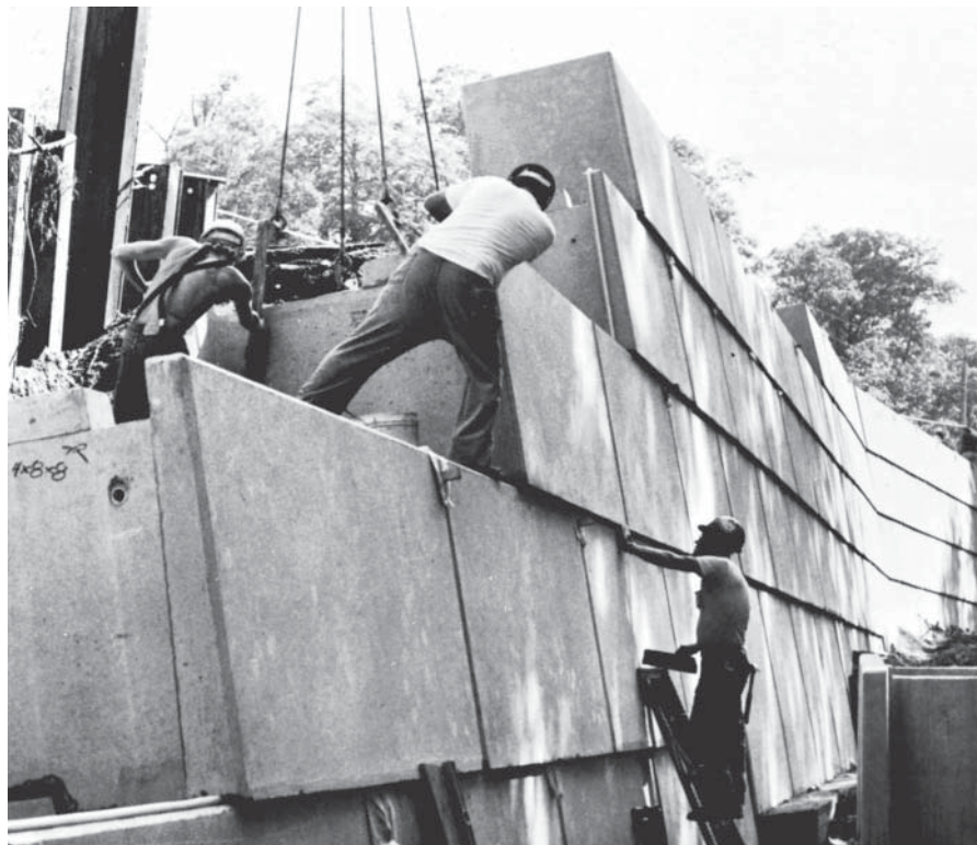
Retaining wall for Long Island Railroad, Huntington, New York. Constructed with precast interlocking reinforced concrete modules.
