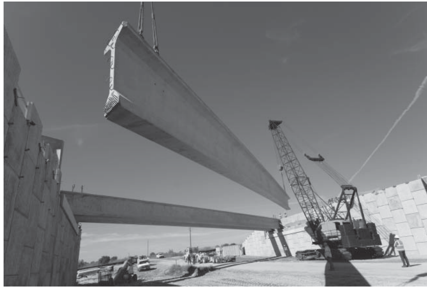
Prestressed bridge girders during erection.
