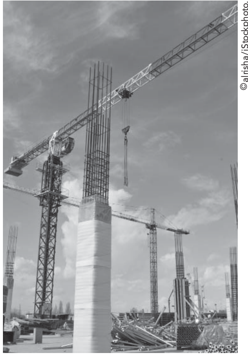
Reinforced concrete columns.
