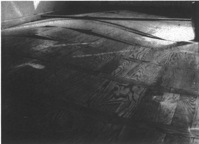
Figure 10.5 Effect of swelling deformations in a wooden floor due to lack of movement gaps at the edges
