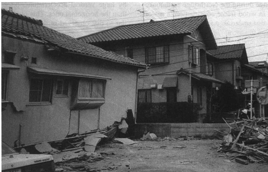
Figure 15.6 Three undamaged modern wood-frame buildings in the background and a collapsed older building in foreground in Nishinomiya, Japan (Photo credit: Hans Rainer. Reproduced by permission)
