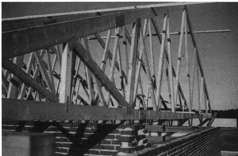
Figure 16.22 Trusses made with nail plates
