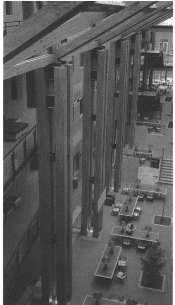
Figure 21.8 Parallam composite columns with discontinuous steel packs connections at UBC, Faculty of Forestry, Vancouver, Canada
