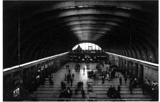
Figure 1.12 Glulam arch roof for Stockholm central railway station, built 1925. Reproduced by permission of Svenskt Limträ AB
