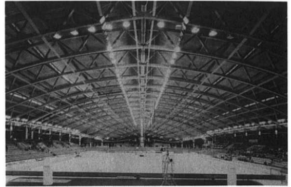
Figure 16.13 Ice skate rink with trusses with doweled joints. Moelven Glulam (Reproduced by permission of Erik Aasheim, NTI)
