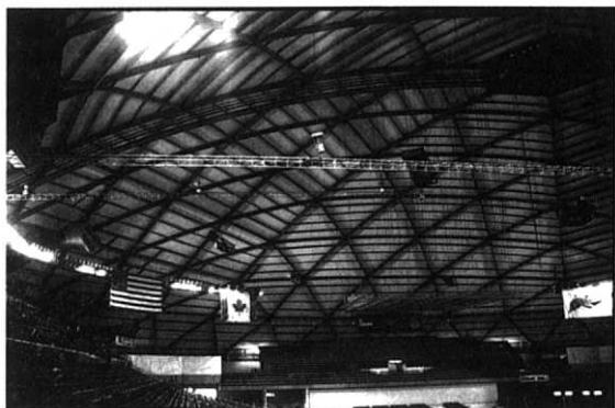
Figure 1.19 Interior from the Tacoma Dome, Washington, USA with a 162 m span (Photo: Sven Thelander-sson)
