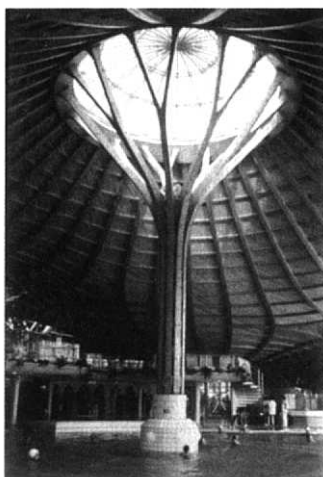
Figure 1.20 Glulam roof for a swimming hall in Bad Durrheim, Germany, built 1987 (Reproduced by permission of Arge Holz, Dusseldorf)
