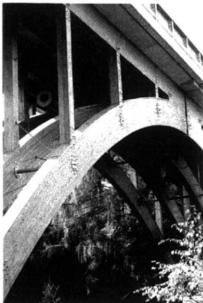
Figure 1.22 Europabrücke, Murau, Austria, built 1993. Glulam structure with concrete bridge deck (Reproduced by permission of Holger Gross)
