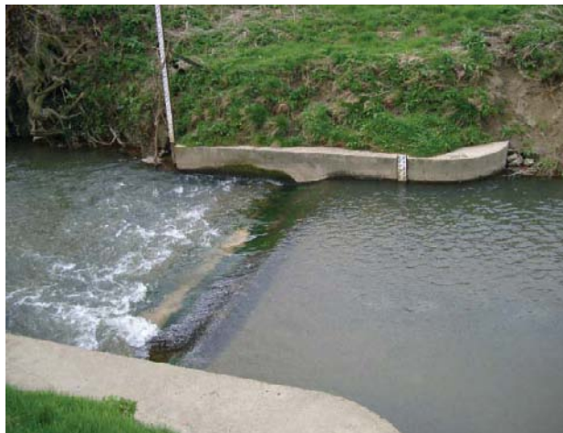
Figure 3 A river weir in the River Brue, SW England
