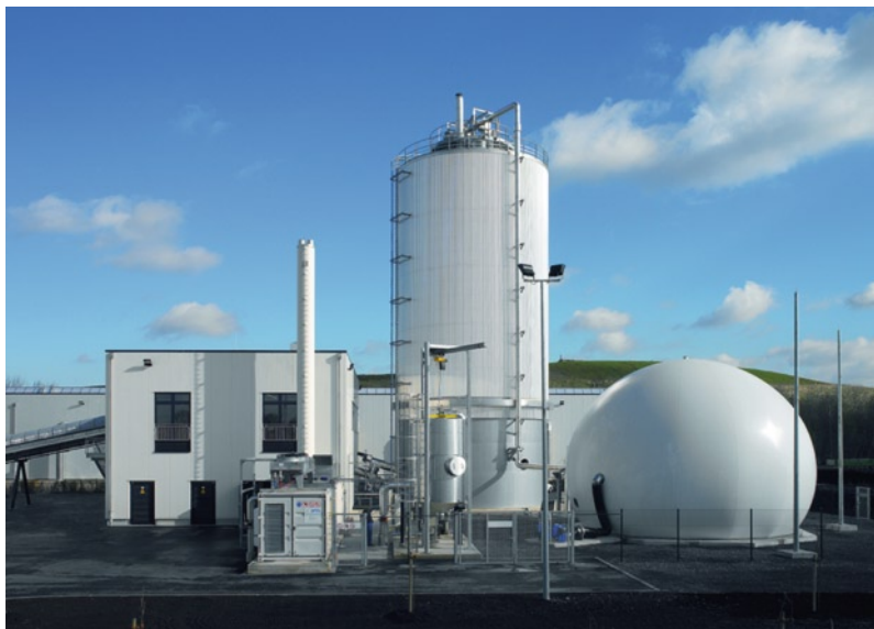
Fig. 7.16 A DRANCO plant at Münster (Germany) which treats 24,000 tonnes per year, of MSW (photo courtesy: Organic waste systems n.v.)
