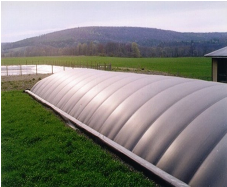
Fig. 5.11 Plug-flow digester (Photo courtesy: AgSTAR)
