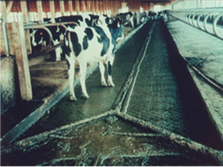
Fig. 5.12 Chain drag alley for scraping manure (Photo courtesy: AgSTAR)
