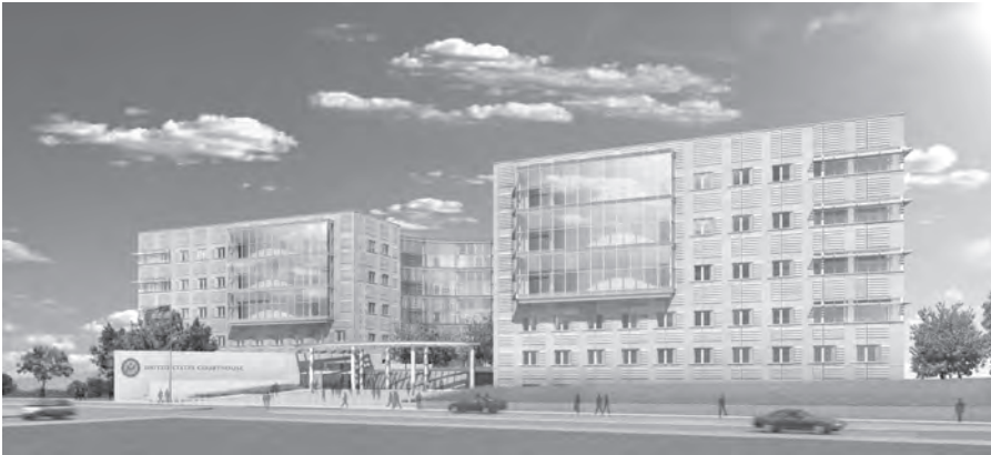
FIGURE 9-10-1 Front facade and entrance to the Jackson Mississippi Courthouse.
