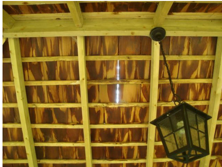
GAP IN SHINGLES TO GAZEBO ROOF
