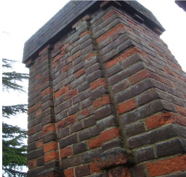
WEATHERED BRICKWORK TO FRONT LEFT HAND CHIMNEY
