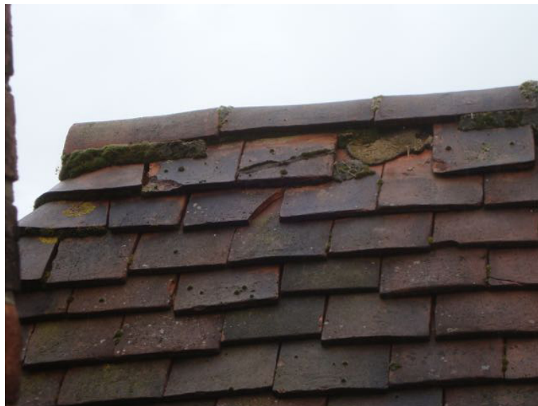
TYPICAL EXAMPLE OF DEFECTIVE TILING TO ROOF AND RIDGE
