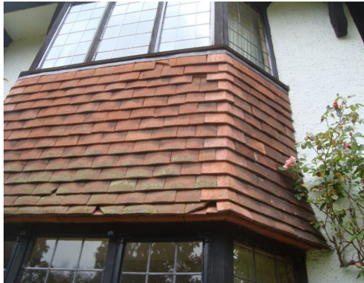
DEFECTIVE TILING HANGING TO LEFT HAND REAR BAY
