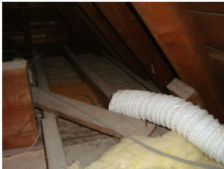
SECOND FLOOR BATHROOM EXTRACT DUCT VENTING INTO ROOF SPACE (LACK OF INSULATION ALSO VISIBLE)
