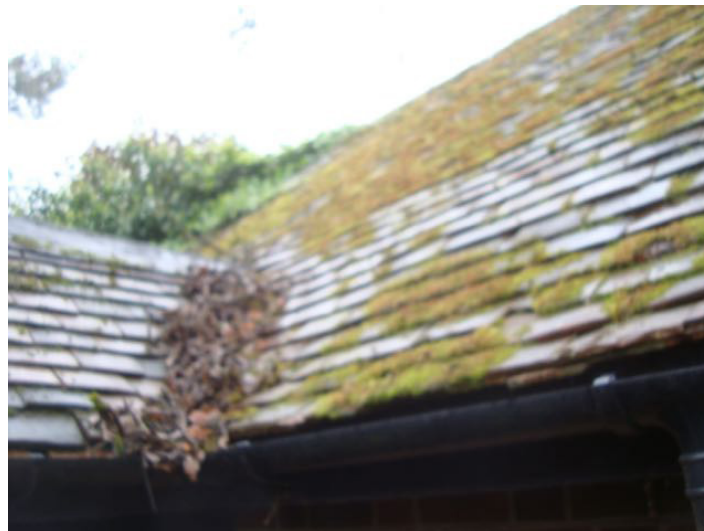
DEBRIS IN VALLEY AND MOSS ON OUTBUILDING ROOF
