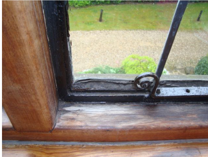
RUSTED WINDOW FRAME AND LOOSE PANE OF GLASS TO STORE WINDOW
