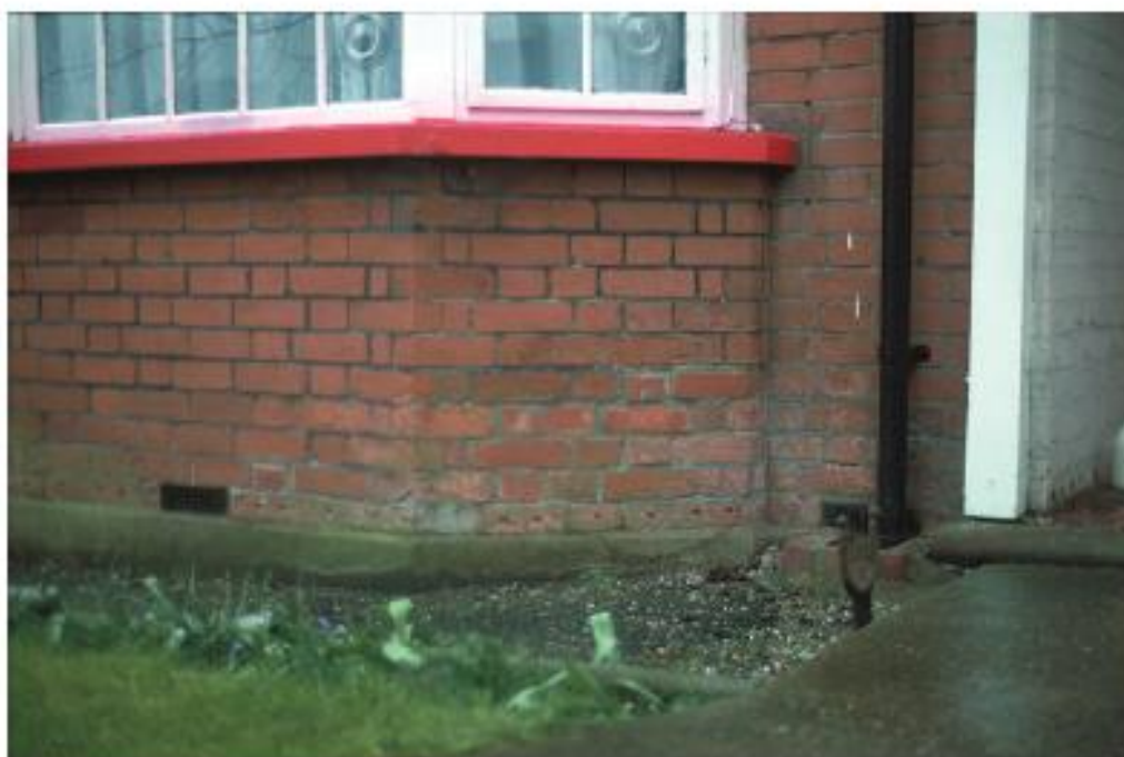
Fig. 4.7 Drill holes at the base of the wall indicate that a chemical injection damp-proof course has been added.
