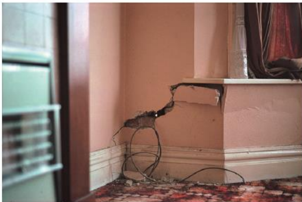
Fig. 3.11 Subsidence damage inside house.
