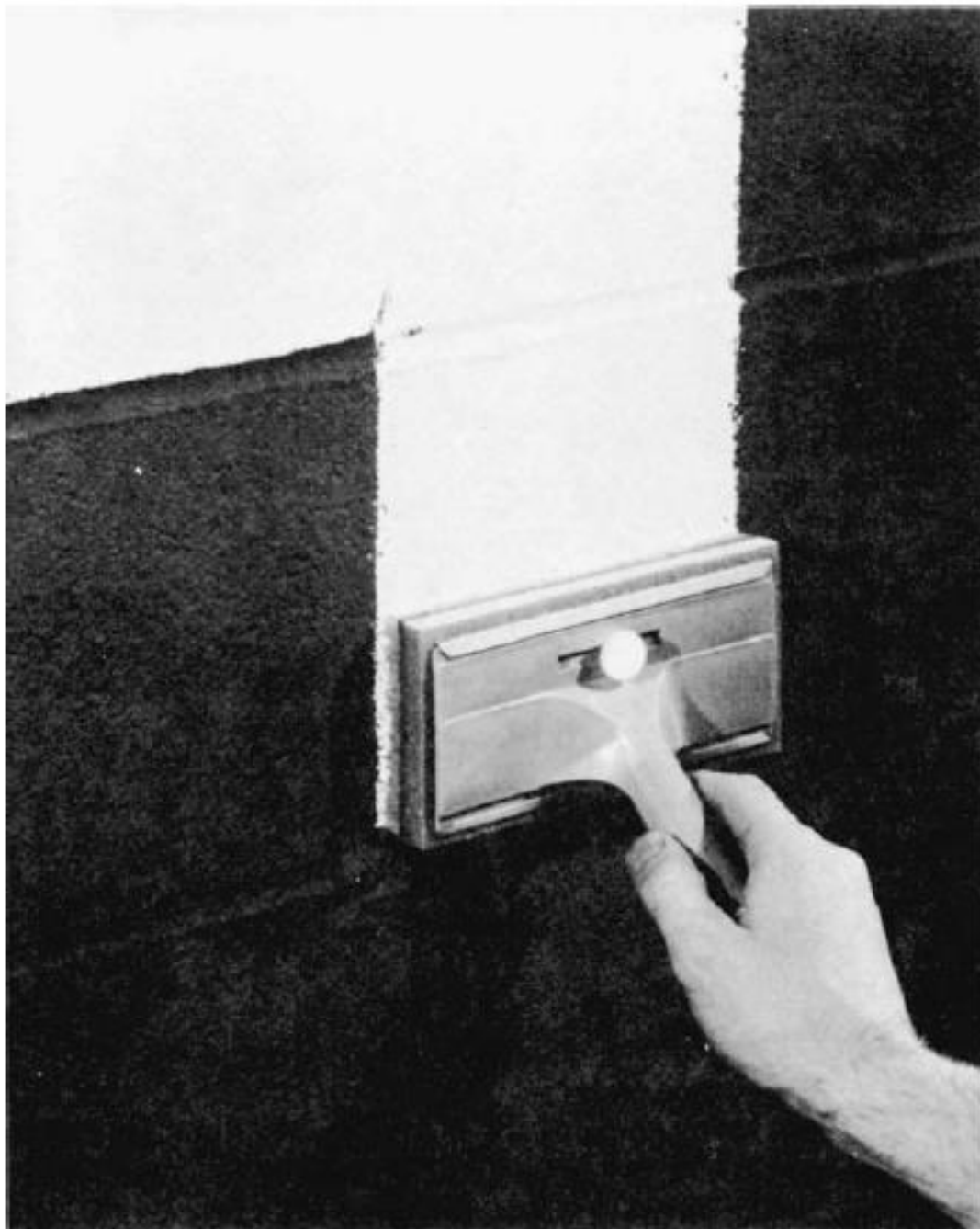
Figure 5-34 Block with V-joints. Block can be painted—pad painter works well on it.
