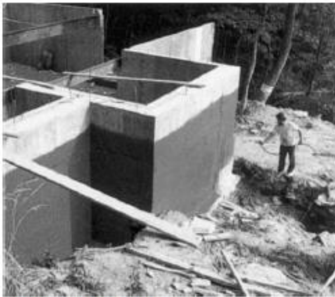
Figure 3-13 The Rub-R-Wall can be applied above or below ground level.
