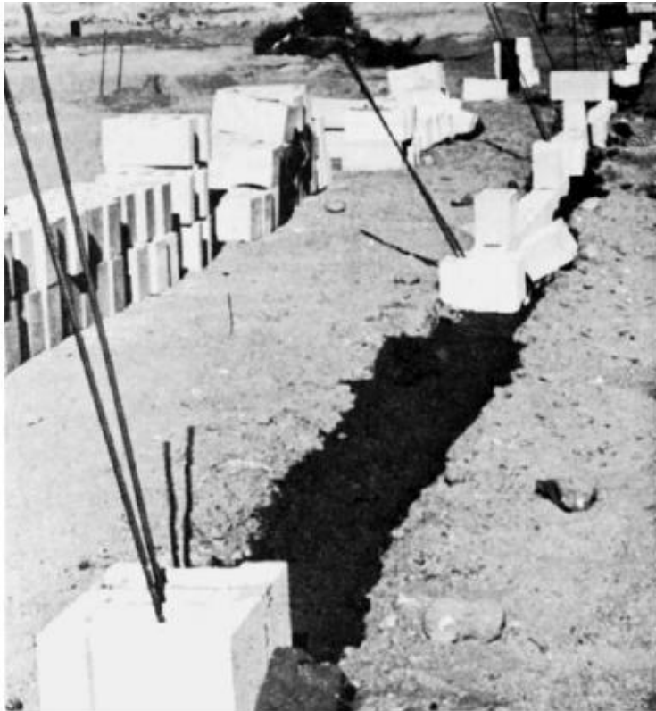
Figure 5-15 Vertical reinforcement rods through double-thick column blocks.
