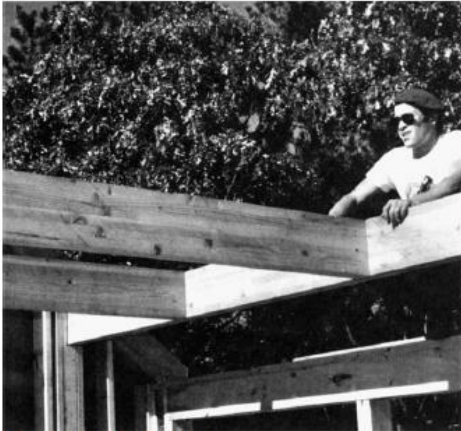
Figure 9-10 Glulam beam. (Courtesy Weyerhaeuser)
