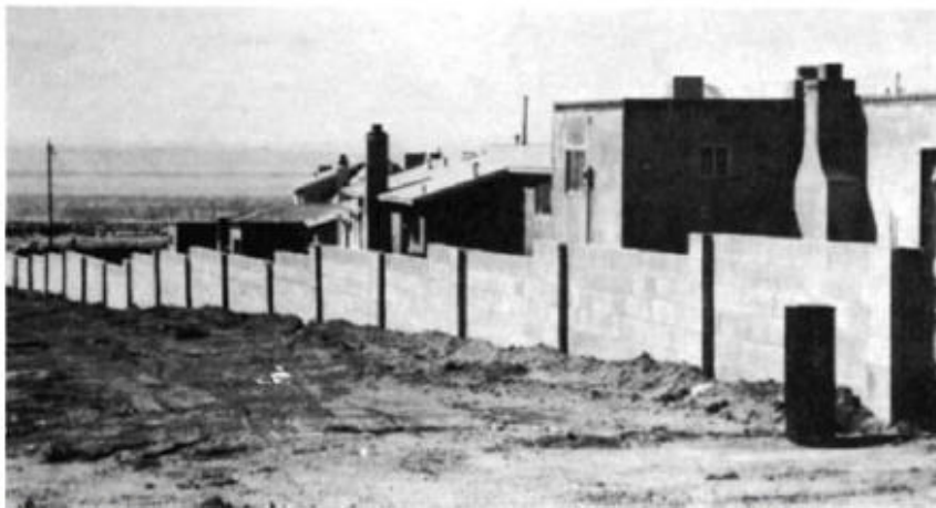
Figure 5-16 A newly finished concrete-block wall. Note reinforcement columns at various intervals.
