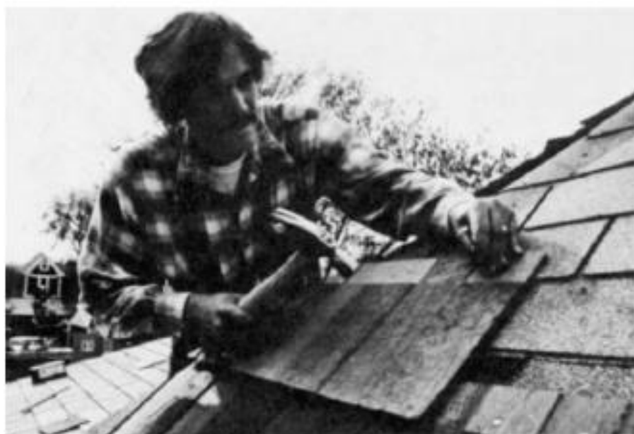
Figure 13-13 Wood fiber roofing from Masonite is a relatively new product. It is available in fire-rated versions and is bigger than standard shingles.
