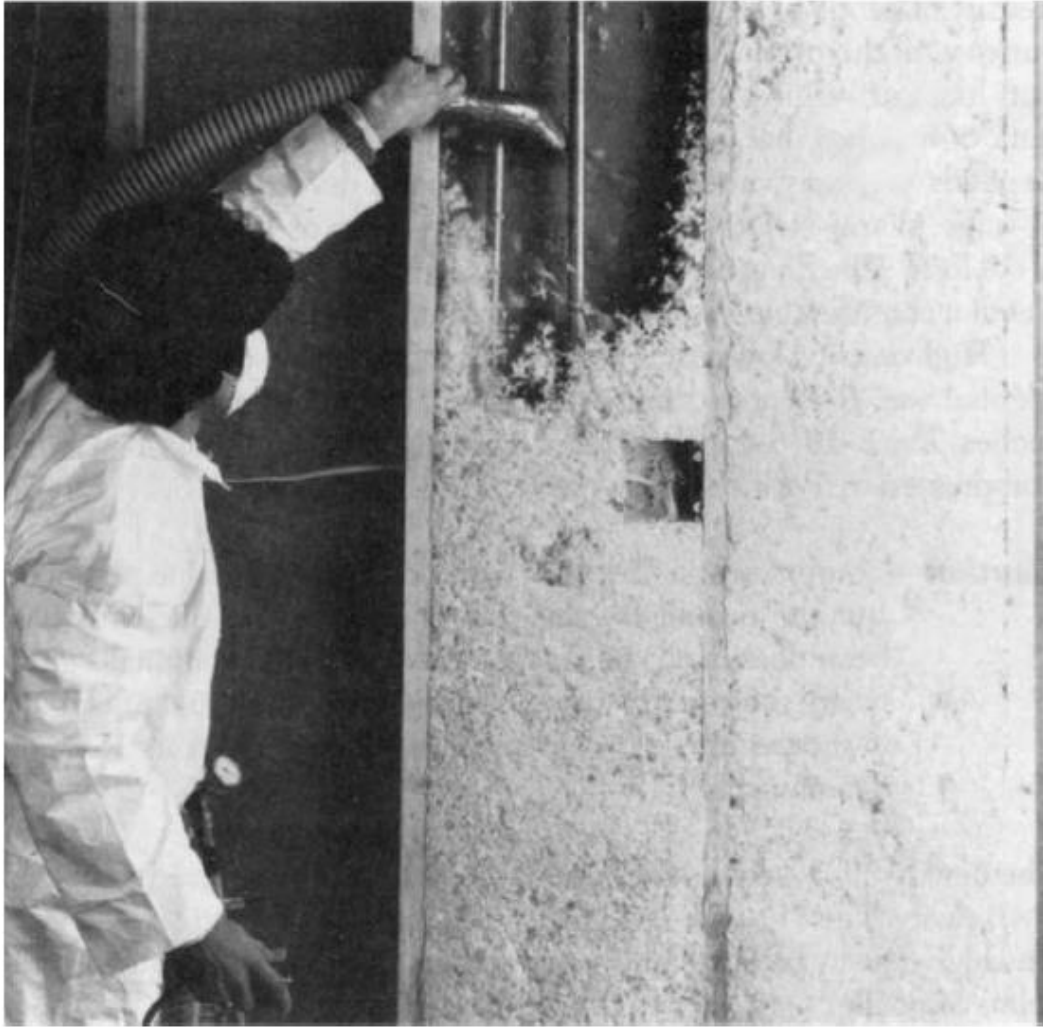
Figure 17-1 BIB Insulation being installed behind the nylon netting. (Courtesy Ark-Seal International)
