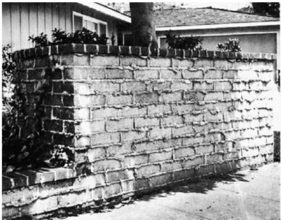
Figure 5-33 Brick wall with extruding joint construction.
