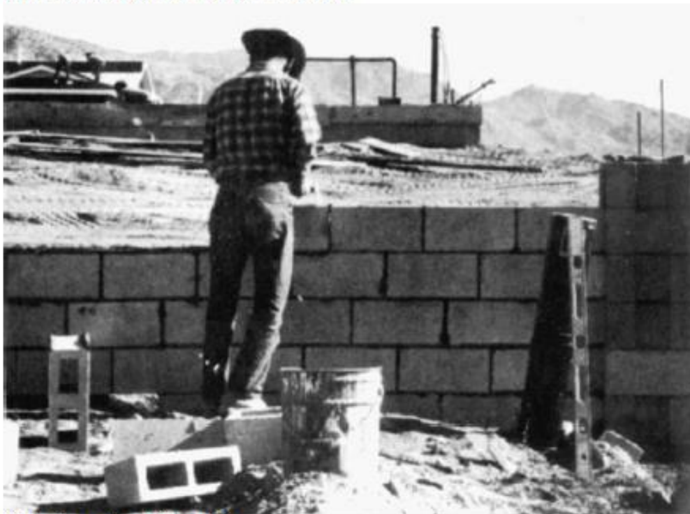
(B) Blocks are tapped into position.
