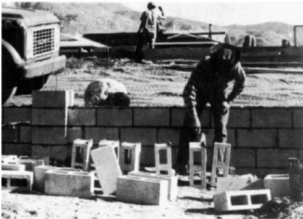
(A) Several blocks are receiving mortar on the end.
