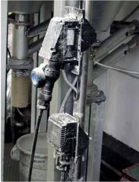
Example of dust Ex zone 21: Explosion-protected plug and socket and terminal box in the field
