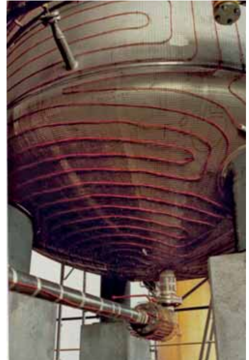
Example of a trace heating system
