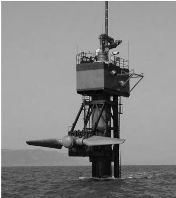
**Figure 13.6** SeaFlow with its rotors raised (Source: [http://en.wikipedia.org/wiki/Marine\\_Current\\_Turbines](http://en.wikipedia.org/wiki/Marine_Current_Turbines))
