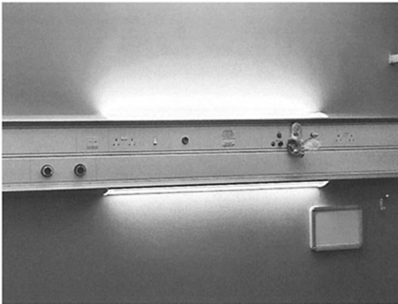
*Figure 11.8* Bedhead trunking (Courtesy of Cableflow Ltd)
