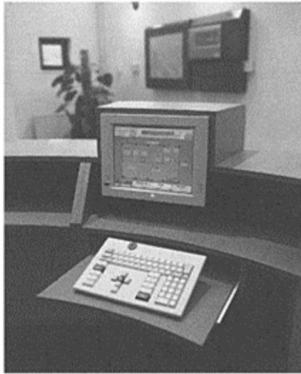
*Figure 10.5* Fire detection central station (Courtesy of Gent & Co. Ltd)
