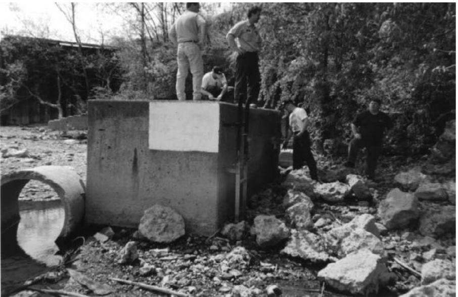
Field inspection crews inspecting a combined sewer overflow (CSO) diversion chamber located near Pittsburgh, Pennsylvania.
