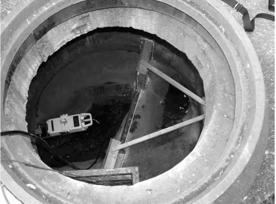
**Figure 10.1** Flowmeter and weir installation in a manhole for monitoring incoming and outgoing flows.
