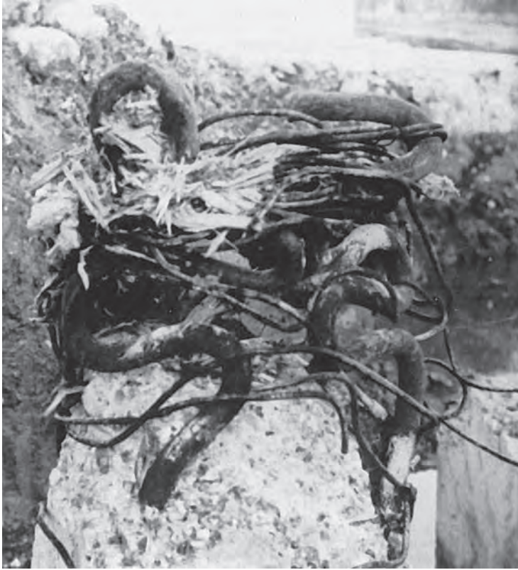
Figure 7.1 Damage to head of precast concrete pile. (Photograph courtesy of W. A. Dawson Ltd.)
