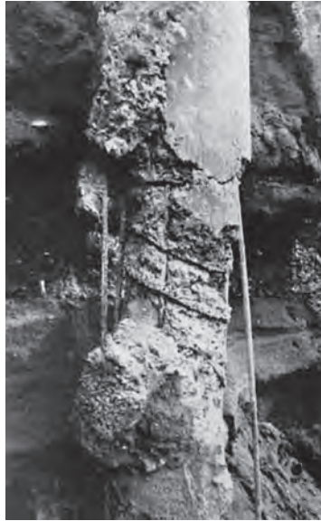
Figure 7.21 Defects associated with displacement of reinforcement. (Photograph courtesy of CIRIA, London.)
