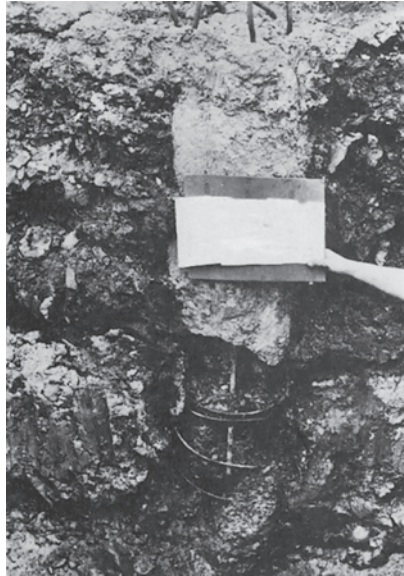
Figure 7.18 Erosion of wet concrete by groundwater flow: pile in fill. (Photograph courtesy of CIRIA, London.)
