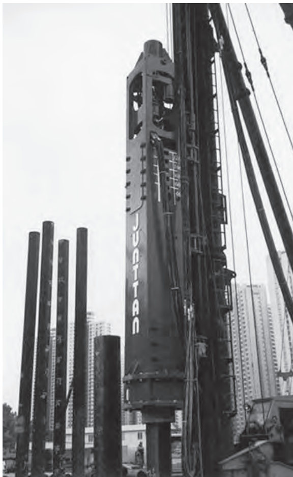
Figure 3.13 A Junttan hydraulic hammer driving steel piles. (Photograph courtesy of Junttan Oy.)
