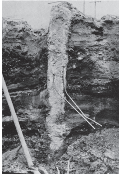
Figure 7.11 Separation of pile shaft caused by extraction of casing. (Photograph courtesy of CIRIA, London.)
