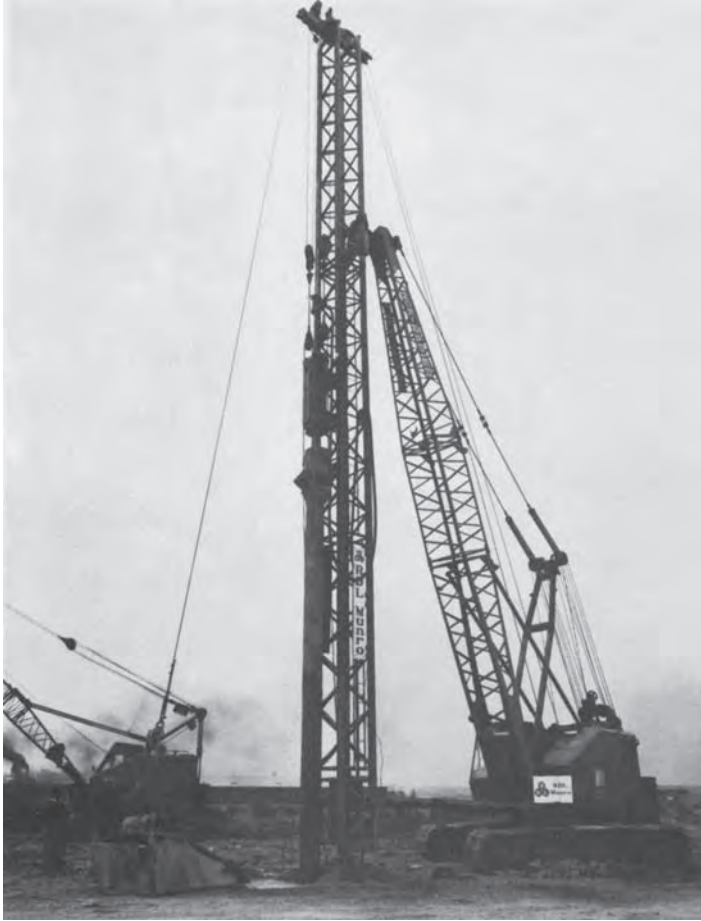
Figure 3.11 Pile driving rig with hanging leaders. (Photograph courtesy of RDL Munro Piling.)
