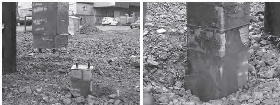
Figure 3.2 Detail of the 'Stent' pile joint. (Photographs courtesy of Stent Piling and Foundations.)
