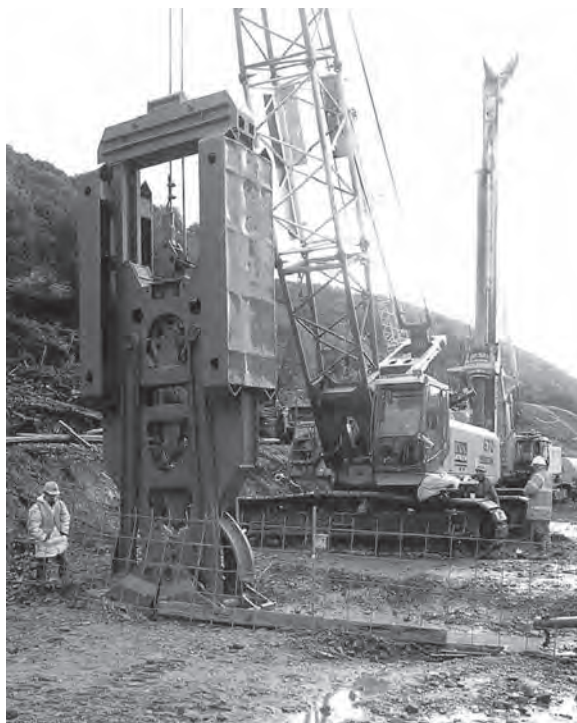
Figure 3.27 Heavy diaphragm wall grab in use for barrette construction. (Photograph courtesy of Carillion Piling.)
