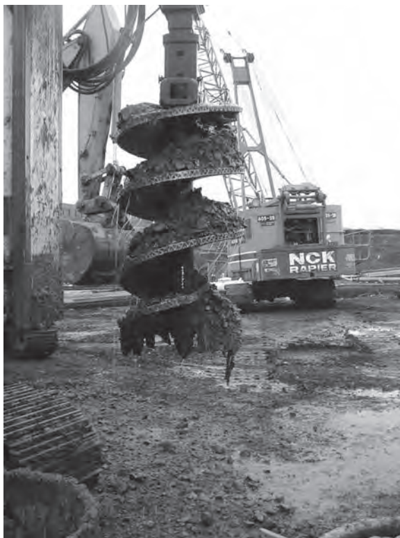
Figure 3.26 Polymer strands attached to excavated spoil on an auger. (Photograph courtesy of Carillion Piling.)
