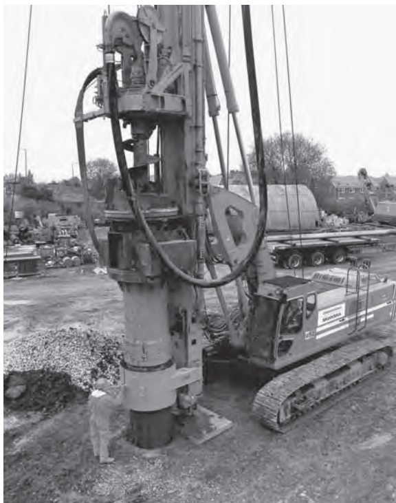
Figure 3.31 Heavy-duty CFA rig with casing. (Photograph courtesy of Cementation Foundations.)
