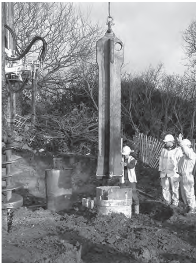
Figure 3.19 Heavy chisel for breaking obstructions. (Photograph courtesy of Carillion Piling.)
