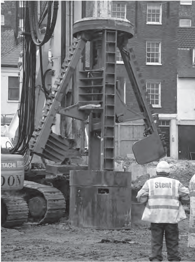
Figure 3.20 An underreaming tool in the open or working position. (Photograph courtesy of Stent Piling.)
