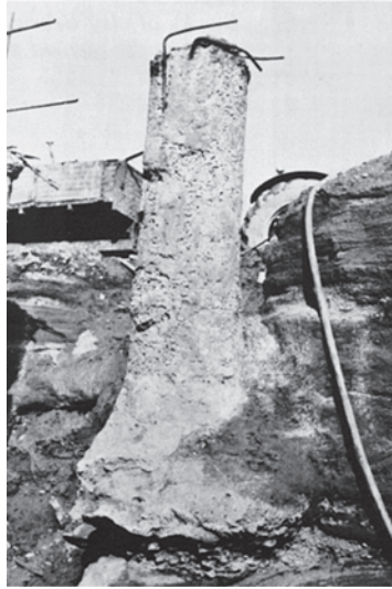
Figure 7.6 Bulbous projection on pile shaft caused by overbreak. (Photograph courtesy of CIRIA, London.)
