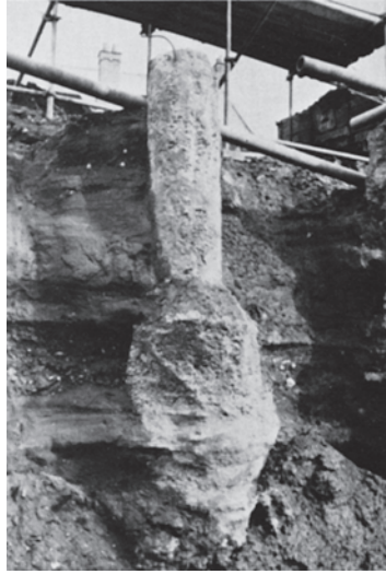
Figure 7.15 Defect caused by concrete slumping into a dry cavity. (Photograph courtesy of CIRIA, London.)
