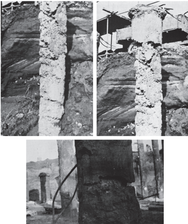
Figure 7.10 The effect of low slump concrete. (Photographs courtesy of CIRIA, London.)
