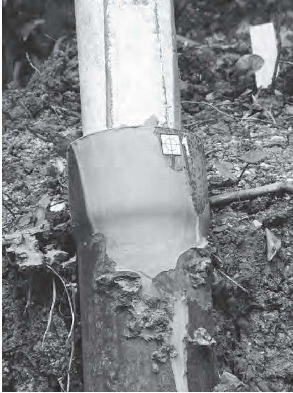
Figure 3.41 Small diameter (150 mm) Grundomat pile with hollow structural steel section centrally grouted in place.
