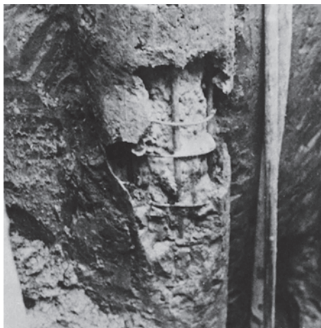
Figure 7.13 Defect in pile shaft caused by water. (Photograph courtesy of CIRIA, London.)
