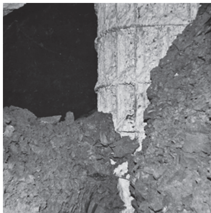
Figure 7.20 Concrete retained by reinforcement cage in underreamed pile. (Photograph courtesy of CIRIA, London.)
