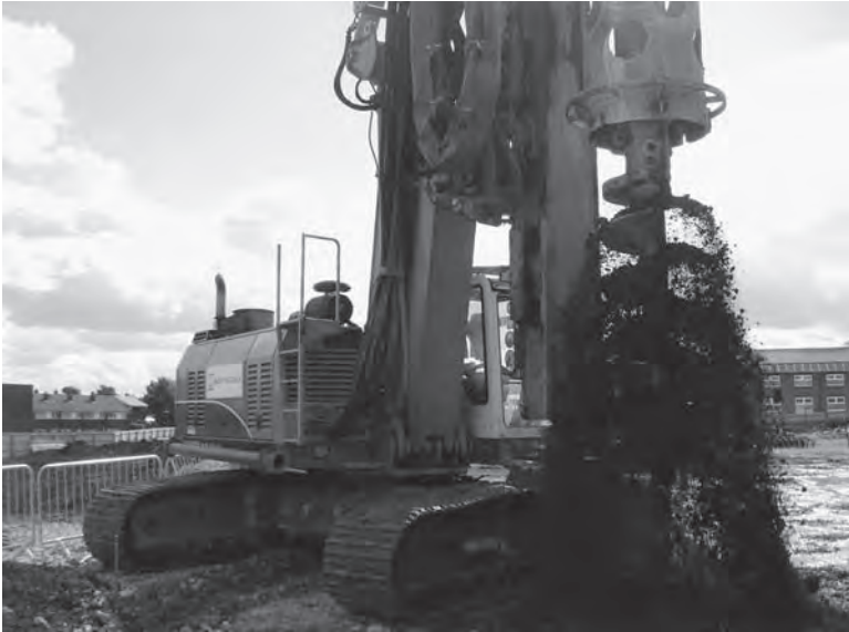
Figure 3.17 Auger rig 'spinning off' spoil. (Photograph courtesy of Bauchy-Soletanche.)
