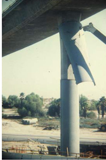
Figure 9.18 Column retrofit using steel casings. (Source: Courtesy of Michael Keever)
