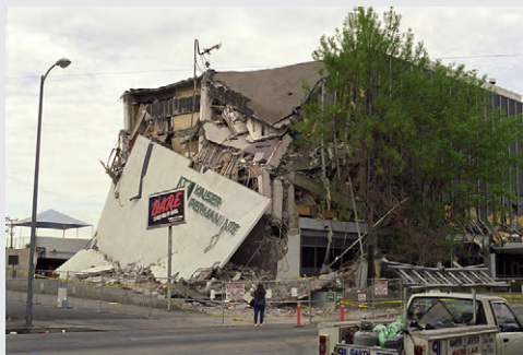
Figure 11.5 Damage to Kaiser Permanente Building after Northridge 1994 Earthquake.
