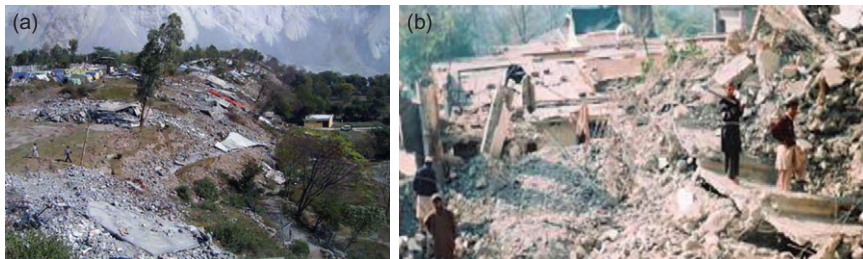
Figure 7.1 (a) Houses along the terrace rim and on flatland, north of Muzaffarabad, with cracks opening along the rim; (b) post-disaster debris disposal.
