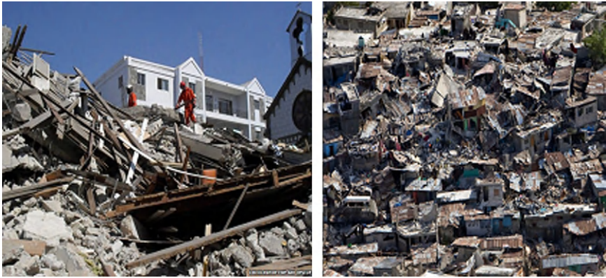
Figure 4.2 Examples of failure of poorly designed versus well-designed buildings.
