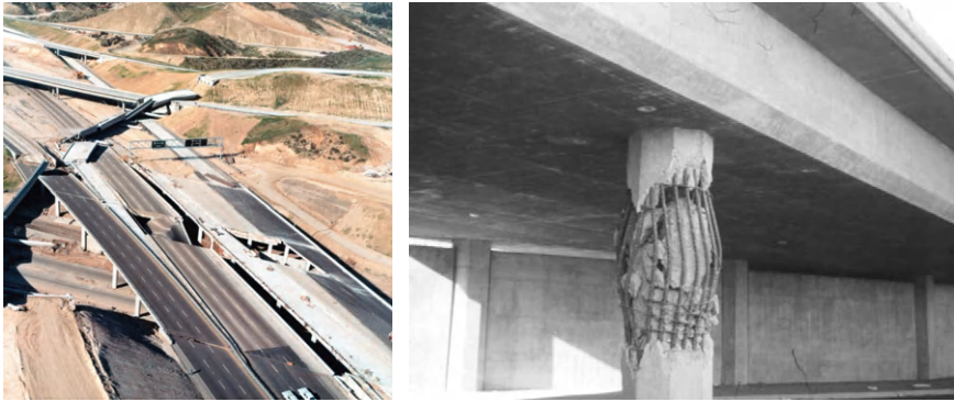
Figure 4.4 Two examples of damage caused by the San Fernando earthquake.
