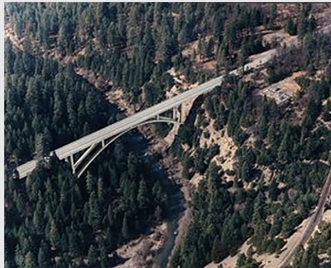
Figure 9.6 Long-span concrete arch Spanish Creek Bridge in California.
