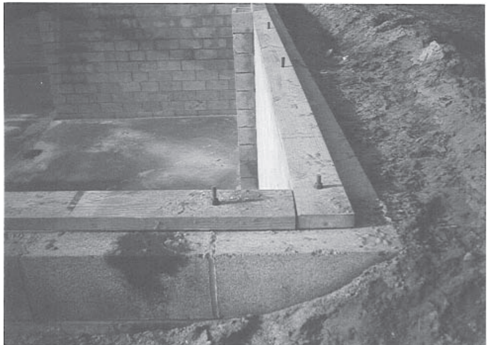
Figure 17–1. Sill plate.
