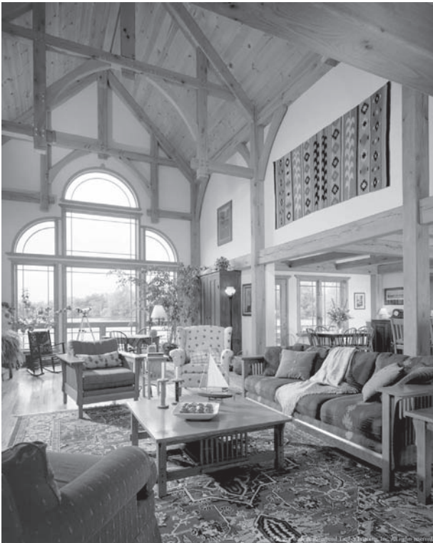
Figure 15-12. The exposed timber framing in this house is an important part of its design. Courtesy of Riverbend Timber Framing, Inc. Photo by Roger Wade.
