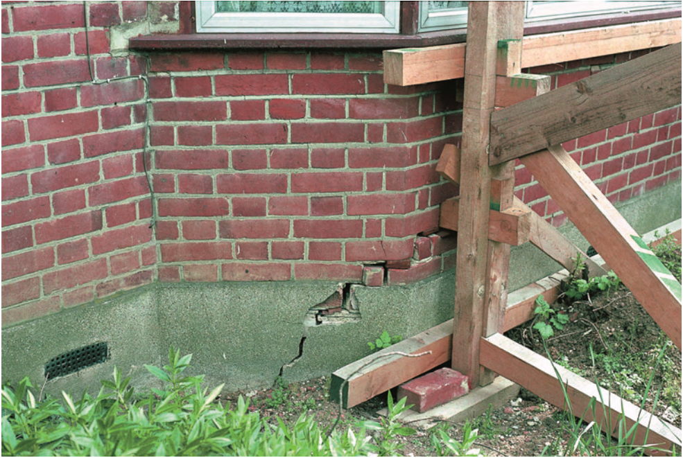
Fig. 3.12 Subsidence damage outside house.
