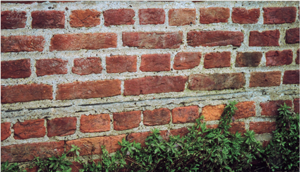
Fig. 4.14 Hand made red facing bricks set in lime mortar to English Bond with a two-course slate damp proof course. Good ground clearance below the damp proof course.
