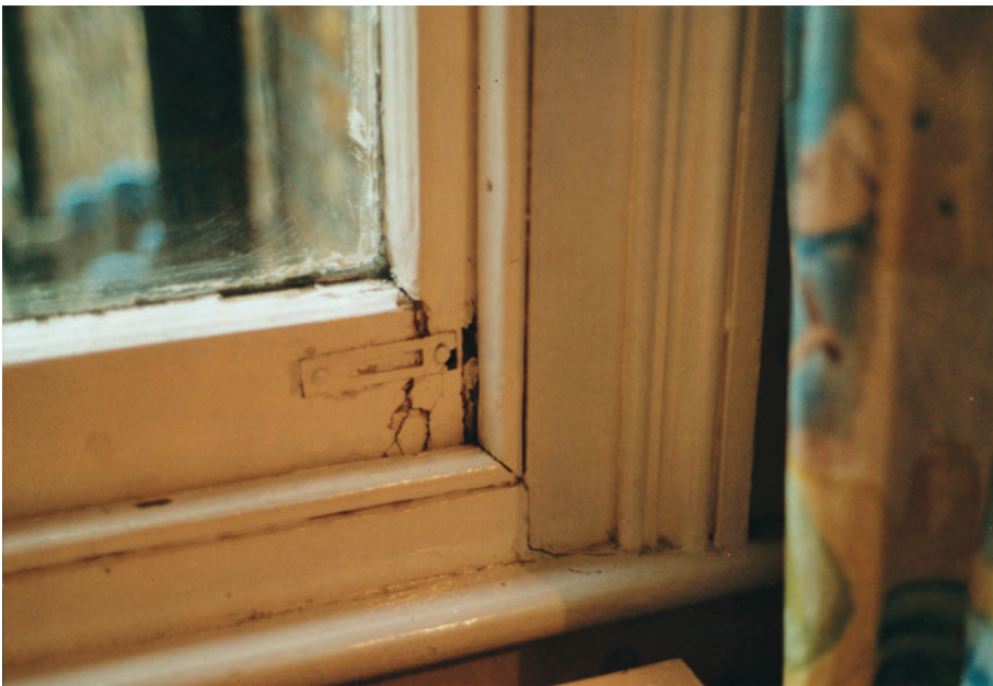
Fig. 18.5 Significant expenditure on repairs or replacements of window frames will be needed prior to the next redecoration.
