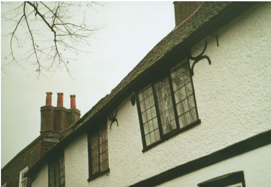
Fig. 21.5 The wall around this window leans out and has been restrained by the use of tie bars with the painted tie bar plates used as an added decorative feature. The tie bars will only work if the steel rods are in good order and very firmly secured at the other end.
