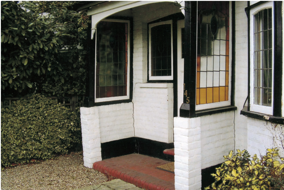
Fig. 3.16 Builders will often use a very shallow foundation for a porch thinking that because the weight is low they do not need to excavate as deeply as for the main house; this is not so and the porch in this case will need to be rebuilt on deeper footings.
