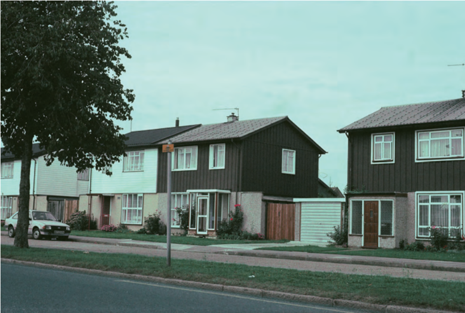
Fig. 4.12 BISF (British Iron and Steel Federation) Houses.
