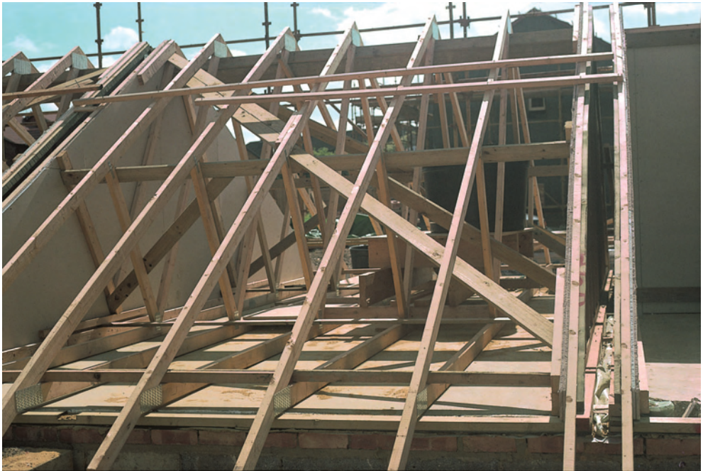
Fig. 6.3 Modern gang-nailed trussed rafter roofs require diagonal bracing and gable-end strapping to prevent racking.
