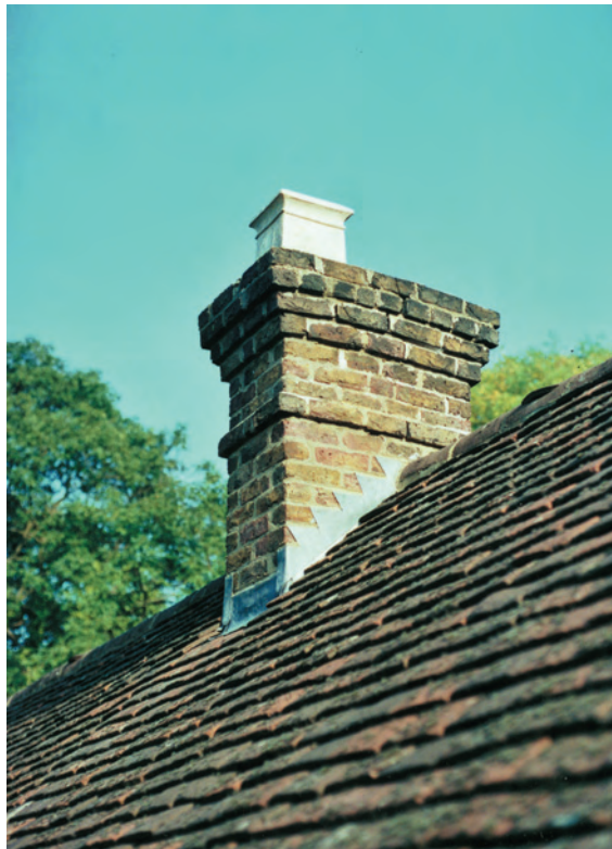
Fig. 6.2 Traditional lead flashings are fixed by plumbers, not roofing contractors, this being part of the plumber's trade.
