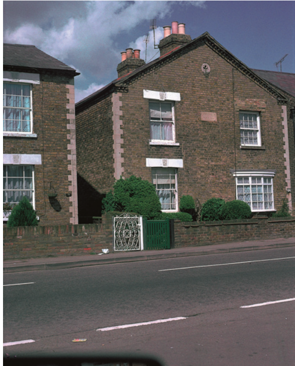
Fig. 21.4 The arch over first floor window has spread and the lintel has dropped. This section of wall will need to be rebuilt.
