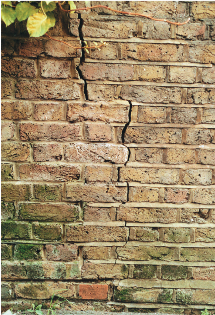
Fig. 3.15 Settlement or subsidence again with the crack widening with height.
