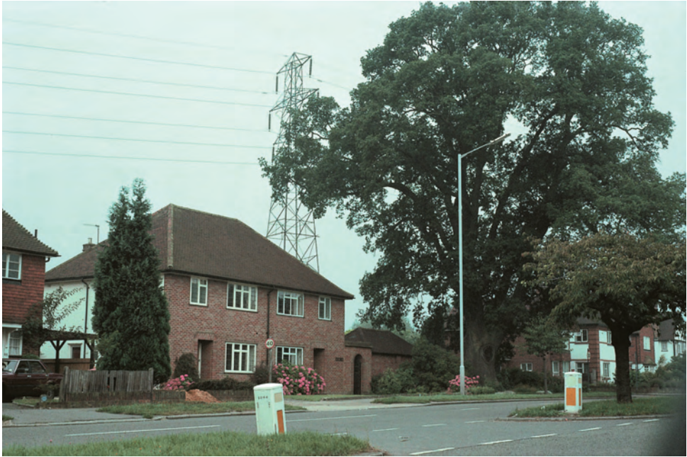
Fig. 2.2 The huge oak tree almost touches the garage wing to this house and there are a pylon and overhead power lines close by, both matters to be reflected in the report.
