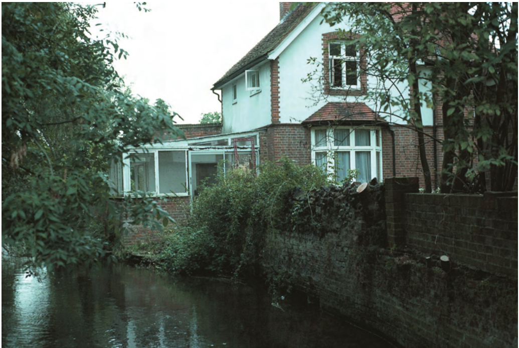
Fig. 2.1 This house is built directly on the riverbank. Issues arising include foundations, potential riparian liabilities and flood risk.
