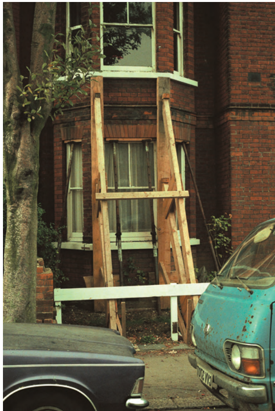
Fig. 4.1 Raking shores used to support bay suffering from subsidence pending repair. Note the tree.
