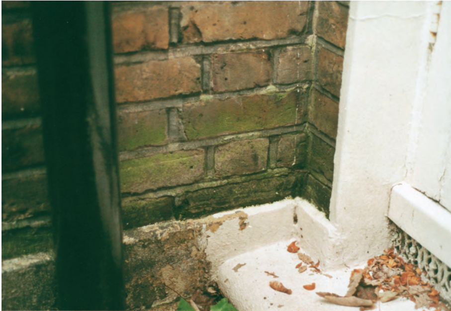
Fig. 18.6 Green algae and moss growing at the base of a wall due to gutter splash.
