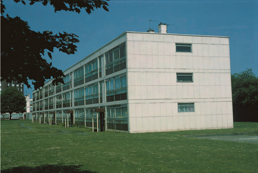
Fig. 13.1 Flats system built in the 1960s using pre-cast concrete panel construction. This construction may be unacceptable as mortgage security for most mainstream mortgage lenders.
