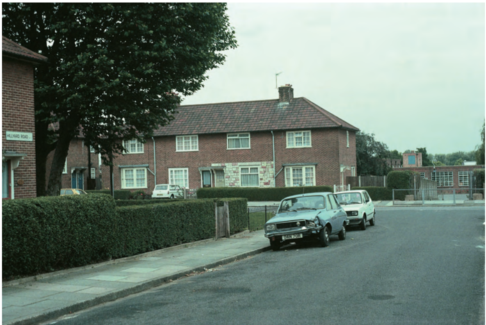
Fig. 2.3 Artificial stone cladding generally reduces the value of the property to which it is applied, and in this case by cladding only at ground floor level the owner has left a ledge for driving rain to penetrate behind the cladding resulting in a damp problem inside.
