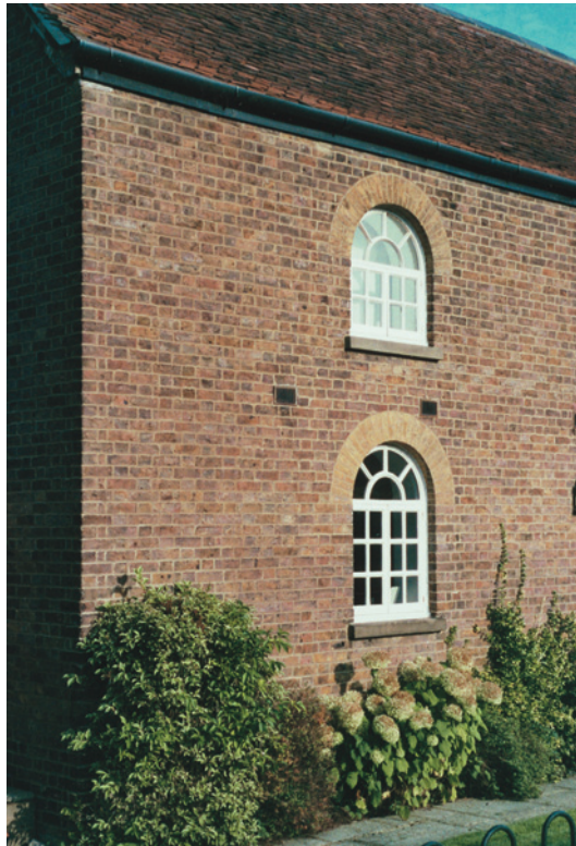
Fig. 21.3 London Stock brick set in lime mortar to Flemish bond. Properly formed arches are self-supporting and do not need lintels. Bricklayers who set out the corners are known as ‘corner men’ whilst those who infill with the main runs of brickwork are known as ‘line men’. Corner men are the most experienced and the final appearance of the wall depends very much on their skill.
