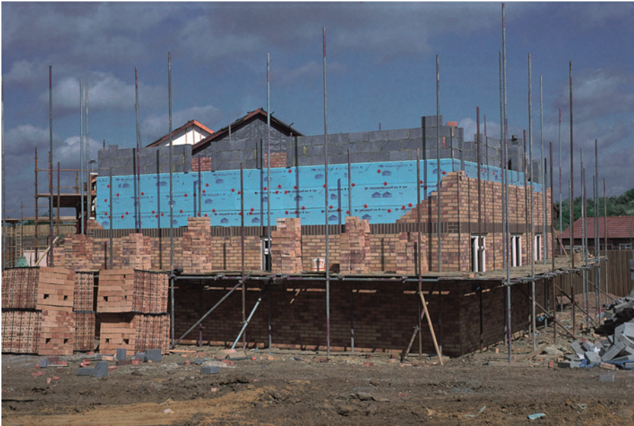
Fig. 7.2 A traditional brick and block house under construction in the same estate as the house in Fig. 7.2.
