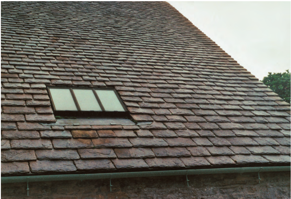
Fig. 6.1 Cotswold stone roof with skylight and lead apron. Careful attention to detail is needed if leakage around skylights is to be avoided.
