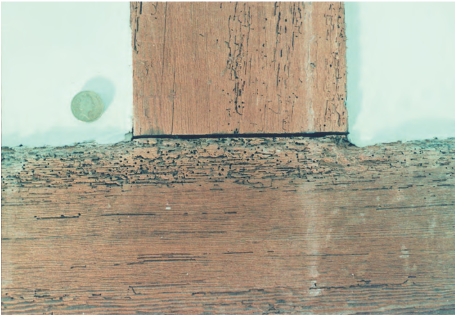
Fig. 7.3 Flight holes of the common furniture beetle ( Anobium punctatum ) in relation to a £1 coin.
