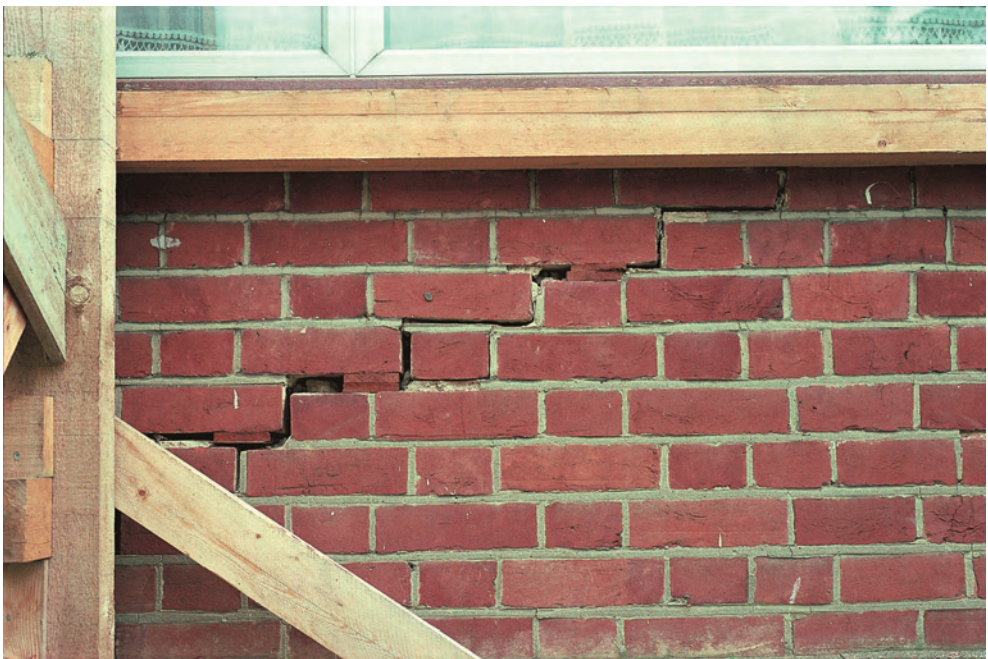
Fig. 3.14 Subsidence has affected the lower part of this wall. As a temporary measure raking shores have been placed against the wall and hardwood wedges driven into the open bed joints to prevent further movement of the construction above.
