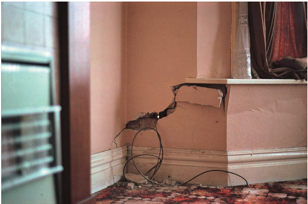
Fig. 3.11 Subsidence damage inside house.
