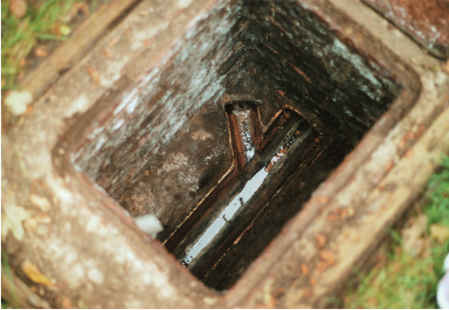
Fig. 18.8 One hundred years old drains. Drain flow satisfactory.
