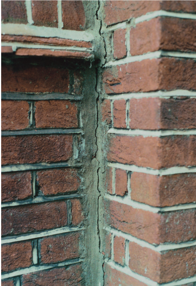
Fig. 3.4 This settlement fracture has been poorly repaired and opened up again indicating continuing movement.
