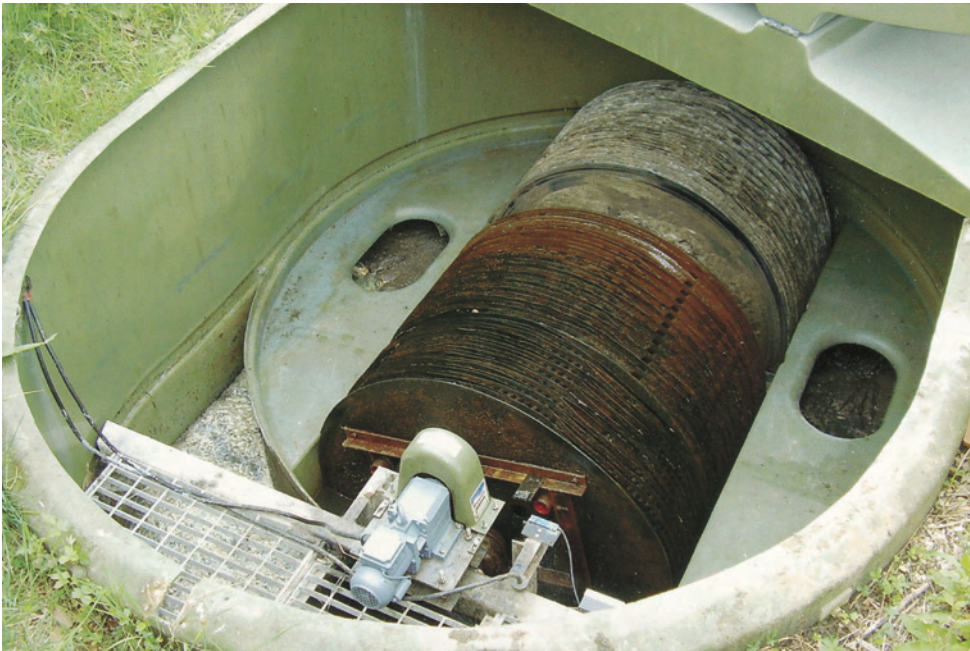
Fig. 9.3 When mains drainage is not available a modern alternative is the Klargester Biodisk septic tank drainage system. Effluent enters the system and is rapidly broken down by bacteria with the process hastened by the electric motor and rotating disks which increase the exposure to oxygen in the air. The treated effluent emerging from the system is clear water suitable for draining into soakaways or an adjoining water course. Consent to discharge effluent is required from the Environment Agency. Periodic de-sludging is necessary.
