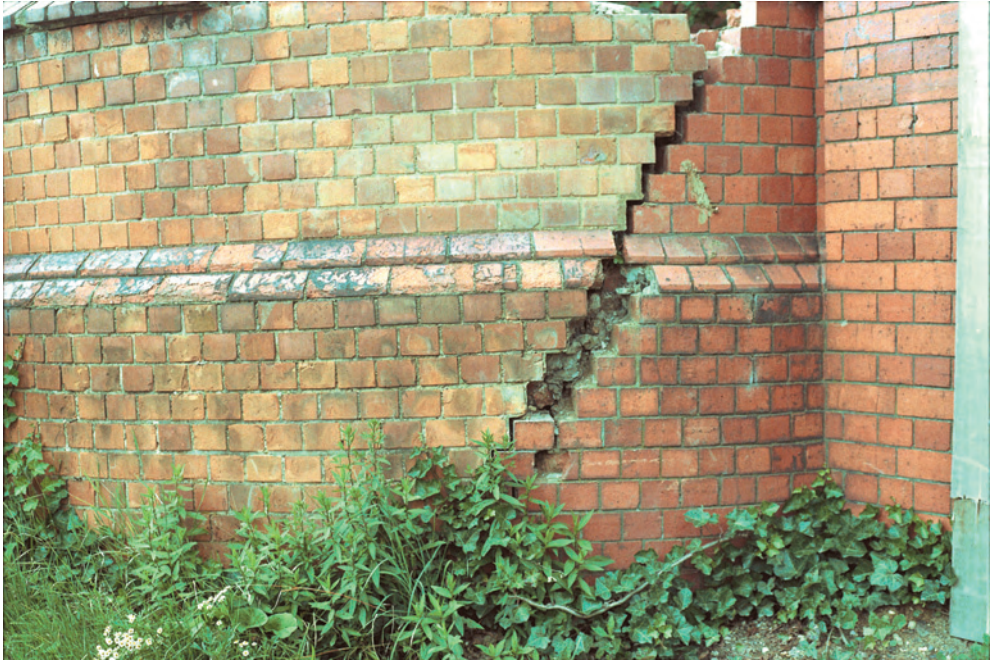
Fig. 3.10 Settlement or subsidence. The crack widens with height.
