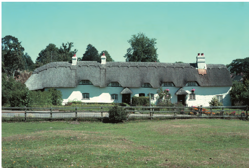
Fig. 6.4 Hampshire thatch with eyebrow window details.
