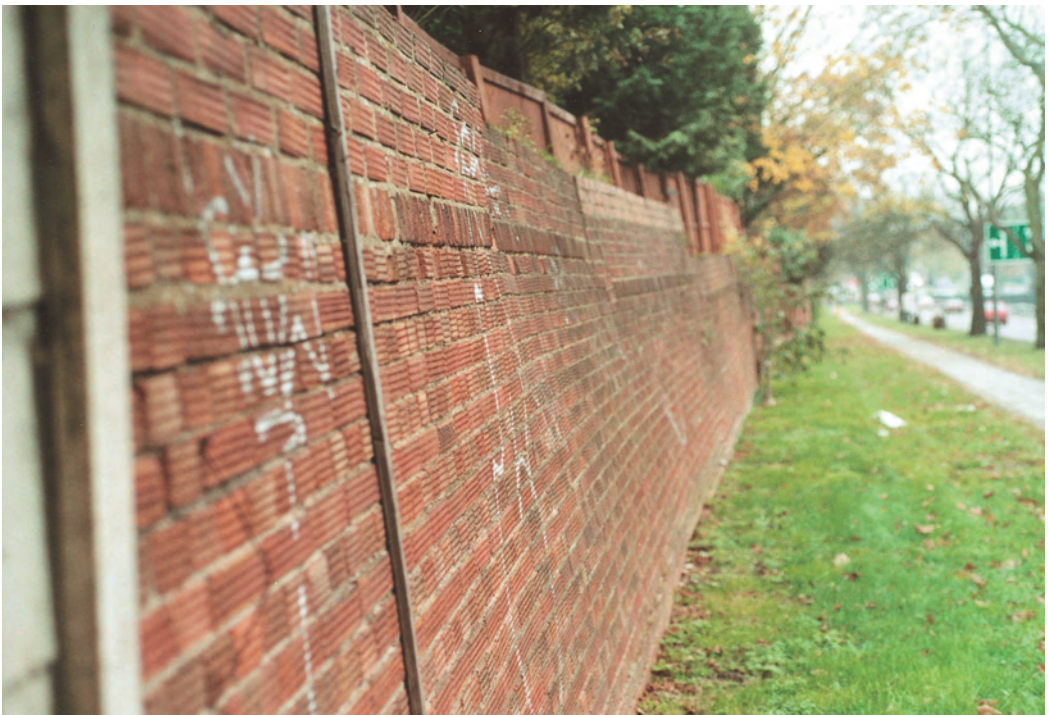
Fig. 2.4 If leaning boundary walls have to be rebuilt this can be very expensive.
