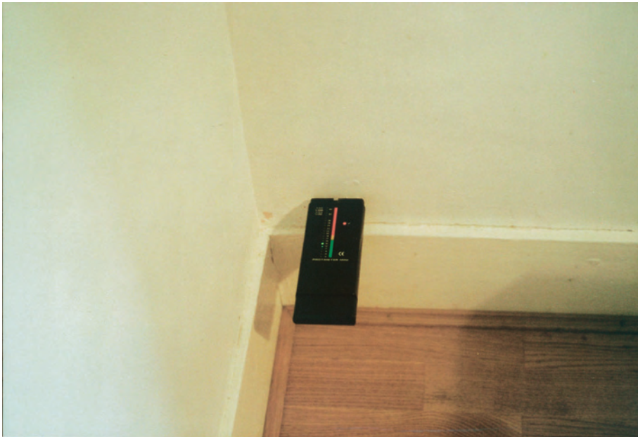
Fig. 18.2 Testing No. 1 Suburban Road for damp. The green light on the left indicates that the wall is dry. If the light moves up into the red sector it would indicate increasing levels of moisture in the wall plaster. This would not necessarily indicate rising damp due to failure of damp-proof courses however; there are many other reasons why wall plaster could be damp.
