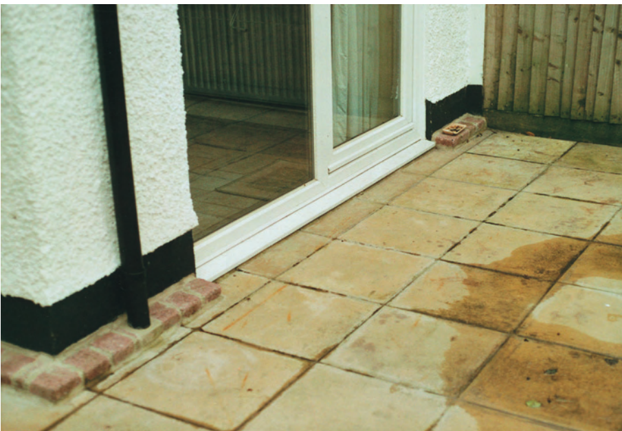
Fig. 4.13 The paving is too high. It should be lowered to at least 150 mm (2 brick courses) below the damp-proof course or internal floor level whichever is the lower, with a slope away from the wall.
