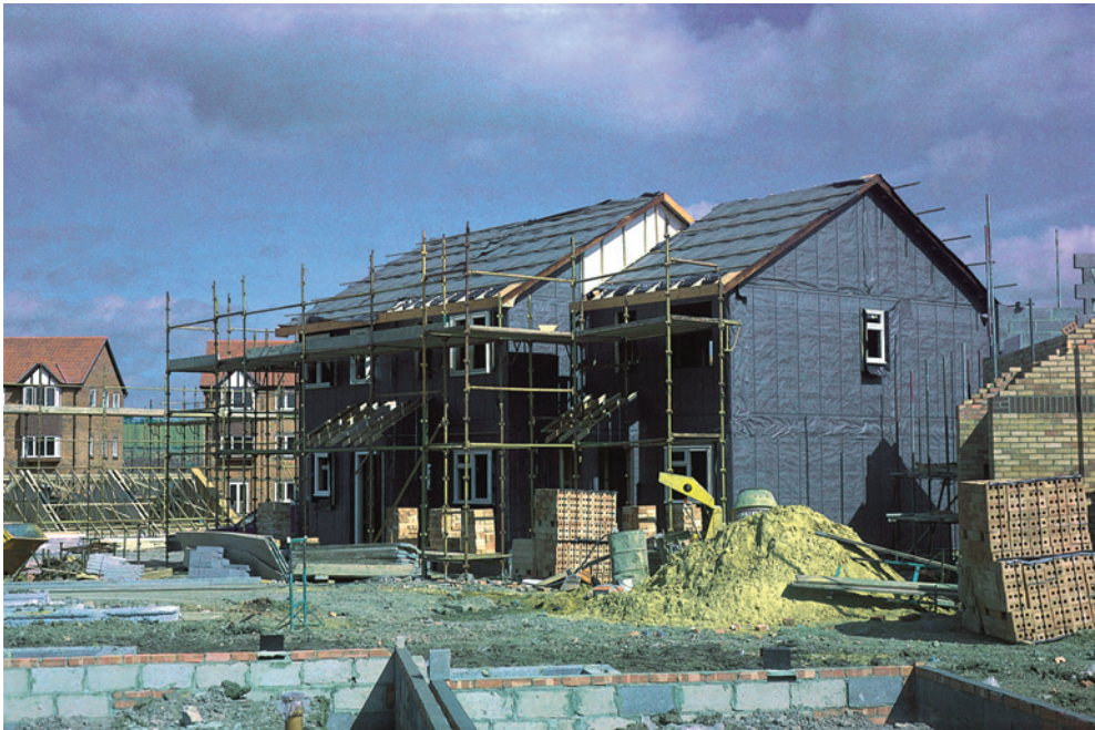
Fig. 7.1 Timber frame house under construction in an estate. Note the breather membrane over the timber frame inner skin to the prefabricated timber frame construction.
