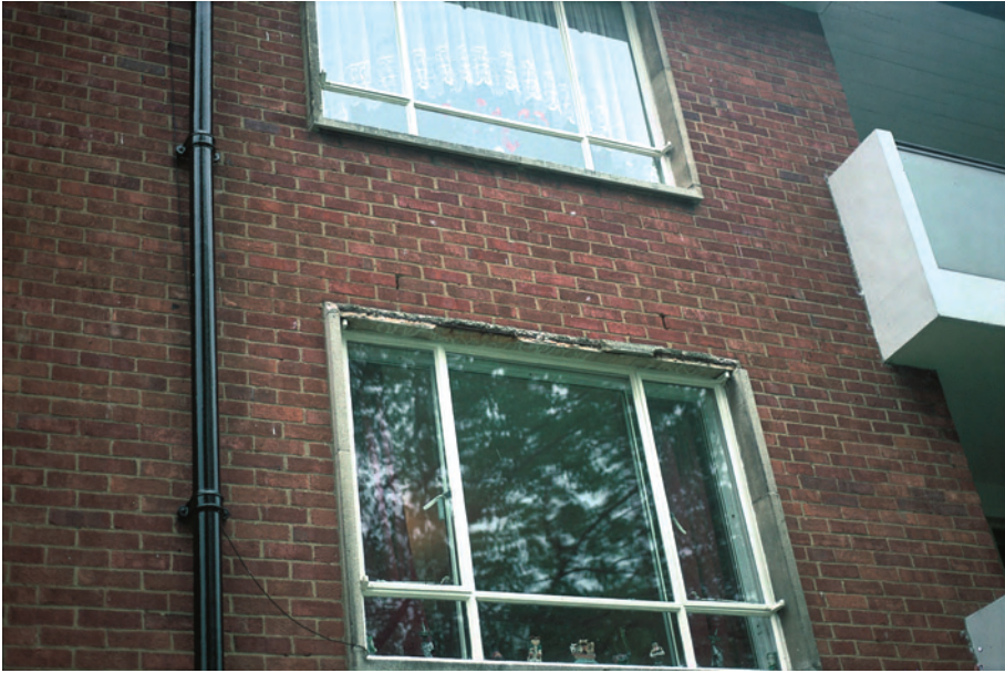
Fig. 4.6 Inadequate cover for steel reinforcement in concrete lintel. Rust can take up to seven times the space of the steel it replaces causing bursting to the concrete surface.
