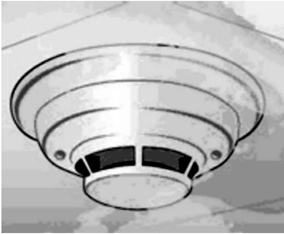
**FIGURE 9.35** Ceiling-mounted smoke detector. (Drawing courtesy of Scott Easton.)
