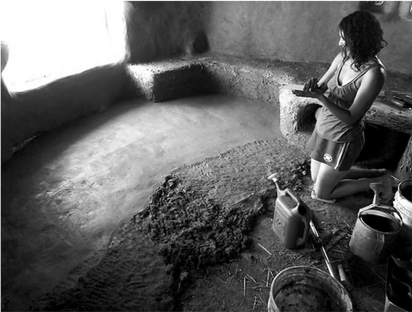
**FIGURE 6.4** Method for installing an earth floor. (Source: Brian “Ziggy” Liloia, “Building My Cob House” blog.)
