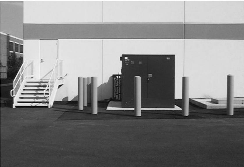
**FIGURE 9.24** Outdoor transformer protected by bollards.
