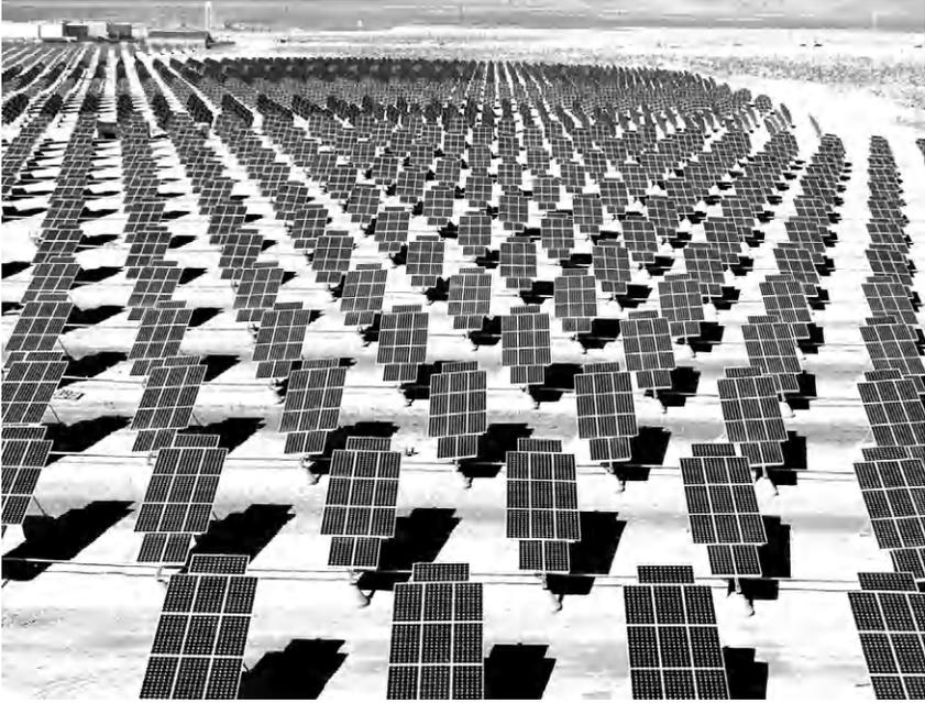
**FIGURE 9.28** This photo, taken by Airman 1st Class Nadine Barclay of the Nellis Solar Power Plant, shows the largest photovoltaic power plant in North America. The 70,000 solar panels sit on 140 acres of unused base land in Nevada, forming part of a solar PV array that will generate in excess of 25 million kilowatt-hours of electricity annually and supply more than 25% of the power the base uses. (Source: Wikimedia Commons; photo by Nadine Y. Barclay, October 2007)
