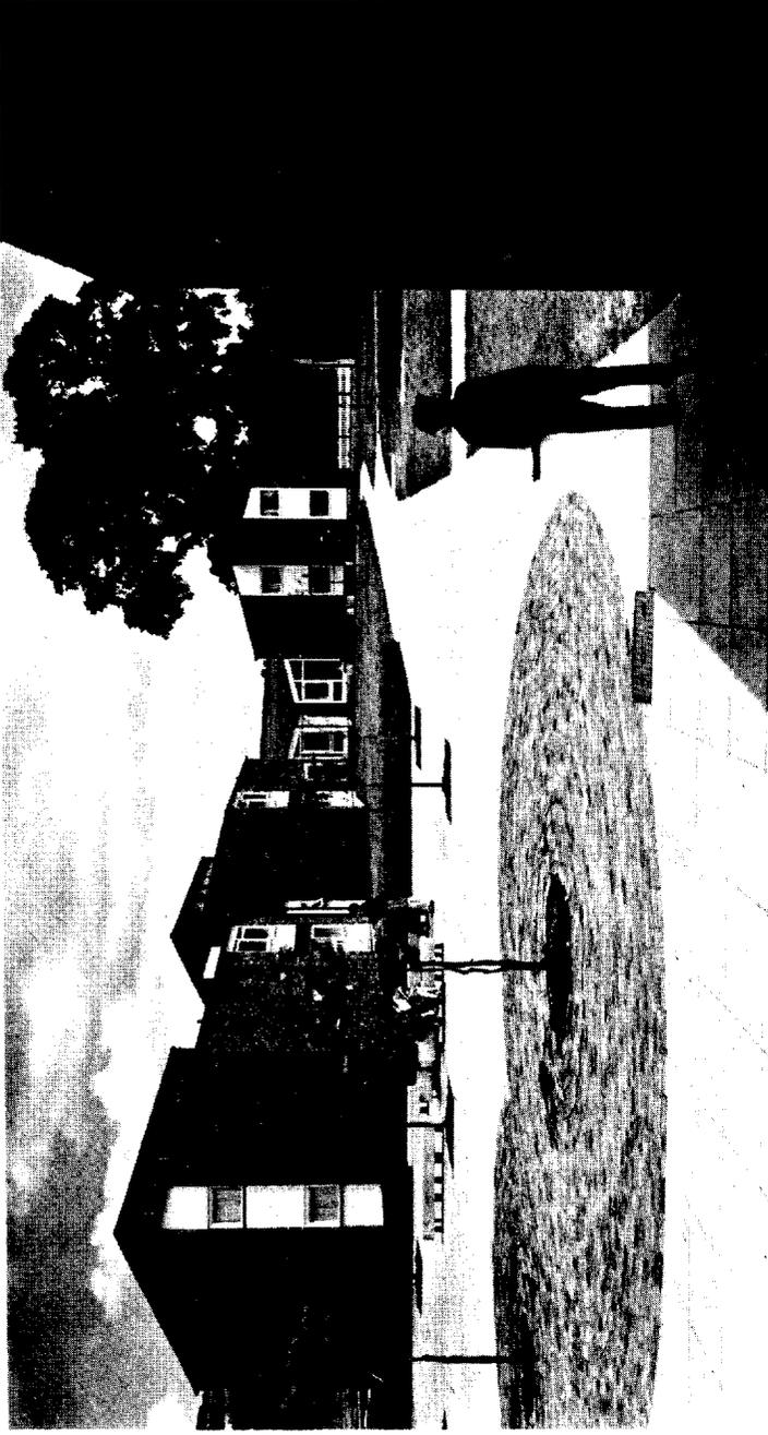
**2.1** Example of what can happen if site elements are not fully related. The manhole cover relates to neither the paving slabs nor the brick pavings
