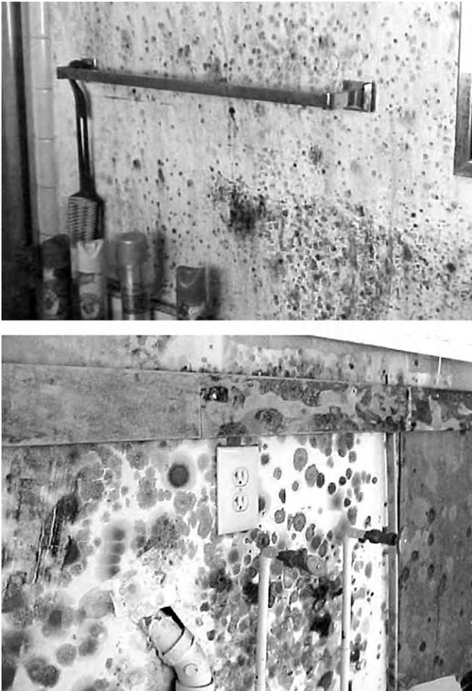
**FIGURE 16.1** Heavy mold infestation caused by water penetration left unattended. (Source: Servpro Industries, Inc.)
