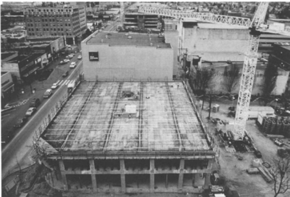
**Figure 1.6** Prestressed flat slab construction (*courtesy VSL International*).
