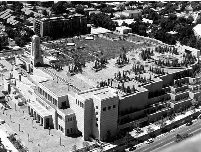
**FIGURE 6.6** Example of a 70,000-square-foot vegetated roof on the LDS Assembly Hall building, Salt Lake City. (Source: American Hydrotech, Inc.)
