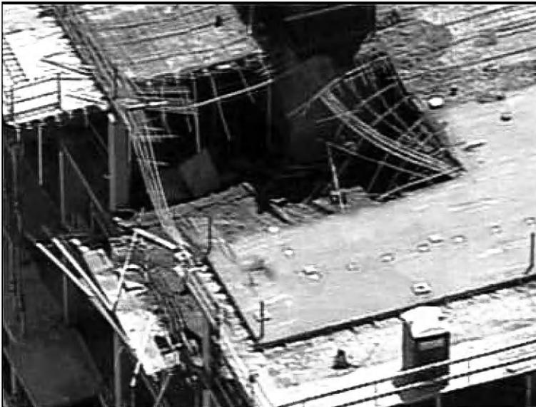
**FIGURE 16.2** Fourteen people were injured when a section of the roof of the “The Landmark,” a \$140 million high-rise building, collapsed onto the 13th and 12th floors as concrete was being poured for the building’s roof. (Source: CBS Broadcasting Inc.)
