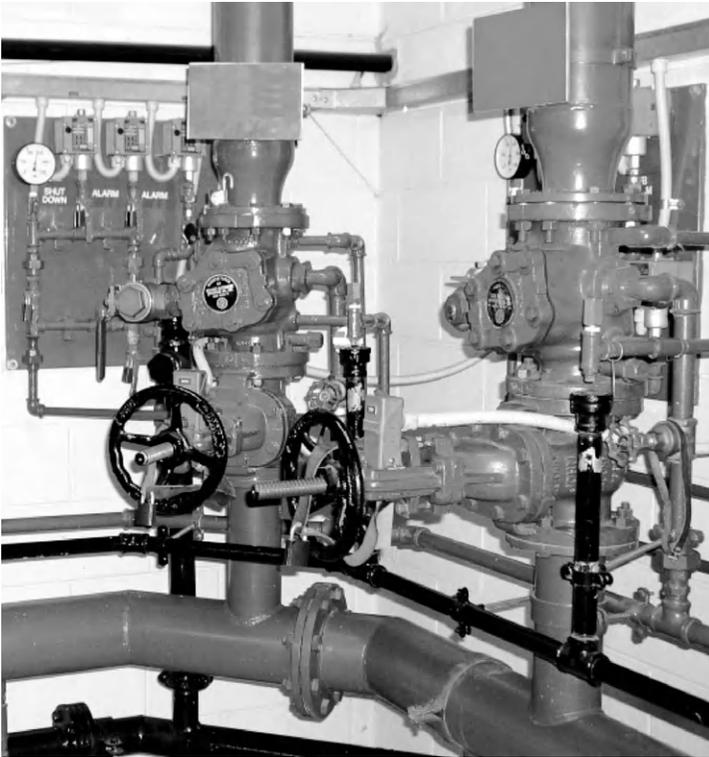
**FIGURE 9.30** Fire sprinkler control valve assembly including pressure switches and valve monitors. (Source: Wikipedia.)
