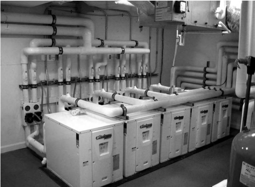
**FIGURE 9.11** Residential geothermal heat pump system. (Source: *Climate Heating and Cooling*.)
