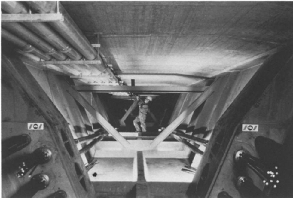
**Figure 1.5** Externally prestressed bridge deck (*courtesy VSL International*).
