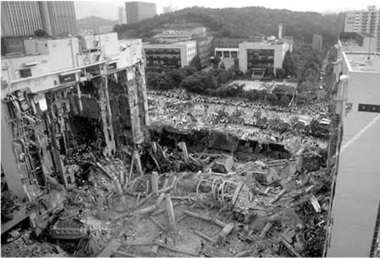
**FIGURE 16.4** There were more than 1500 people in this luxury department store in Seoul, South Korea, when a section of the five-story building collapsed in June 1995. More than 500 people were killed as a result. The building was constructed using steel-reinforced concrete pillars. The collapse was blamed on faulty construction.
