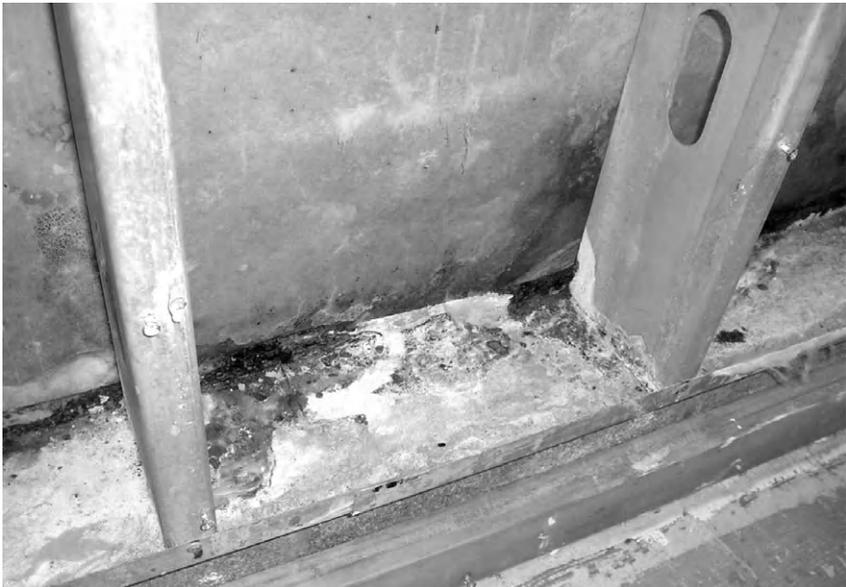
FIGURE 9.5 Effects of water penetration contributing to mold growth.
