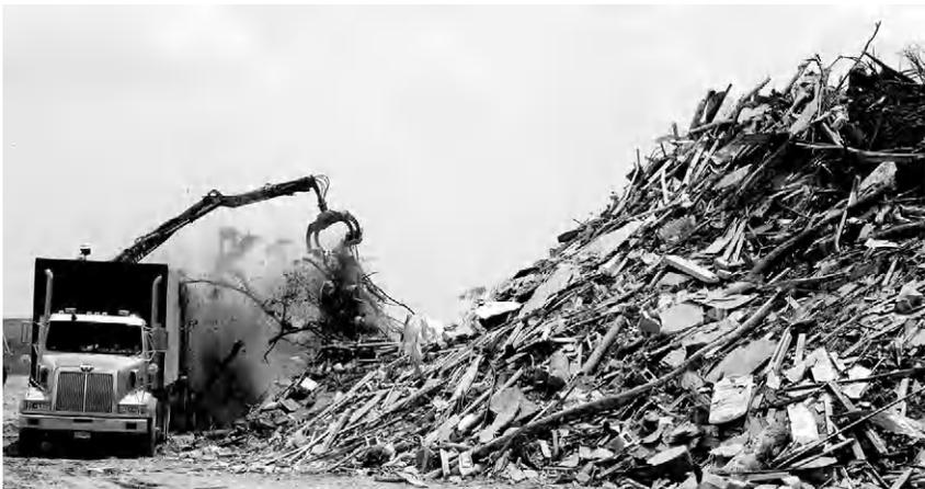
**FIGURE 6.11** Truck from DRC Emergency Services unloading construction and demolition debris at Birmingham’s New Georgia Landfill, which is being used for brush, tree, construction, and demolition debris from the April 27, 2011, tornadoes. (Source: Birmingham News/Joe Songer.)
