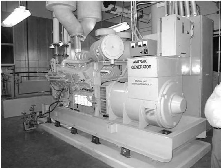
**FIGURE 9.23** Amtrak generator for emergency backup power.
