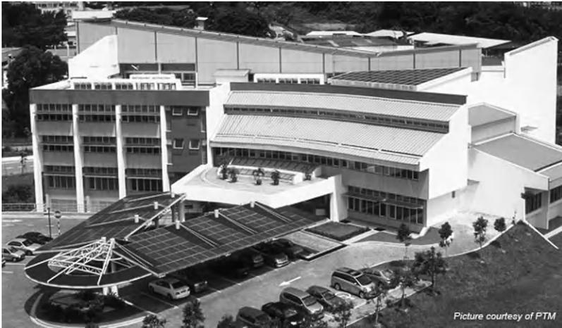
**FIGURE 2.10** PTM Green Energy Office (GEO) Building is Malaysia's first GBI-certified building and is designed as an administration-cum-research office for Pusat Tenaga Malaysia (Malaysia Energy Centre). The GEO building is built on five acres in Seksyen 9, Bandar Baru Bangi, Selangor, Malaysia. It is among the first Malaysian government office buildings with a design based on green concepts and is environmentally friendly. (Courtesy of PTM-GreenBuildingIndex.)
