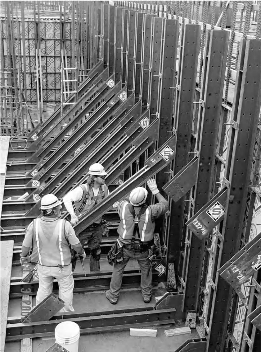
**FIGURE 6.10** Workers setting concrete formwork for the walls of a high-level waste facility pit. (Source: Bechtel Corporation.)
