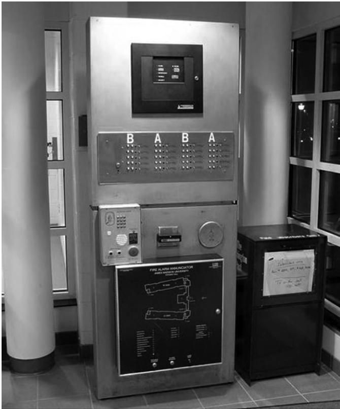
**FIGURE 9.37** Siemens MXL fire alarm control panel (*top*) and graphic annunciator (*bottom*). These devices were installed in Potomac Hall at James Madison University. (*Photograph by Ben Schumin, 2003, Wikipedia.*)
