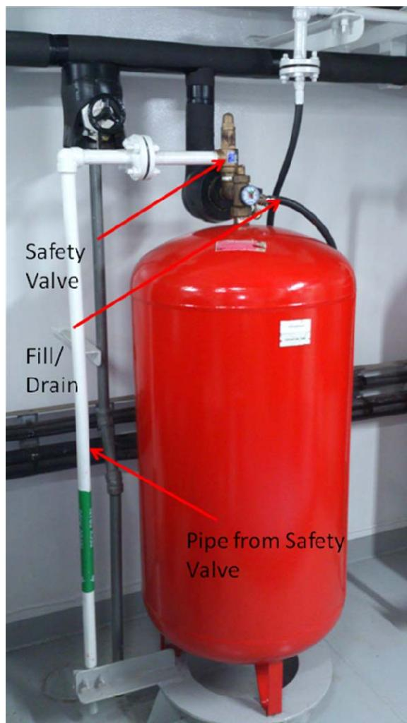
Fig.4.3. Expansion tank installation
