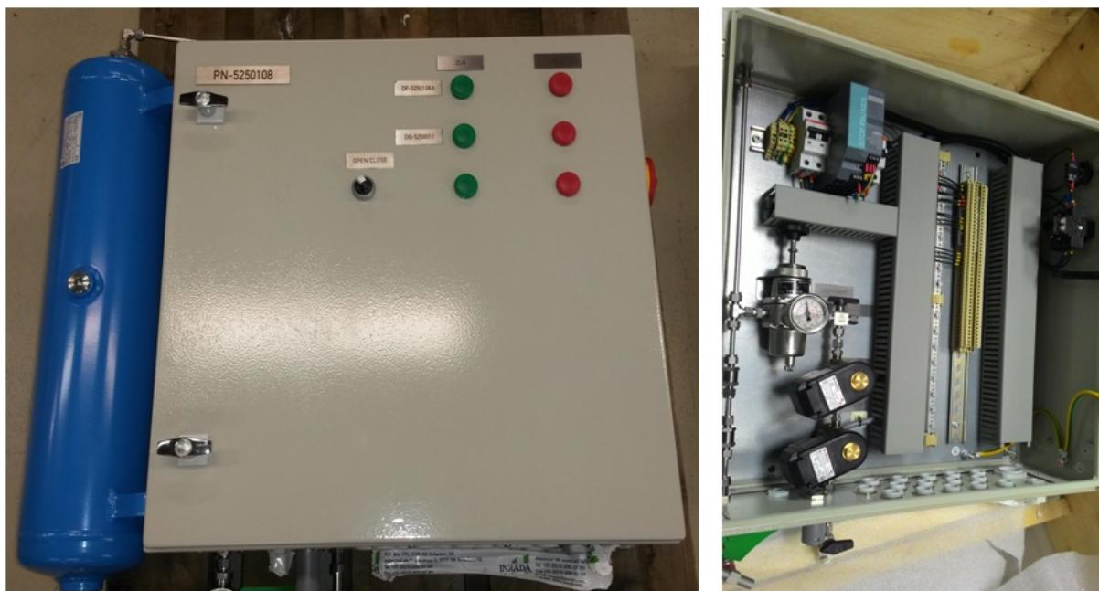
Fig. 9.21. Damper control panel
