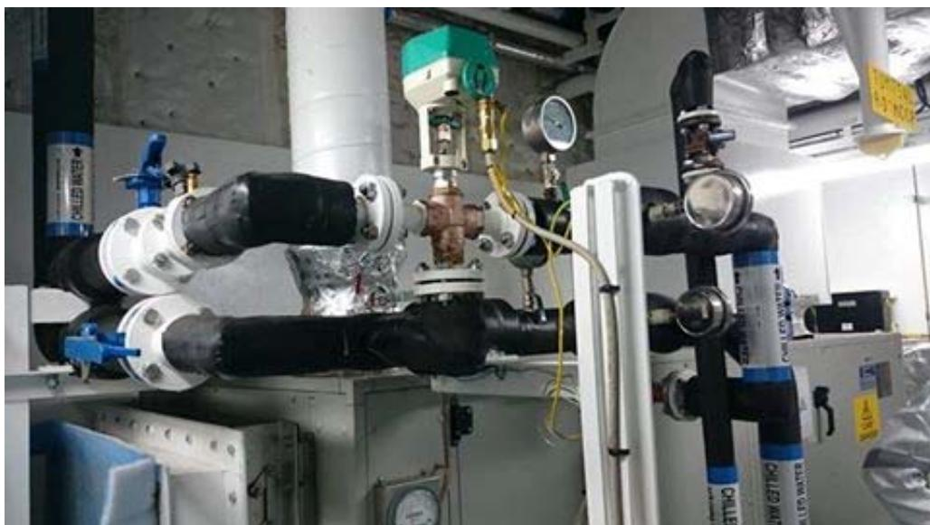
Fig 7.10. Chilled water circuit at AHU
