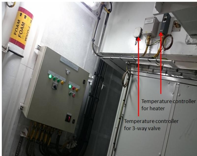
Fig 7.19. Duct mount temperatures and HVAC Control Panel
