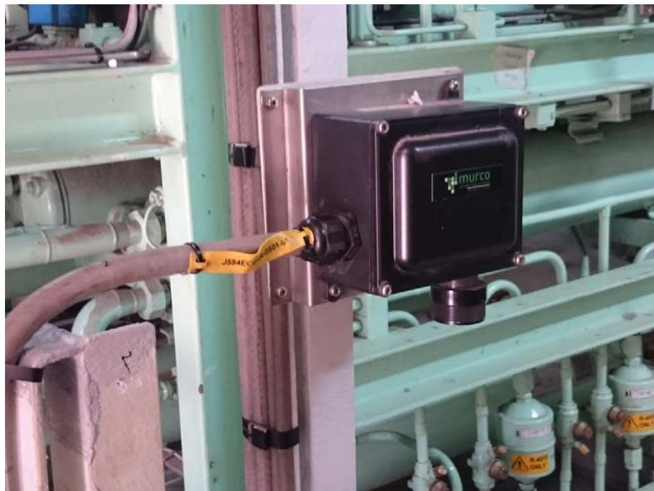
Fig.10.1. Gas Sensor at the nearby condensing unit
