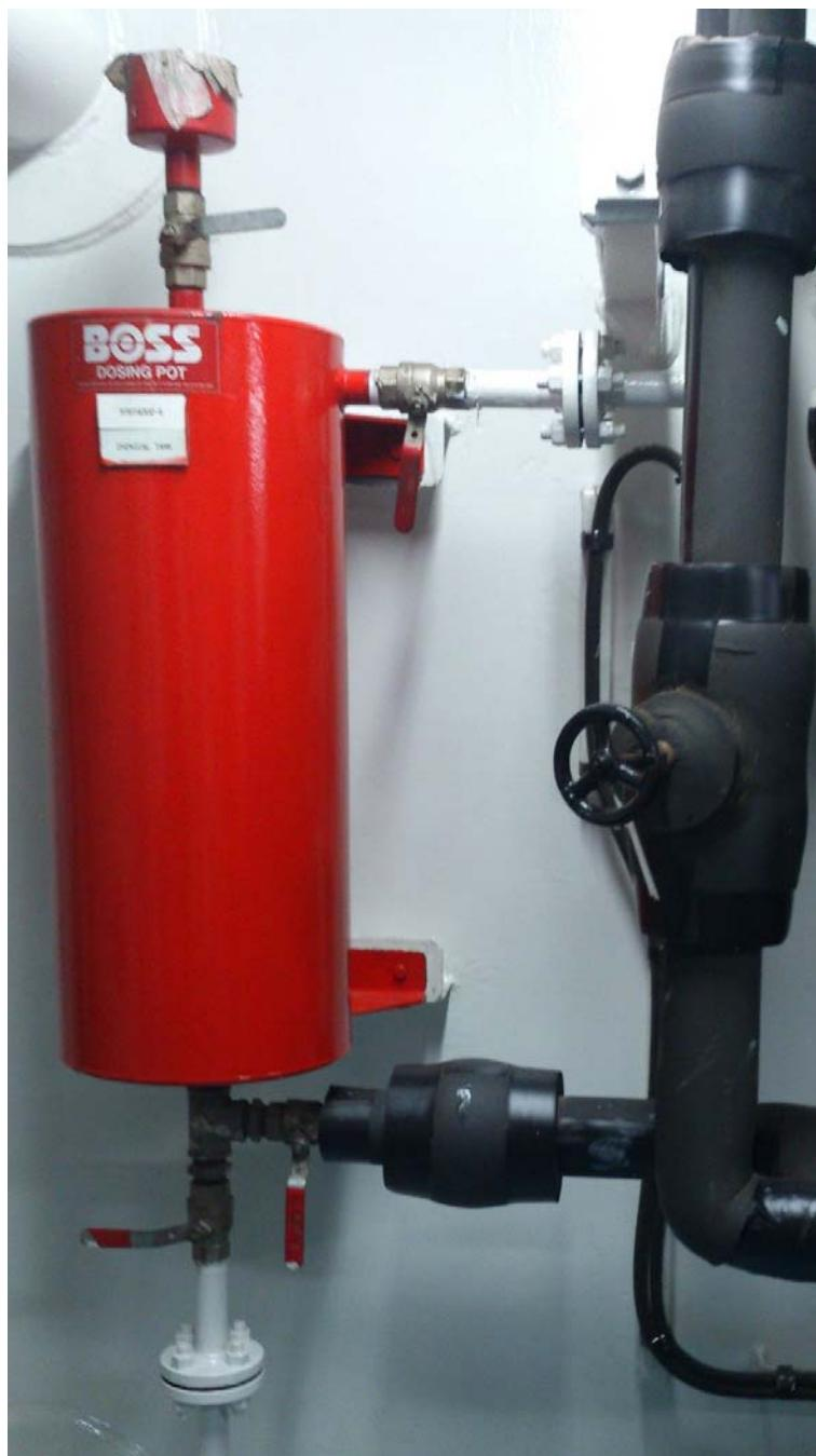
Fig.5.3. 50 Lit Chemical dosing pot installation
