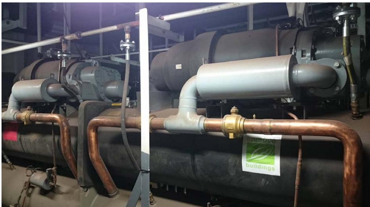
Fig. 2.5. Carier twin screw chiller (1300 kW cooling capacity)
