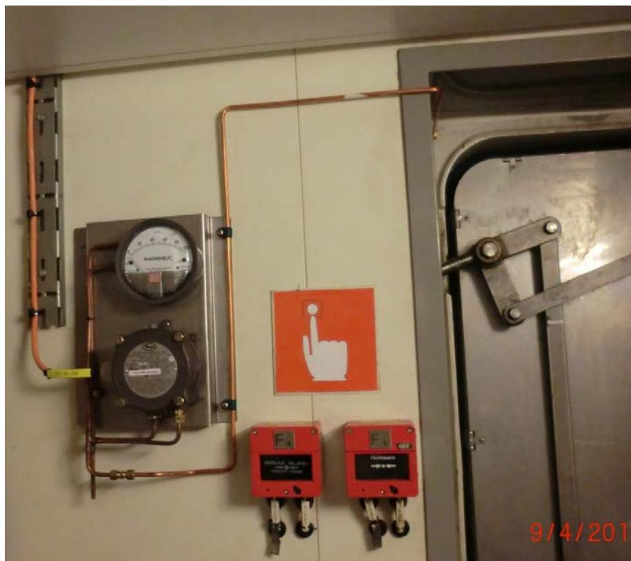
Fig.11.2. Differential pressure monitoring system at wheelhouse
