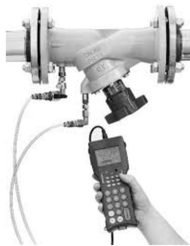
Fig 7.1 Balancing Valve
