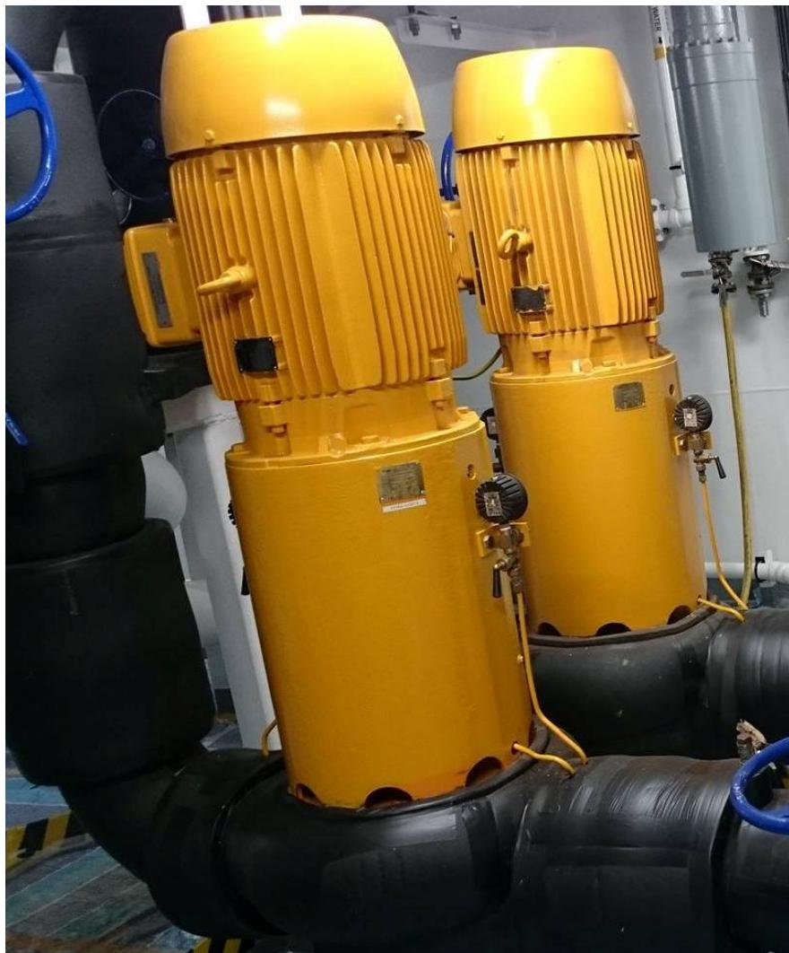
Fig. 3.3. Vertical in-line centrifugal pump
