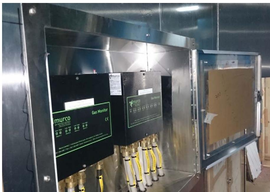
Fig.10.2. Gas controller for 4 and 6 sensors
