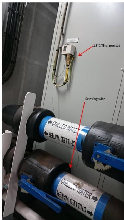
Fig 7.20. 18°C thermostat for chilled water temperature
