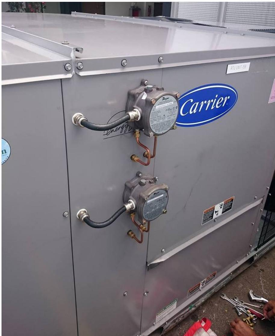
Fig.11.3. Differential pressure switch on Carrier package unit
