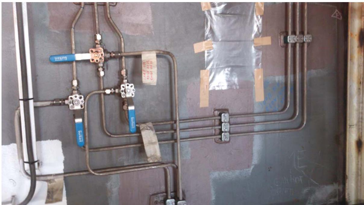
Fig. 9.18. 3-way ball valve and pneumatic tubing
