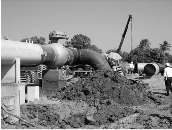
FIGURE 2-8-3 Typical construction site – Note the main line valves welded to the pipeline.
