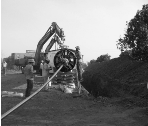
FIGURE 2-3-2b Mechanized welding of 48 inch diameter pipe.
