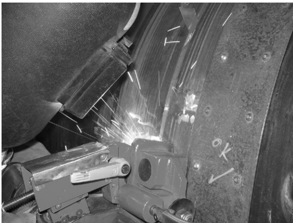
FIGURE 2-3-2a Mechanized welding being performed.
