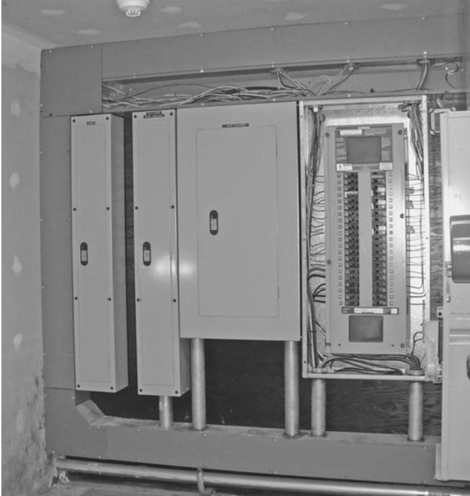
FIGURE 9.148 Metal wireways can often avoid derating penalties for mutual conductor heating.
