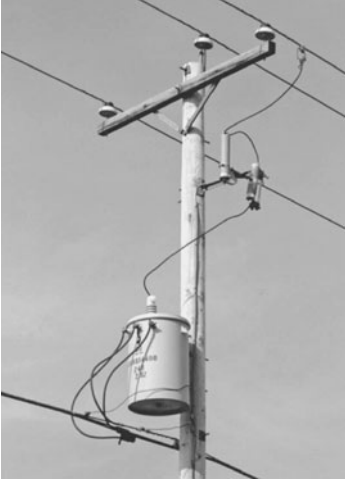
FIGURE 5.80 Pole-mounted 30-kVA distribution transformer protected with conventional surge arrester and separate current-limiting fuse. [Cooper Power Systems]
