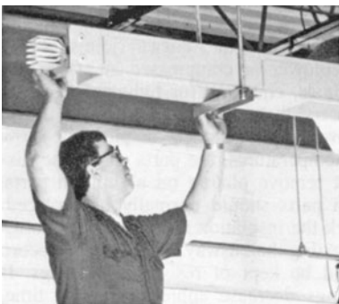
FIGURE 9.173 Installing busway on hangers.
