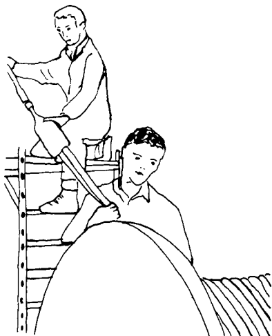
FIGURE 2.52 When bare steel basket grips and similar pull-line-to-cable devices must be used, cover them with plastic tape or rubberlike shields.
