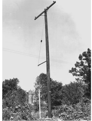
FIGURE 8.92 A vertical or "sidewalk" guy completely installed.
