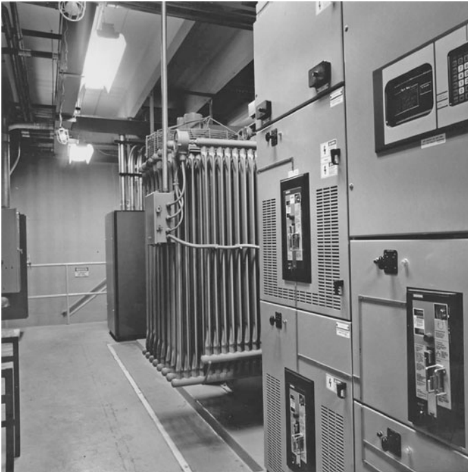
FIGURE 5.11 Liquid filled transformer utilizing silicone liquid listed by UL as a dielectric medium and less flammable per 450.23 of the NEC. [Dow Corning]
