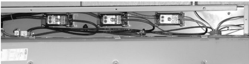
FIGURE 9.147 Length of wireway with power distribution blocks, each with a clear plastic cover over the uninsulated live parts.
