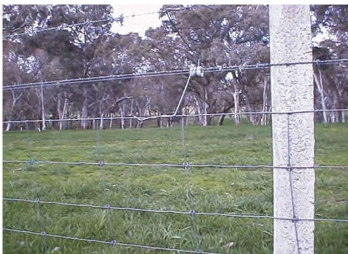
Figure1. Ringlock electric fence. Photo courtesy of A Cole
