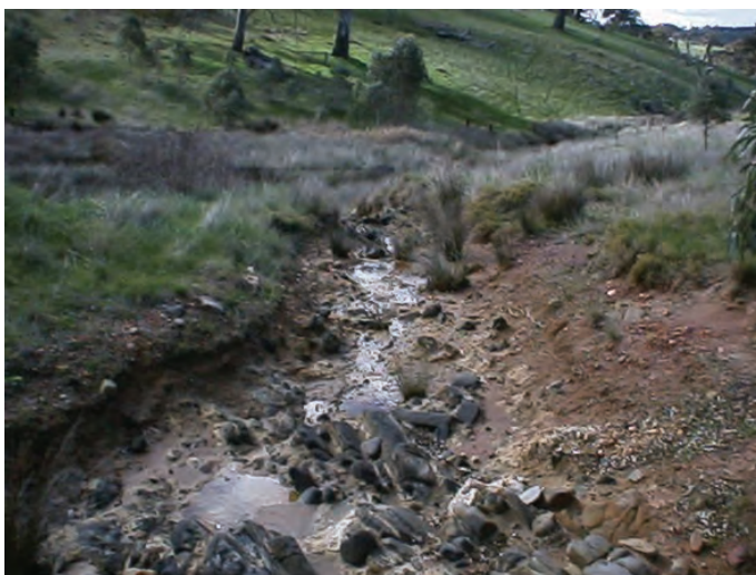
Figure 14. A correctly constructed spillway Photo courtesy A Cole
