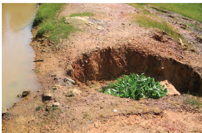
Figure 13. Seepage through the dam wall creates erosion Photo courtesy A Cole
