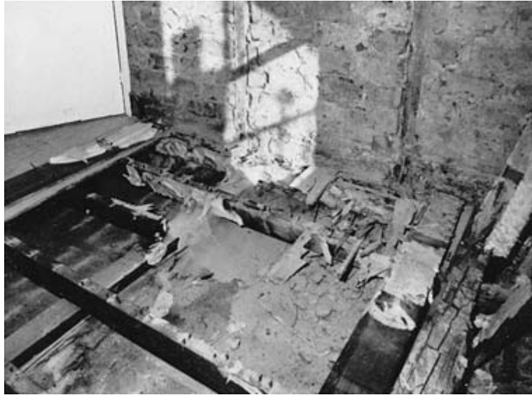
Figure 9.1 Dry rot spore dust in floor joists and partition (courtesy of SGB Group Publicity).
