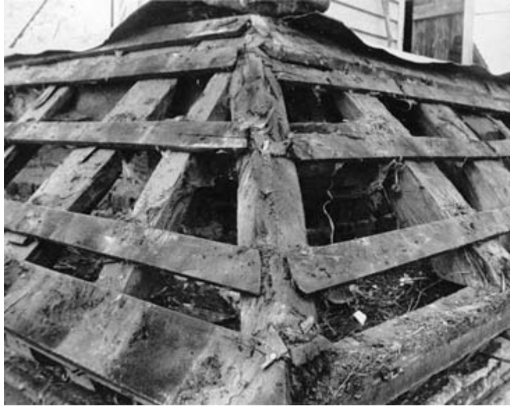
Figure 10.11 Timber roof structure after worn stone slates have been removed.
