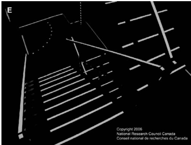
Figure 10.4 Photoluminescent material can help people see their way in evacuation routes that are without power or filled with smoke (photo courtesy of Dr Guylene Proulx, reproduced by permission of the National Research Council Canada).
