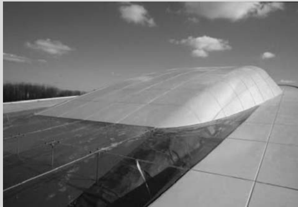
Figure E.11 Roof panels created with the Exploform technique after installation.
