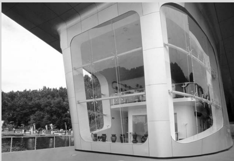
Figure E.9 Cold-deformed glass panels in the south façade.
