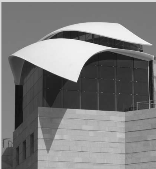
Figure E.17 The Library just after installment of the composite sandwich roofs in November 2005.
