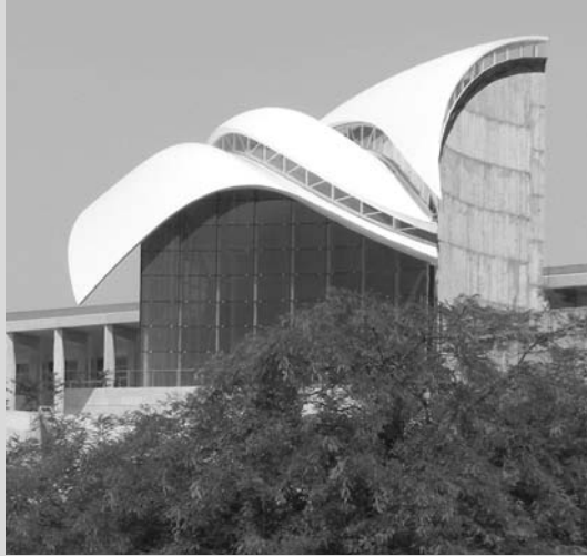
Figure E.18 The Great Hall just after installment of the composite sandwich roofs in November 2005.
