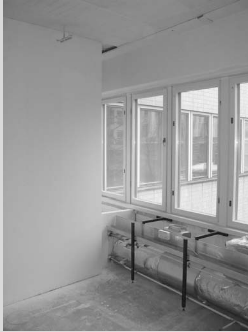
Figure C.3 The passage for the primary HPAC systems was found in between the exterior wall and the columns under the window sill. Construction phase.
