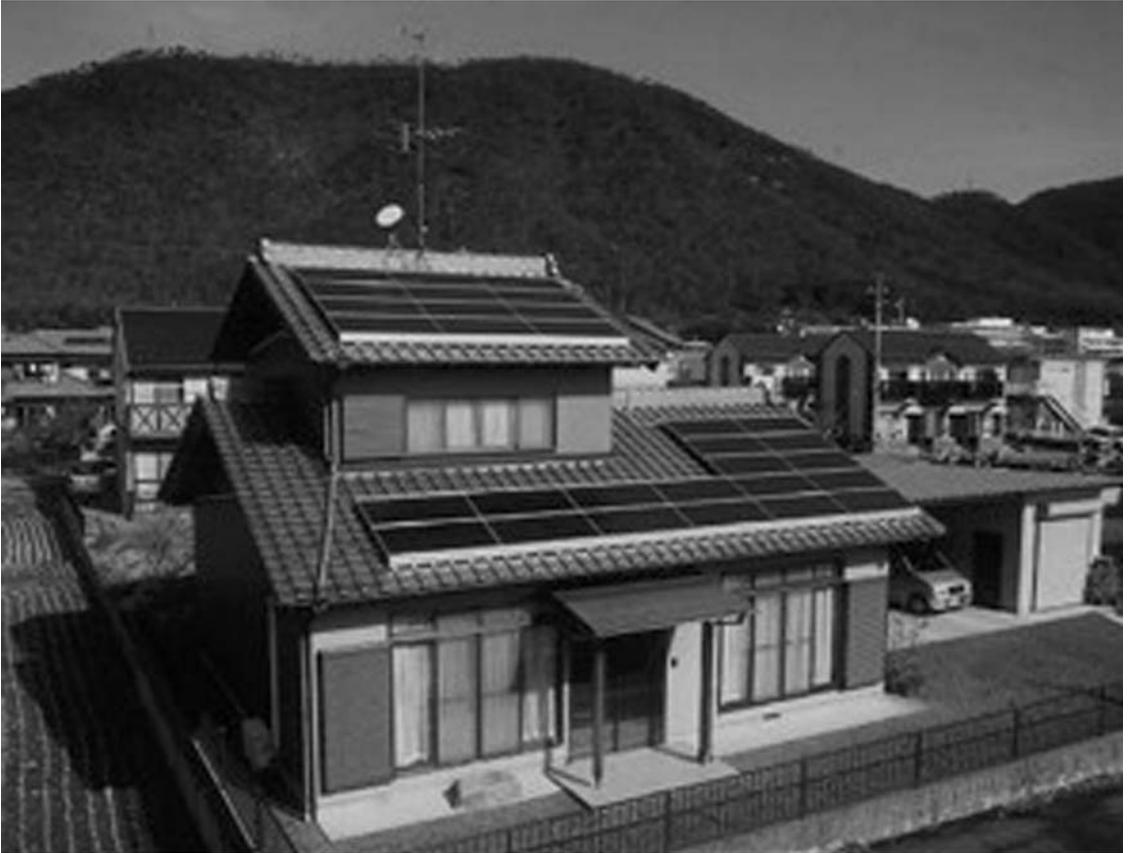
**Figure 6.17** Residential solar power installation (Courtesy of Evergreen Solar)
