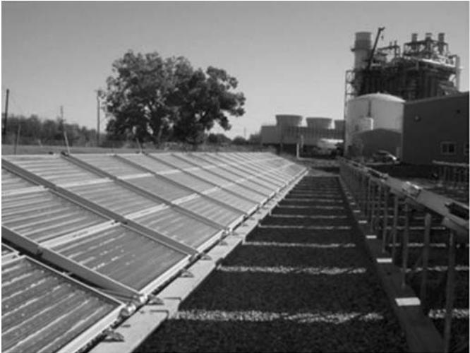
Figure 6.35 Solar cooling installation, industrial application (Courtesy of Solargenix)
