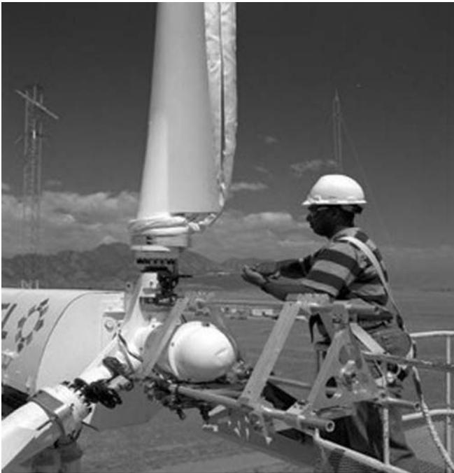
**Figure 4.18** Wind turbine installation (Courtesy of AWEMA)
