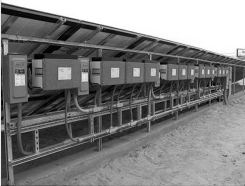
**Figure 6.8** Sunny Boy Inverter system for ground mount solar power installation (Courtesy AES)
