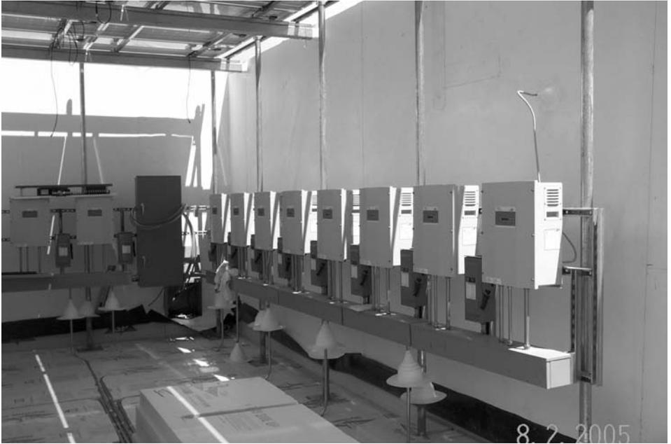
**Figure 2.27** Water and Life Museum Sunny Boy inverter assembly (Courtesy of Vector Delta Design Group, Inc.)
