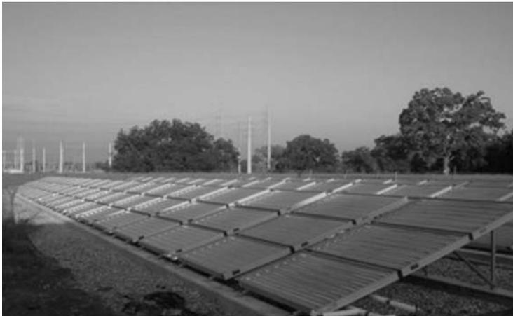
**Figure 4.5** Solar heat collector panel used in hybrid chillers (Courtesy of Solargenix)
