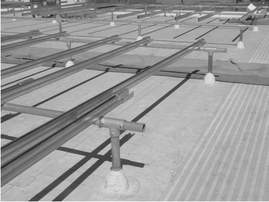
**Figure 2.23** Water and Life Museum photovoltaic panel support assemble (Courtesy of Lehrer Gangi Architects and engineered by Vector Delta Design Group, Inc.)
