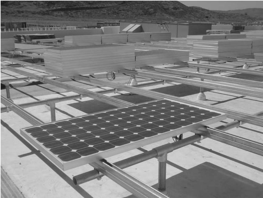
**Figure 2.24** Water and Life Museum photovoltaic panel support assembly (Courtesy of Vector Delta Design Group, Inc.)
