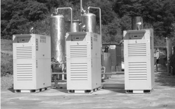
**Figure 4.44** Microturbine installation (Courtesy of Capstone Microturbine)
