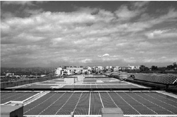
**Figure 6.15** Roof mount commercial solar power installation (Courtesy of PowerLight Corporation)
