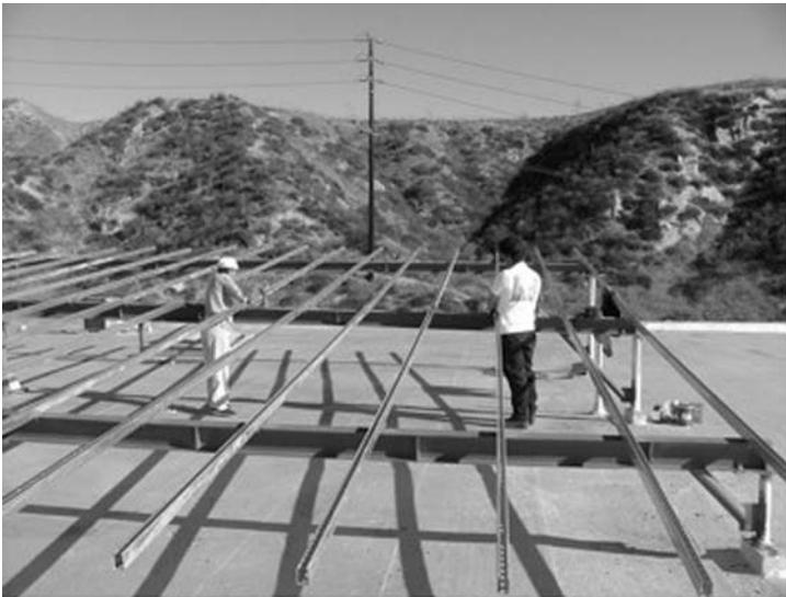
**Figure 6.27** Roof mount solar power support system (Courtesy of California Green Design)
