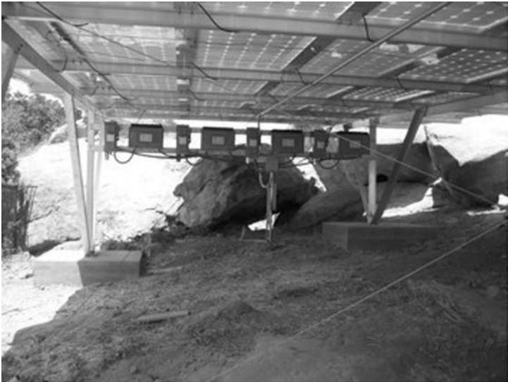
**Figure 6.24** Inverter system for ground mount solar power installation (Courtesy of California Green Design)
