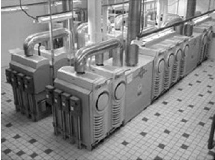
Figure 4.45 Microturbine indoor installation (Courtesy of Capstone Microturbine)
