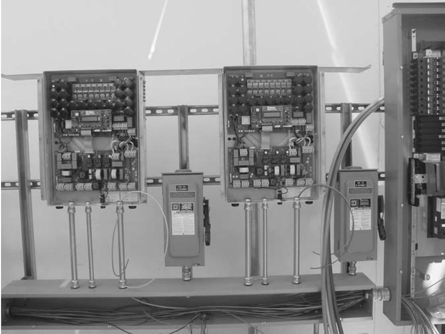
**Figure 2.28** Water and Life Museum inverter electronics (Courtesy of Vector Delta Design Group, Inc.)
