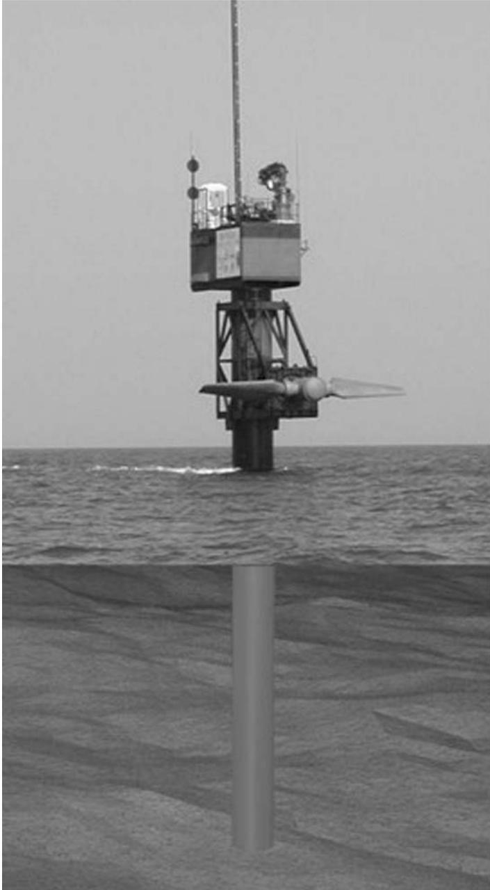
Figure 4.25 Marine current pile mounted turbine installation (Courtesy of MCT, UK)
