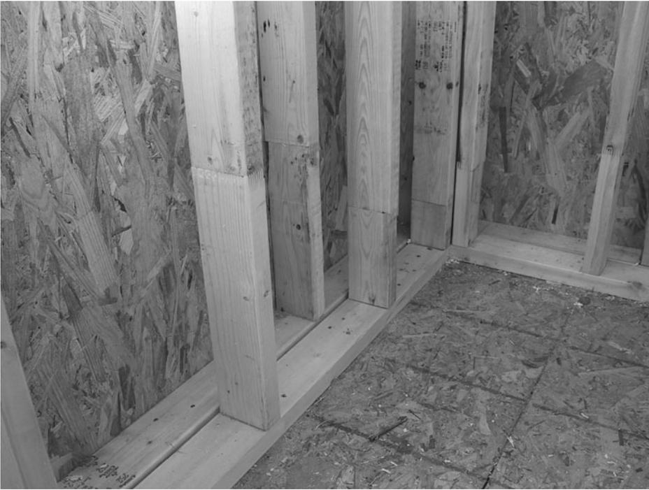
Staggered Stud Exterior Wall, Finger Joined Studs. *Dale Miller, Photographer.*
