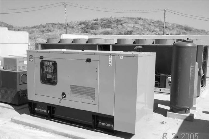
**Figure 2.29** Water and Life Museum emergency generator system (Courtesy of Vector Delta Design Group, Inc.)
