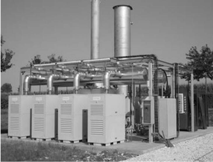
**Figure 4.47** Microturbine in landfill installation (Courtesy of Capstone Microturbine)
