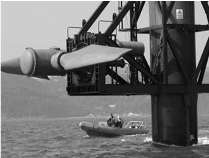
**Figure 4.24** Marine current pile mounted turbine installation (Courtesy of MCT, UK)
