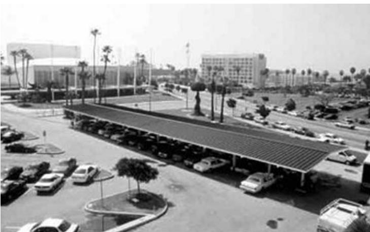
**Figure 6.13** Carport solar power installation (Courtesy of United Solar Ovonic Corporation, Santa Monica, California)
