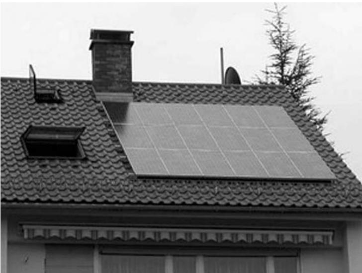
**Figure 6.18** Residential roof mount solar power installation (Courtesy of Evergreen Solar)
