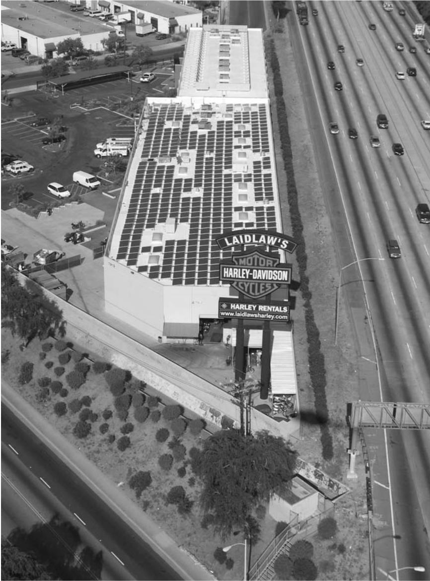
Figure 6.1 Roof mounted solar power installation (Courtesy of Solar Electrical Systems)
