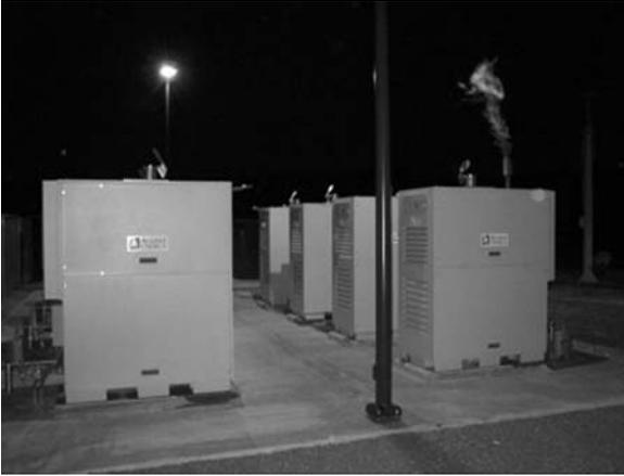
**Figure 6.31** Tandem microturbine installation (Courtesy of Capstone Micro Turbine)
