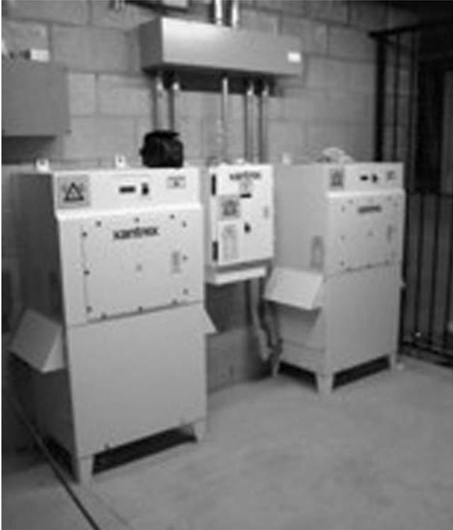
Figure 2.16 Inverter equipment for TCA A. Dickranian Armenian School's solar power cogeneration system diagram
