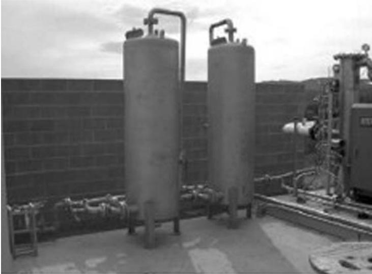
Figure 4.51 Gas filtration component installation (Courtesy of Capstone Microturbine)
