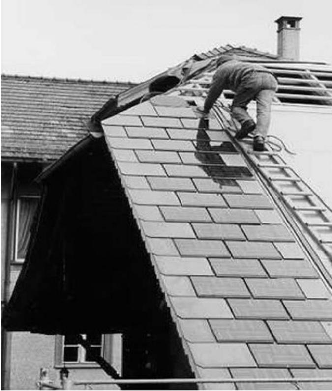
**Figure 2.9** Solar power slate system (Courtesy of Atlantis Energy)
