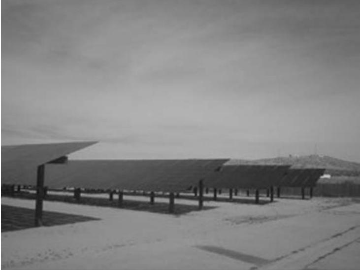
**Figure 6.2** Two hundred kilowatt ground mount solar power installation, Mojave Desert, California (Courtesy of Grant Electric)
