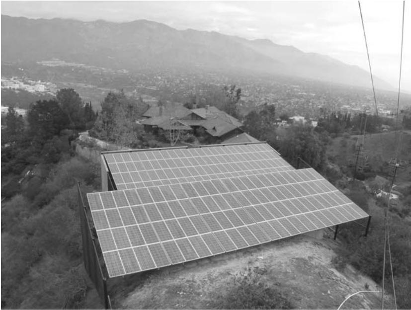
Figure 6.7 Ground mount solar power installation (Courtesy of Solar Electrical Systems)
