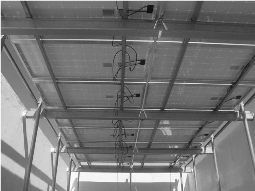
**Figure 2.26** Water and Life Museum photovoltaic panel module inter-wiring (Courtesy of Vector Delta Design Group, Inc.)
