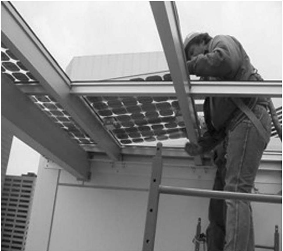
Figure 1.8 Example of a transparent solar power panel installation (Courtesy of Atlantis Energy)
