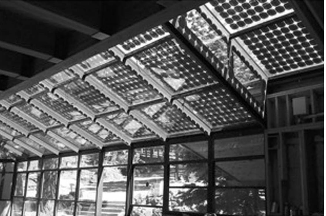
**Figure 1.9** Example of a transparent solar power panel application in a solarium (Courtesy of Atlantis Energy)
