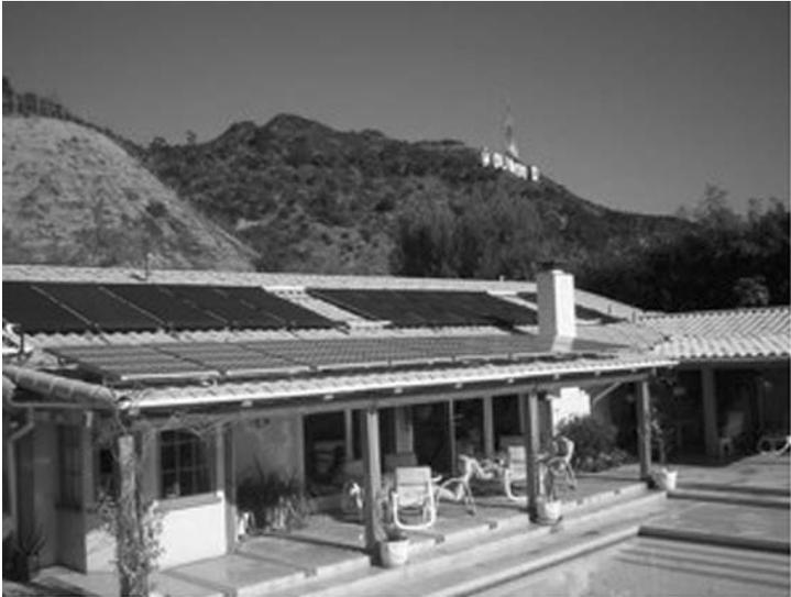
Figure 6.20 Four-kilowatt residential solar power installation, Hollywood, California (Courtesy of Grant Electric)
