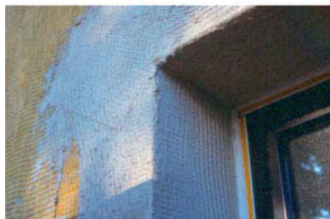
Fixing the stucco guides
