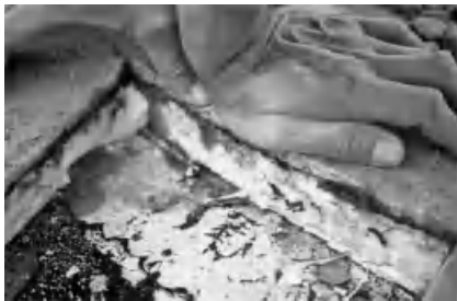
Figure 5.25. Heavy deck roof without vapour retarder above an indoor climate class 5 building, interstitial condensation in the PUR-insulation.
