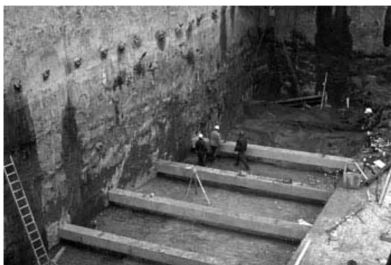
Figure 3.2. Deep walls nailed with grout anchors.
