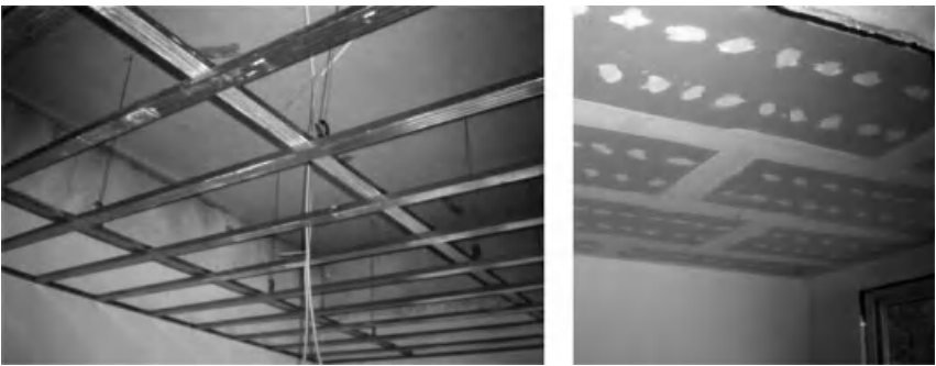
Figure 10.15. Closed gypsum board hung ceiling.
