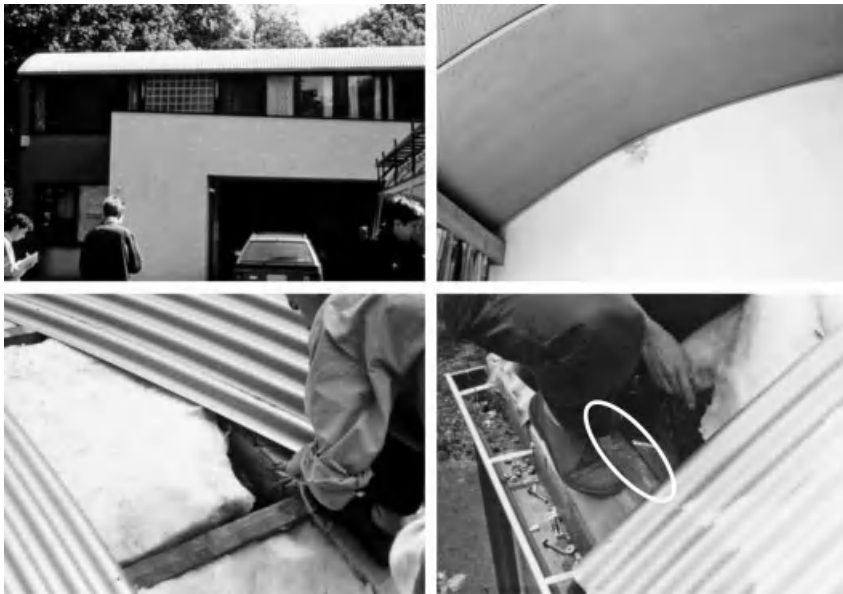
Figure 7.11. Dwelling. Up on the left a view of the metal roof, up on the right traces of moisture leakage, down on the left opening the roof, down on the right leaky vapour retarder along the perimeter.
