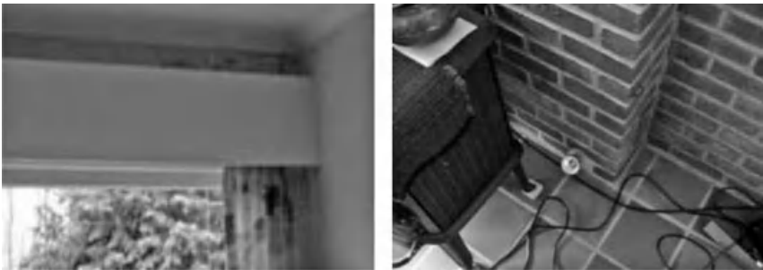
Figure 10.11. Mould on the lintel (on the left) caused by the ventilation pipe connecting the living room to the crawlspace (the pipe is where the lamp sits, see picture on the right).
