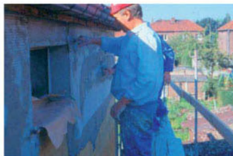
Embedding the glass fibre fabric
