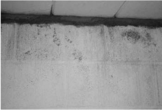
Figure 5.26. Outside protruding waterproof barrier below the floor at grade causes rain leakage into the basement.
