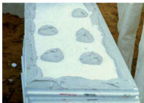
Pointwise mopping the bonding mortar
