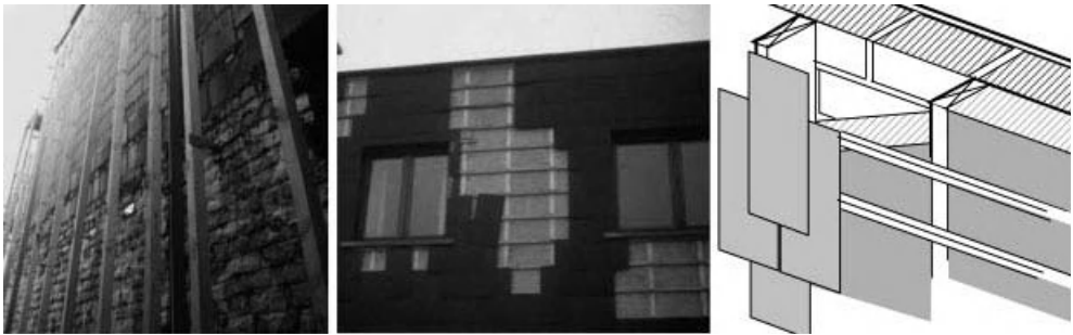
Figure 9.29. Massive walls with outside insulation: stud systems.
