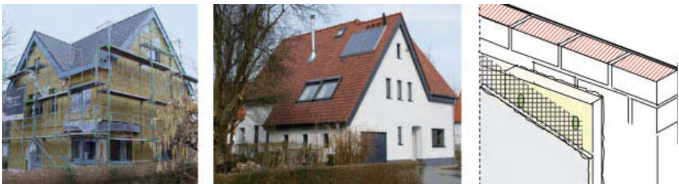
Figure 9.30. Massive walls with EIFS (on the left: while insulating, in the middle: once finished, on the right: a view of the assembly).
