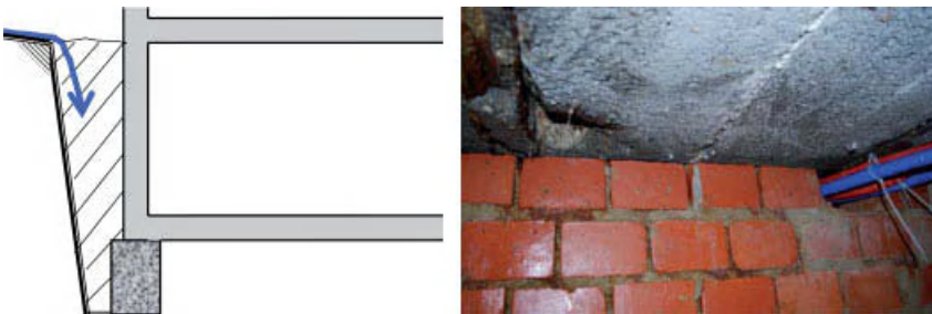
Figure 5.20. Seeping rainwater wedge around a basement.
