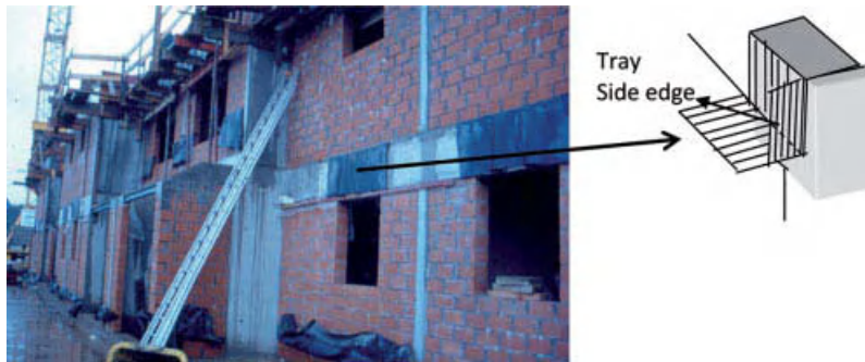
Figure 10.28. Cavity trays with side edges.
