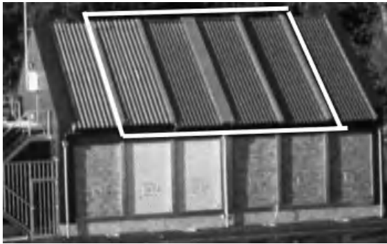
Figure 6.32. Test building used for testing the two times four saddle roofs (the four in the parallelogram).
