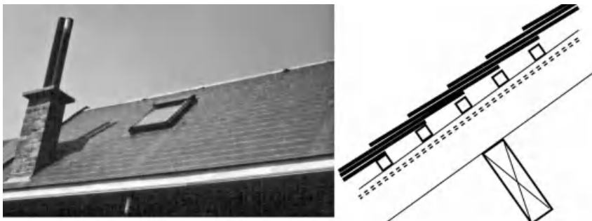
Figure 6.7. Slates, nailed in overlap on laths.
