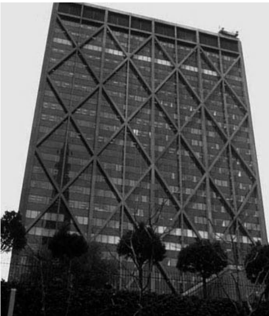
Figure 6.11. Trussed tube.
