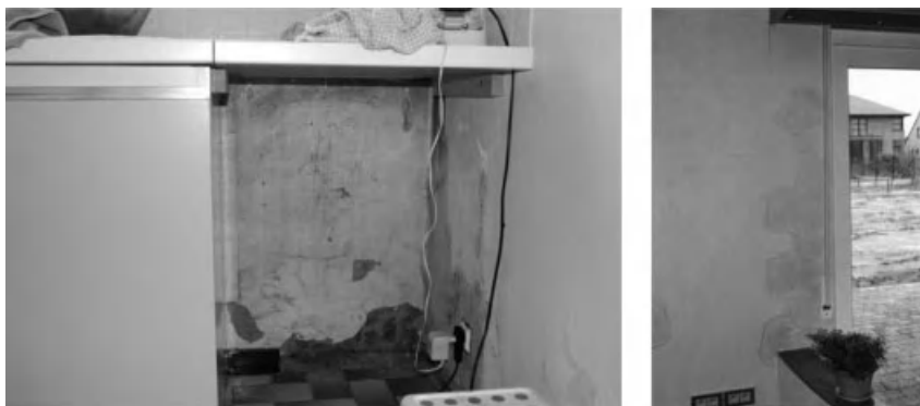
Figure 11.3. Rain penetration: on the left seen as rising damp in the inside, on the right giving a wet inside leaf along window bay.
