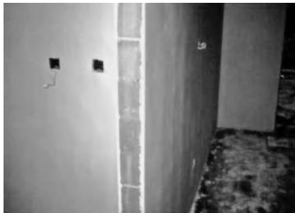
Figure 10.7. Partition wall, wet finish with gypsum plaster.
