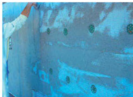
Additional fixing with synthetic nails
