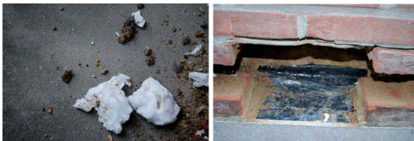
Figure 10.30. Post-fill with UF-foam (left), cavity tray with too low back flange as it looked after removing all mortar drops (right).
