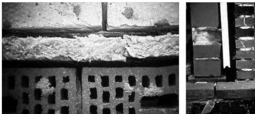
Figure 10.6. Insulation not linking up with the inside leaf (left), not touching the cavity tray (right).
