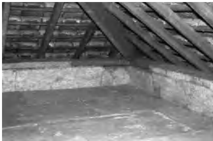
Figure 6.35. Insulation at ceiling level.
