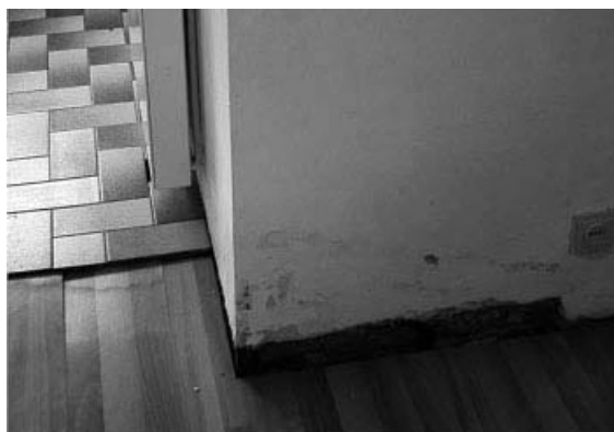
Figure 7.6. Floor in contact with bottom-wet partition wall.
