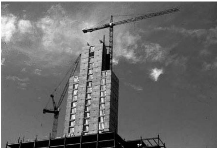
Figure 6.9. High rise with central core under construction.
