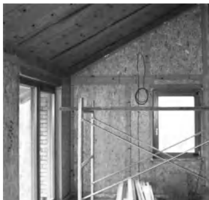
Figure 1.4. Taped OSB as air barrier.
