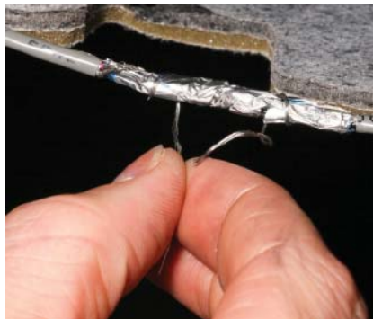
PS7-11 Wrap the drain wire around the outside of the Mylar tape.
