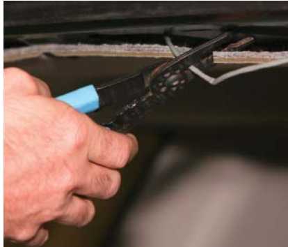
PS7-2 Locate and cut out the damaged section of wire.
