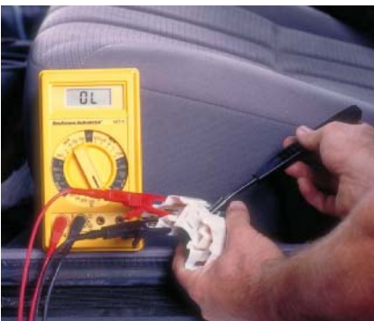
P16-16 When the dimmer switch is placed in the flash to pass position, there should be a closed circuit between terminals 196 and 12, and an open circuit between 196 and 13.
