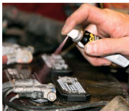
P9-17 Coat the battery terminals with corrosion-preventive spray. Perform a terminal test to assure tight connections.
