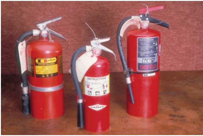
FIGURE 1-18 Know the location and types of fire extinguishers that are available in the shop.
