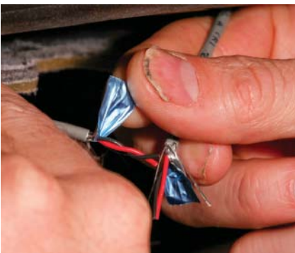
PS7-4 Unwrap the Mylar tape. Do not remove the tape from the cable.
