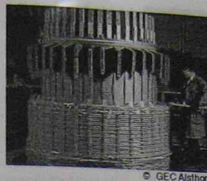
Figure 21: Interleaving discal coils showing internal transposition and external crossover
