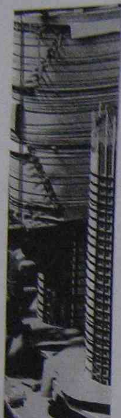
Figure 23: A three-phase distribution transformer in course of construction
