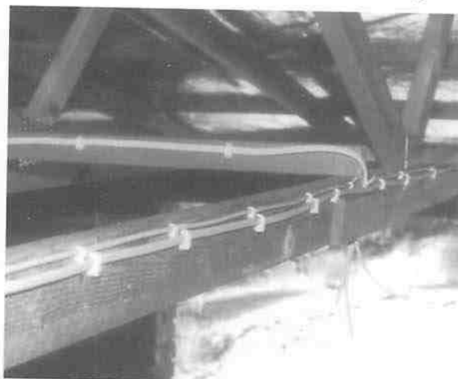
Fig. 8.6 Cables 'likely to be disturbed'
