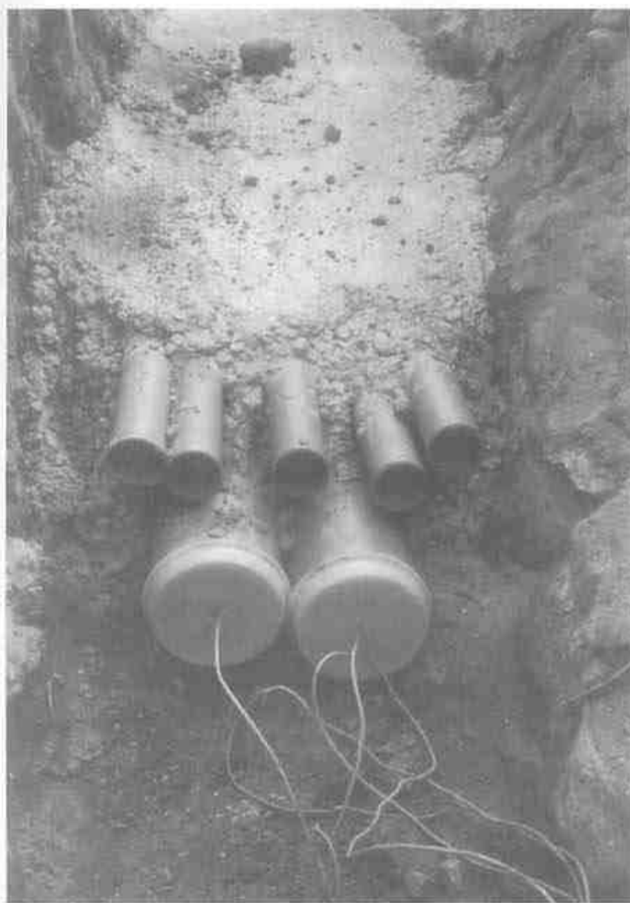
Fig. 7.23(a) Heavy-duty rigid unplasticised PVC conduits and ducts for an underground service
