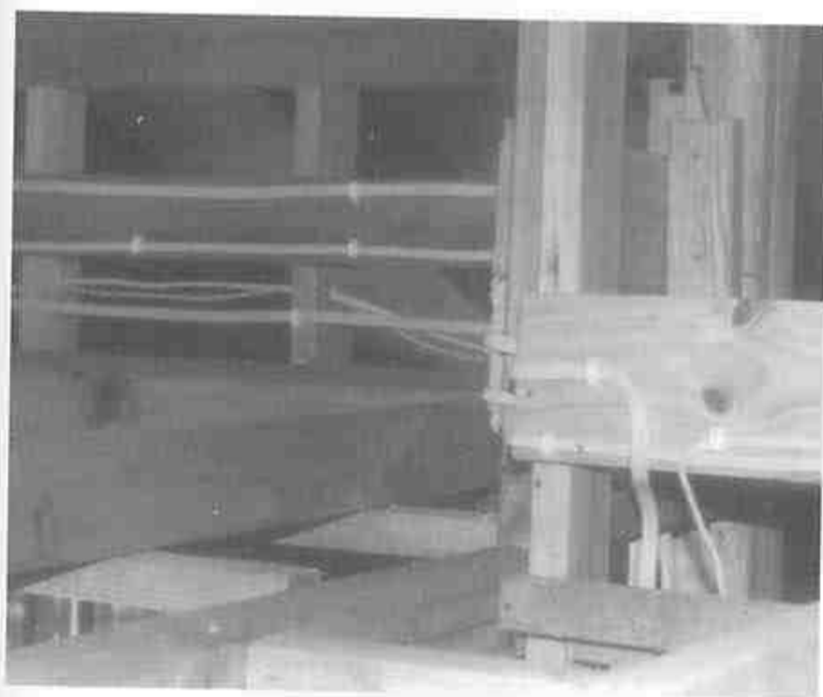
Fig. 8.5(b) Cables positioned clear of thermal insulation and to avoid the effects of mutual heating, with consequent derating of current-carrying capacity
