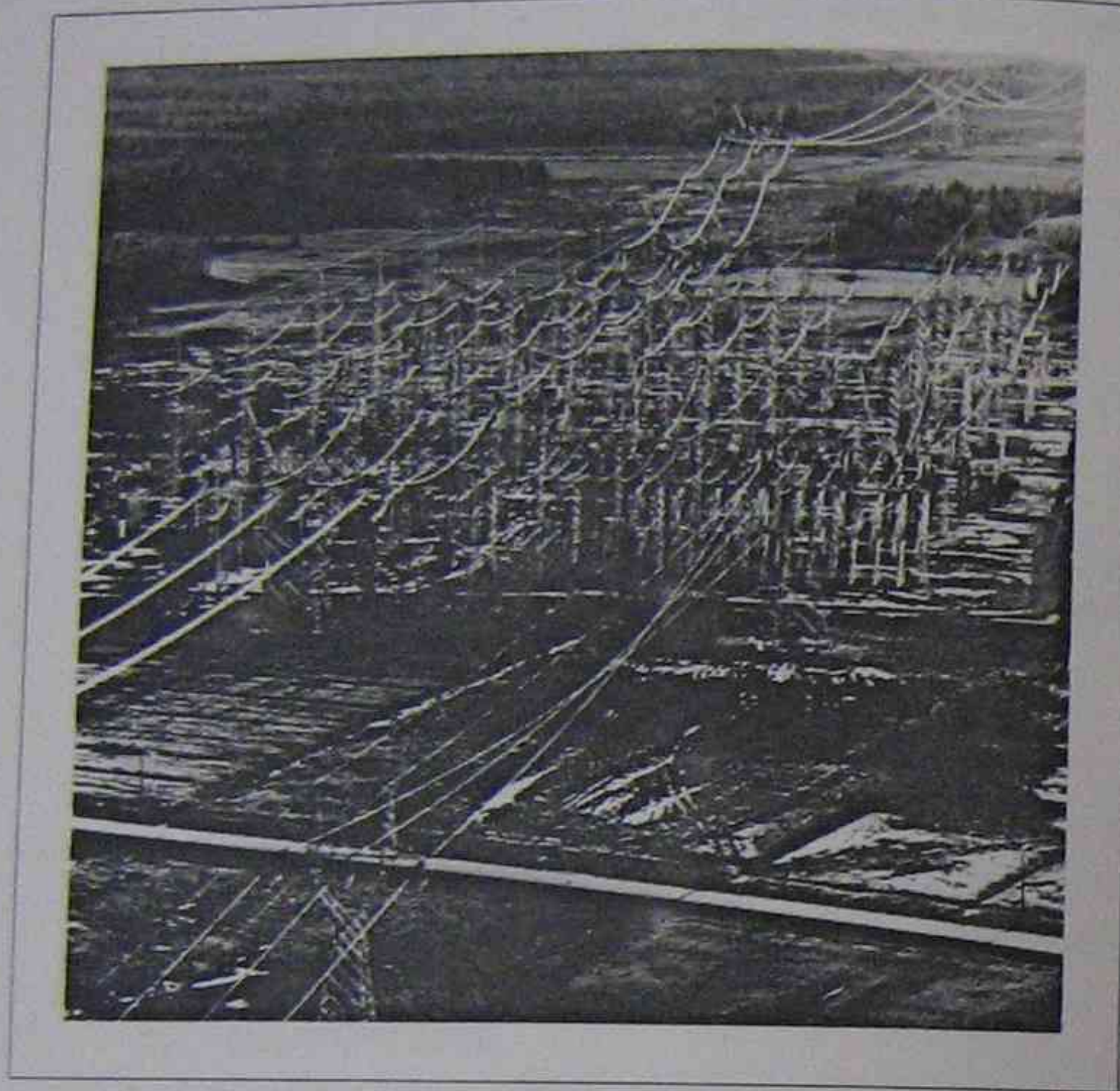
This large 735 kV switching station enables a spin-off of electric power and also serves as an intermediate voltage-regulating station.
