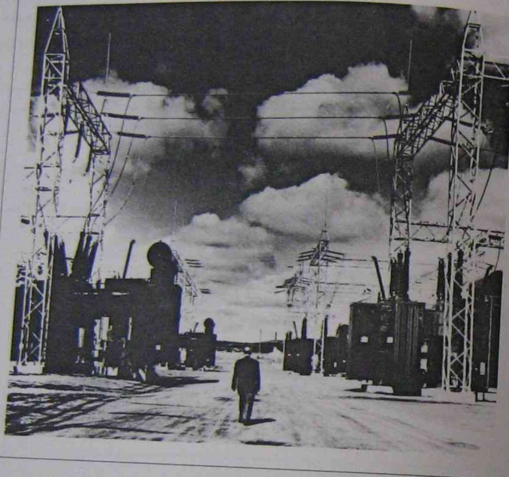
Three-phase, oil-filled, fan-cooled phase-shift transformer. Line-to-line voltage is 300 kV.
