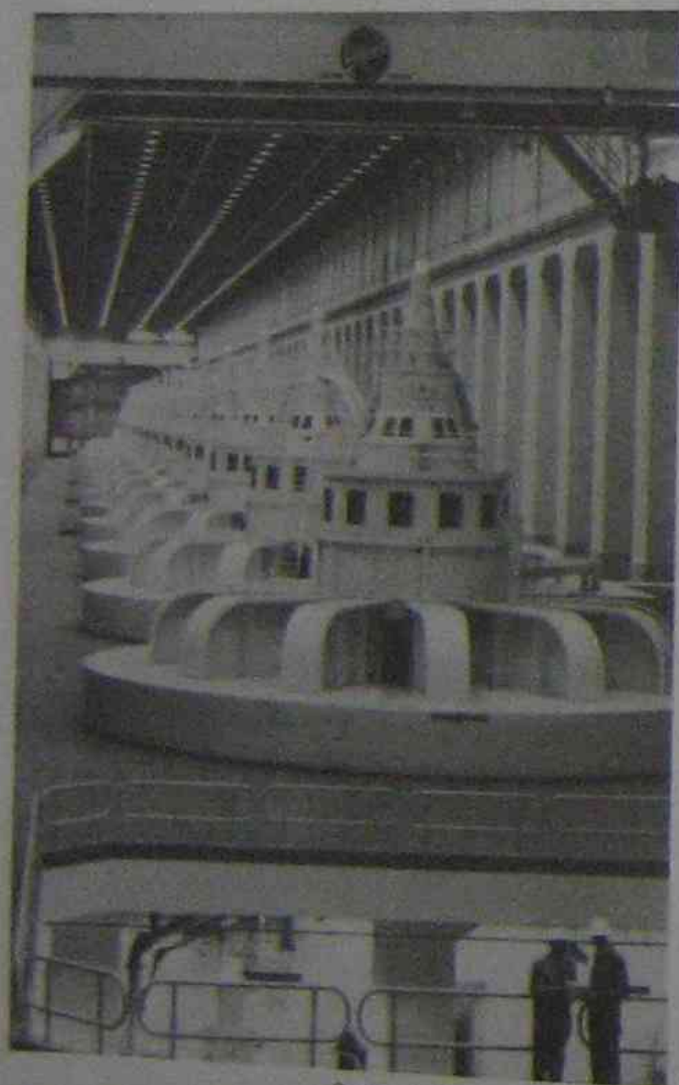
Fig. 2-21. Generators inside a hydroelectric power plant.
