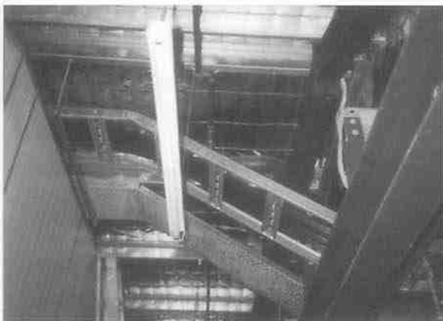
Fig. 7.14 Perforated-tray cable support (background) and ladder support (foreground)
