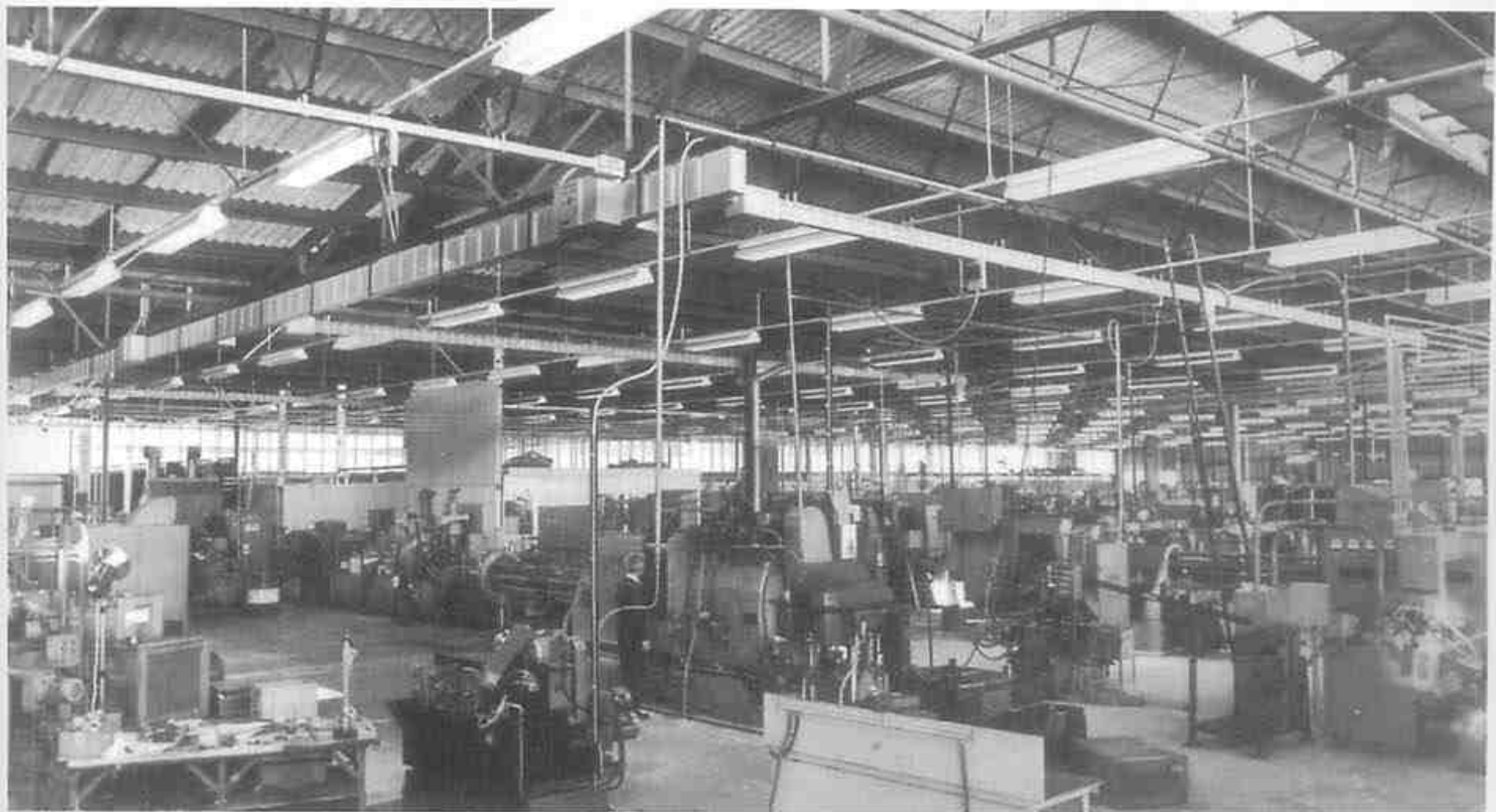
Fig. 7.18 Aluminium feeder (1200 A) with plug-in take-offs VASS ELECTRICAL INDUSTRIES
