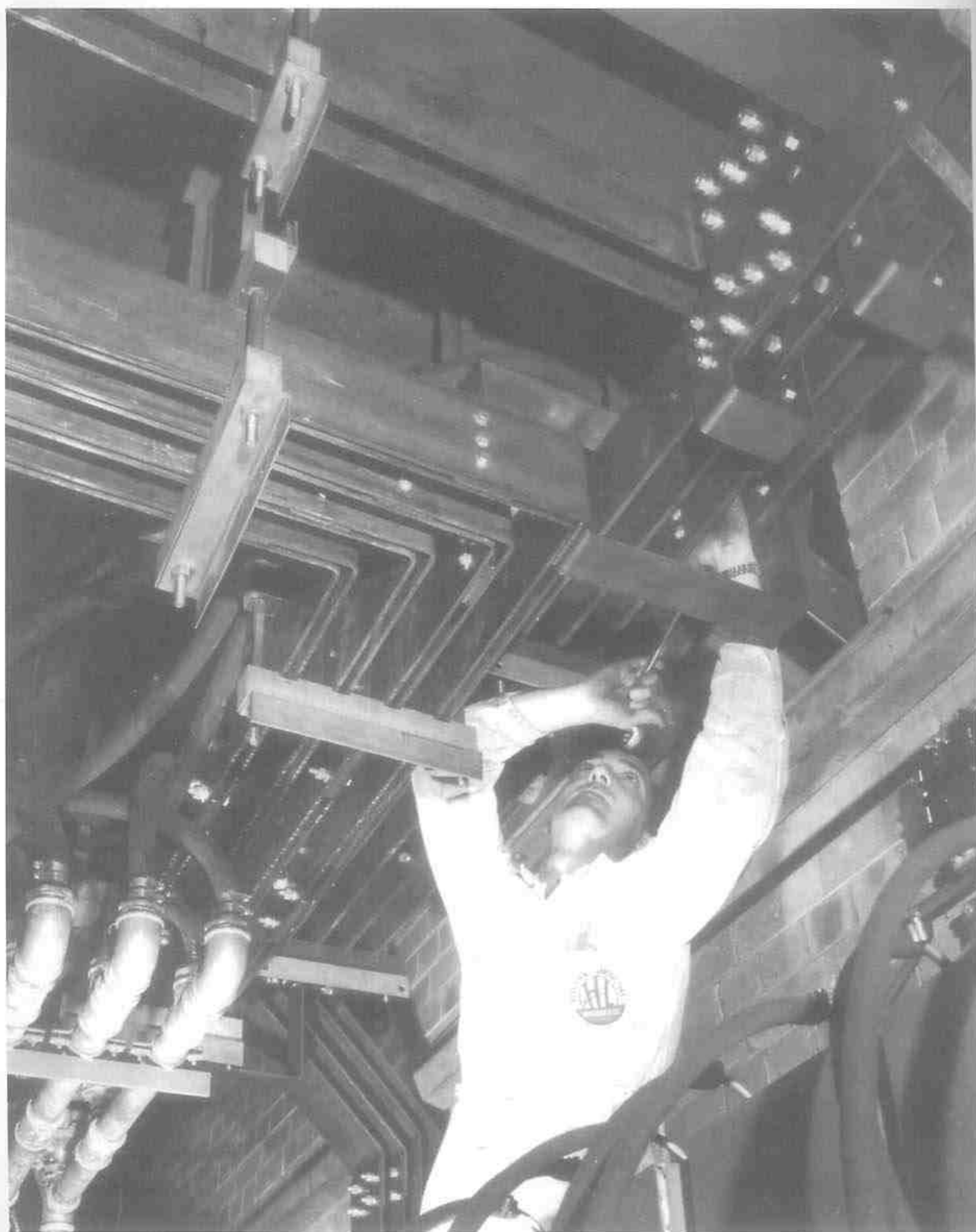
Fig. 7.2 5000 A busbars on a triple induction furnace HODGSON & LEE
