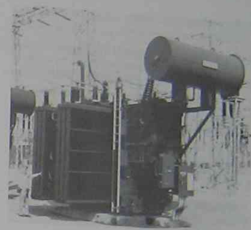
Figure 10.19 Three-phase, type OA/FA/FOA transformer rated 36/48/60 MVA, 225 kV/26.4 kV, 60 Hz, impedance 7.4%. The circular tank enables the oil to expand as the temperature rises and reduces the surface of the oil in contact with air. Other details:
